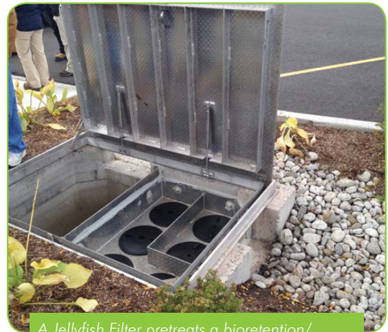
A Jellyfish Filter pretreats a bioretention/bioswale system at a commercial site in Ontario, Canada.
