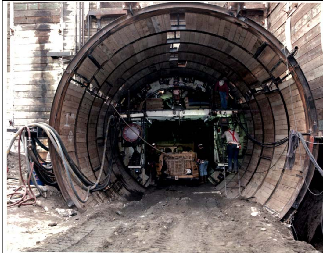
Photo No. 1. False tunnel sets at the South Tunnel Portal of YR Tunnel (south of LAUS) with tunnel shield and mucking machine in the background. Photo taken: 01/30/90. Source: SCRTRD, 1990a.
