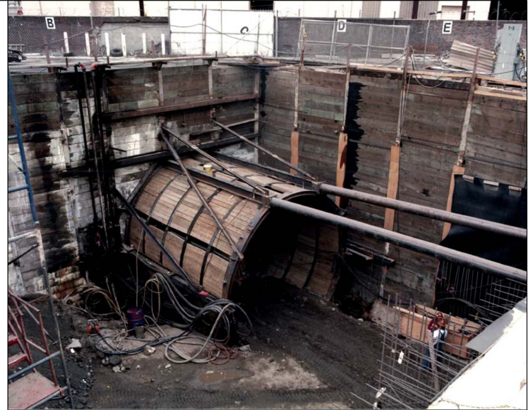
Photo No. 2. False tunnel sets and the jacking frame and struts for pushing the shield off of at the South Tunnel Portal (south of LAUS). Photo taken: 01/30/90. Source: SCRTRD, 1990a.
