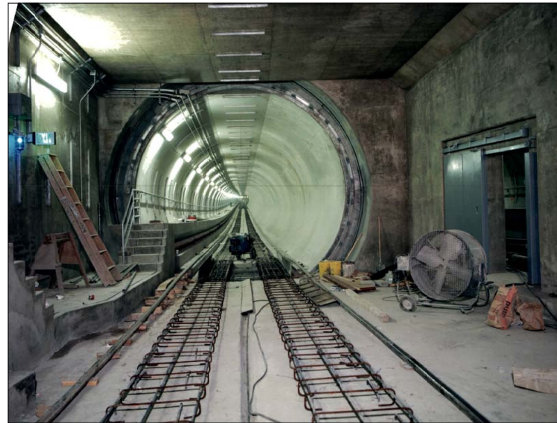
Photo No. 6. Interface between the box structure (LAUS area) on the YL side at Sta. 89+7 and the YL Tunnel (south of LAUS). Photo taken: 03/04/90. Source: SCRTD, 1990a.
