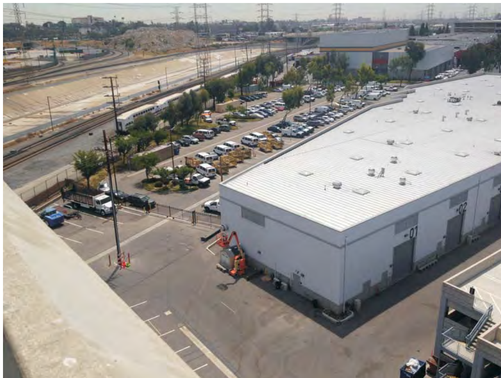
Looking south-east from top of parking structure
