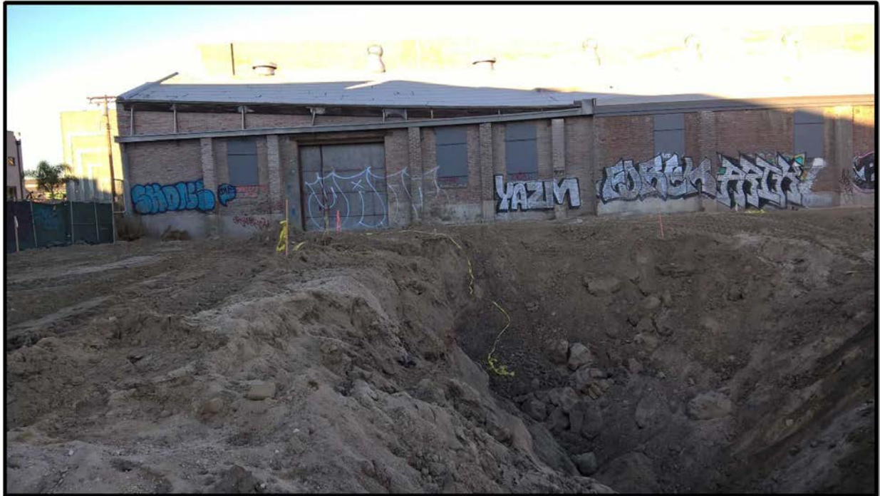
Photograph 25 – Overview looking west on December 15, 2015 of Excavation Area EA-5.
