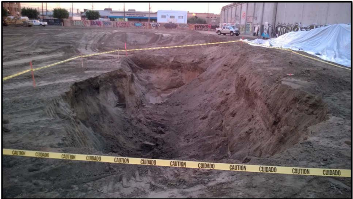
Photograph 23 – View looking east on December 9, 2015 at Excavation Area EA-5.
