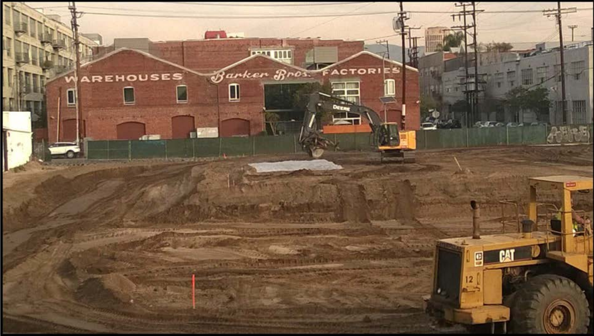
Photograph 21 – View on December 9, 2015 of removed oil piping being placed on plastic sheeting.
