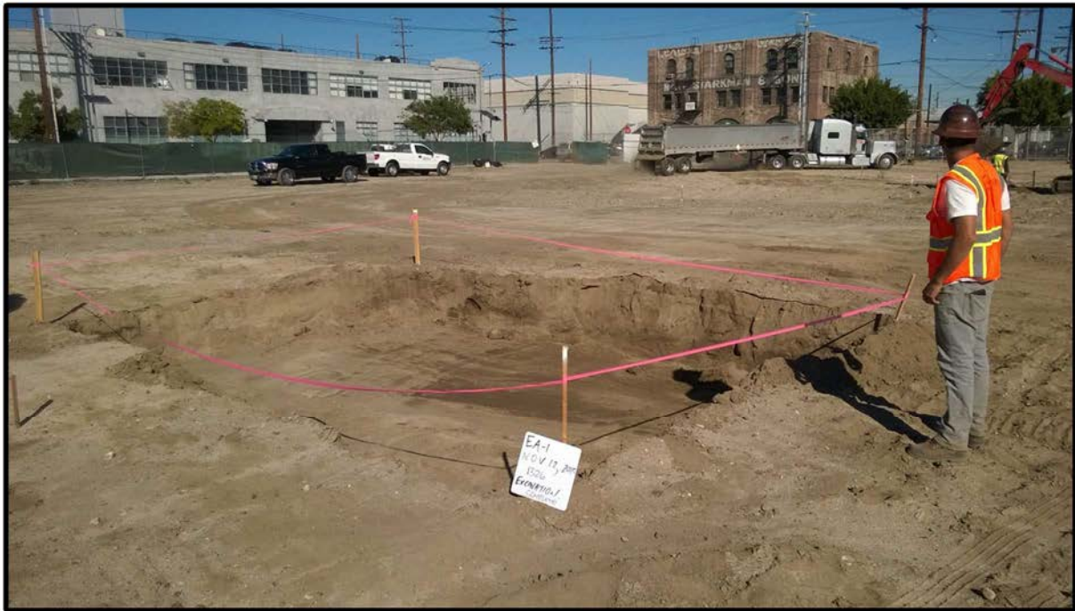
Photograph 15 – View looking northeast on November 12, 2015 at Excavation Area EA-1 excavation.
