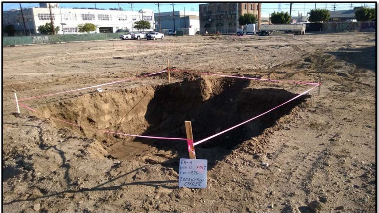
Photograph 10 – View on November 12, 2015 looking northeast at Excavation Area EA-4 excavation.
