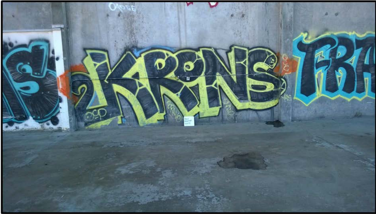
Photograph 3 – View looking south on November 12, 2015 at the southern dust monitor (on concrete wall).
