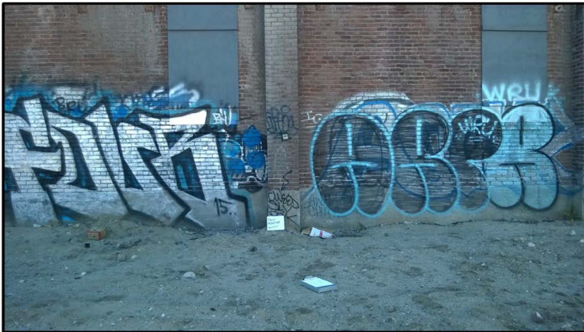
Photograph 2 – View looking west on November 12, 2015 at the western dust monitor (on brick wall).
