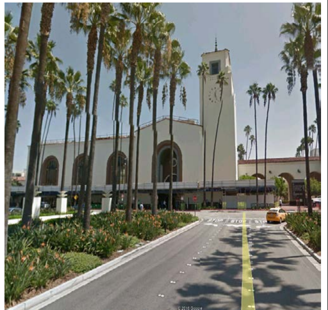
Photo 24: Map Code #76 – 800 N. Alameda Street. Potential for petroleum hydrocarbon impacted soil and soil vapor, and naturally occurring petroleum seeps and methane. The view is toward the north.
