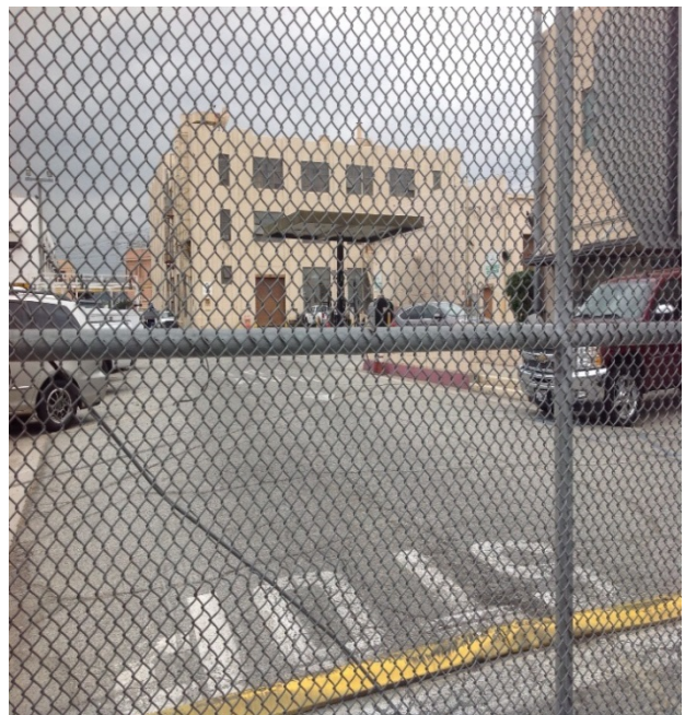
Photo 4: HDR Map Code #17 - 1630 N. Main Street. Los Angeles Water Department yard with gasoline pumps. Site has an open LUST case. The view is toward the northeast.
