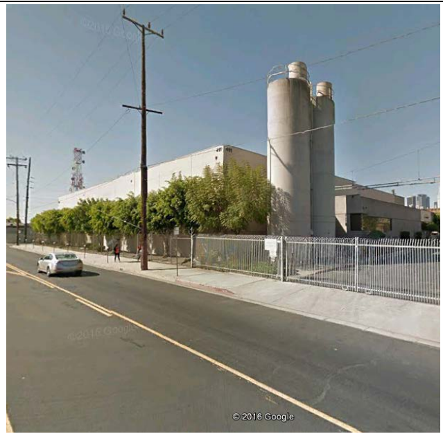
Photo 18: No HDR Map Code - 411 Center Street. Site of Upper Crust Bakery with three ASTs. View is toward the southwest. Previous site of Manley Oil.
