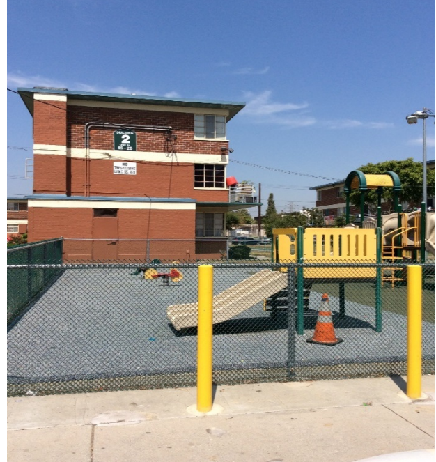
Photo 6: HDR Map Code #31 - 1300 Cardinal Street. William Mead residential area and playground. Active cleanup site with deed restrictions. The view is toward the northwest.
