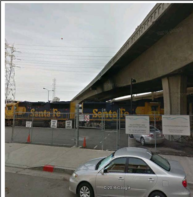
Photo 25: HDR Map Code #84 – 720 Keller Street. Current Site of the Keller Street Yard. Site has land use restrictions and is a voluntary cleanup site. The view is toward the south.
