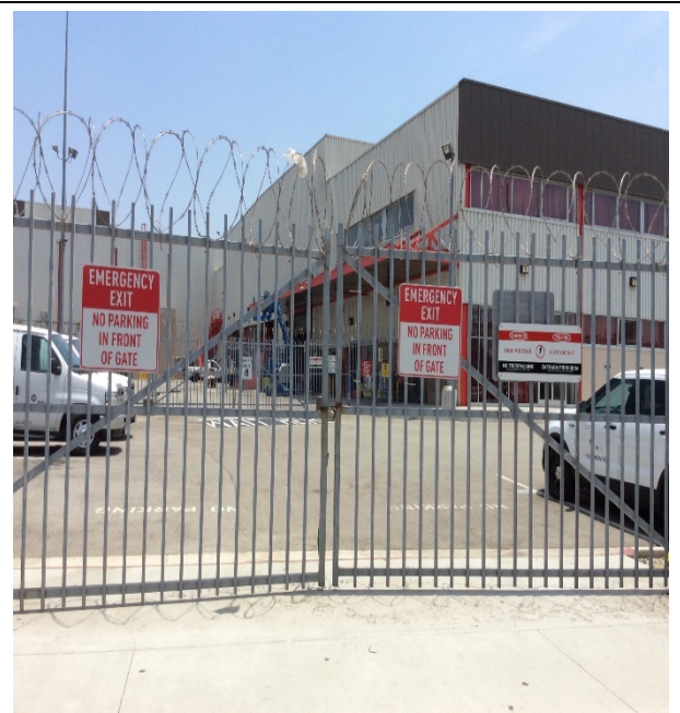
Photo 26: HDR Map Code #95 – 284 S. Santa Fe Avenue. Site of the MTA Red Line Maintenance facility. The view is toward the east.
