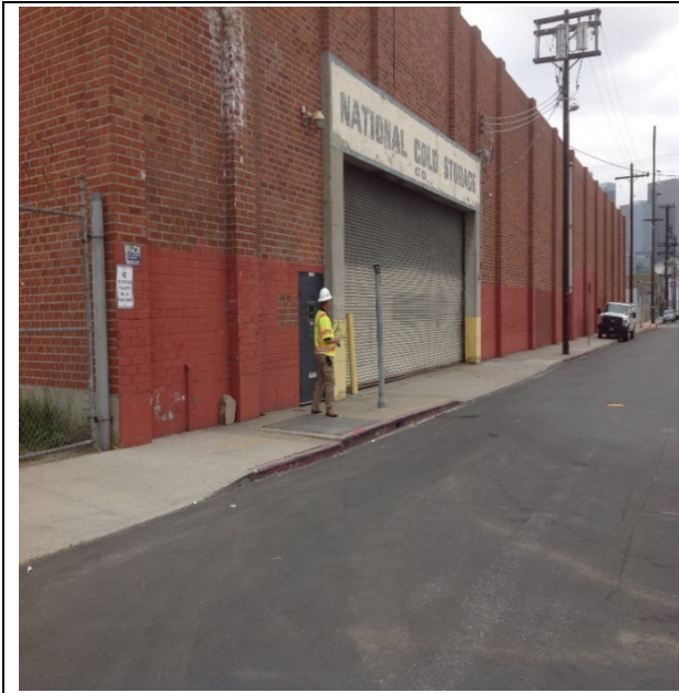
Photo 17: HDR Map Code #64 - 820 E. Jackson Street. Site of the former National Cold Storage Company. Site has land use restrictions due to the former Alisson MGP. The view is toward the west.
