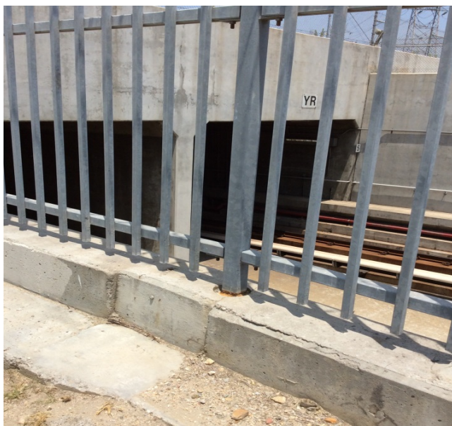
Photo 15: No HDR Map Code. Railroad tunnel into LAUS at the end of E. Commercial Street.
