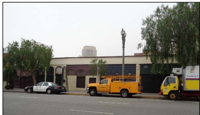
Figure 28: Jones Building, camera facing southeast. ICF, 2018.
