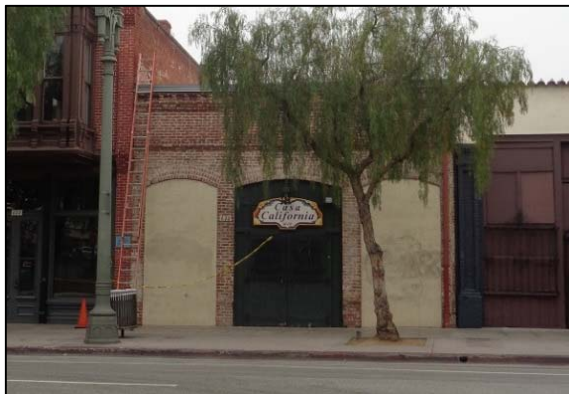
Figure 27: Machine Shop, camera facing southeast. ICF, 2018.
