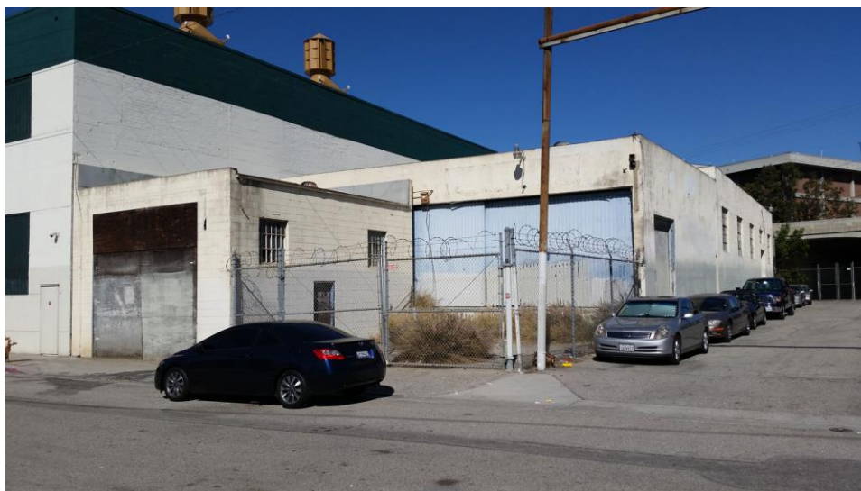
Looking northwest, Photo #105117.jpg. Photo: ICF International, 11/7/2014
