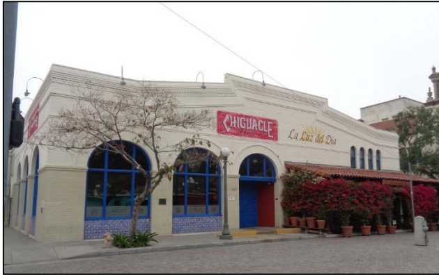
Figure 29: Jones-Simpson Building, camera facing north. ICF, 2018.
