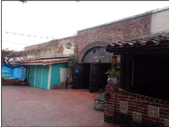
Figure 21: The Winery, camera facing north. ICF, 2018.
