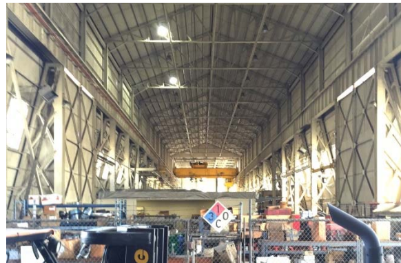
Hoist House, 1935. (19-176370). Camera Facing W. Photo: ICF International, July, 2016. IMG_9127.jpg
