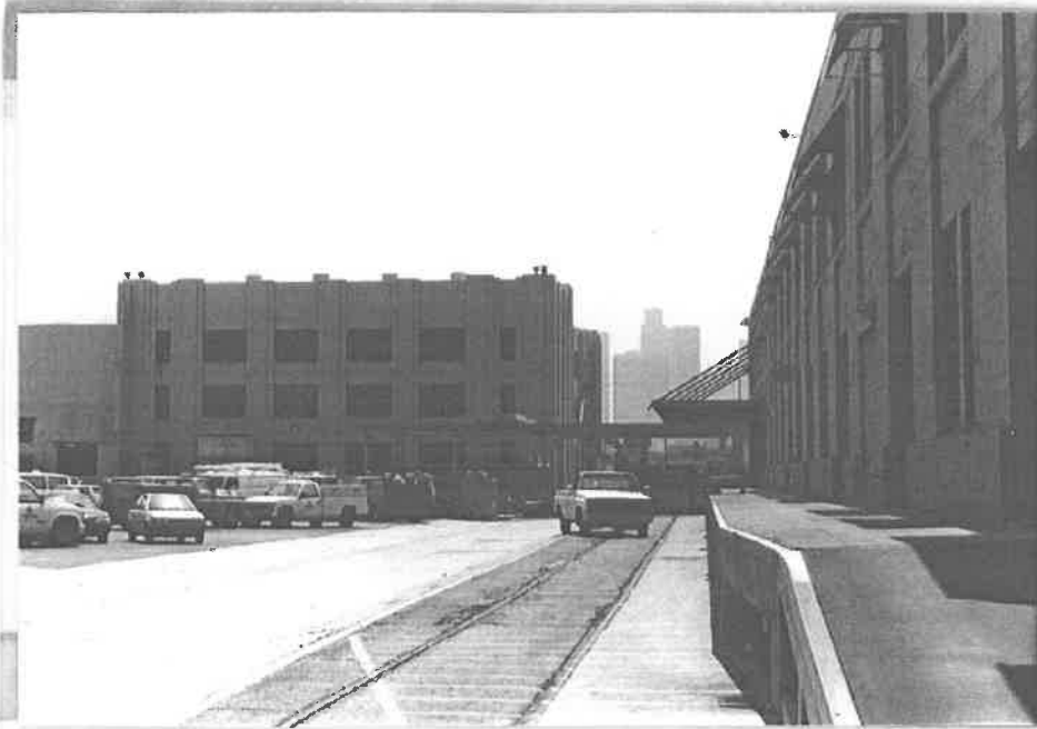
Building No. 9 (left), Building No. 3 (right)-W - Context
