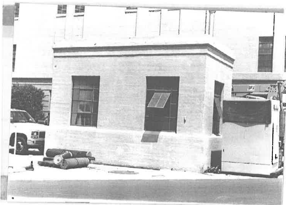
Hoist House-NE - Contributing
