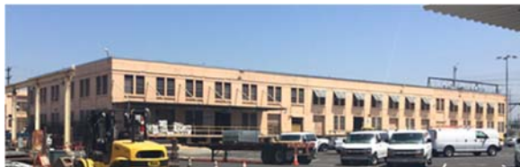
Building 3: General Warehouse, 1924. (19-175282). Camera facing NW. Photo: ICF International, July, 2016. IMG_9284.jpg
