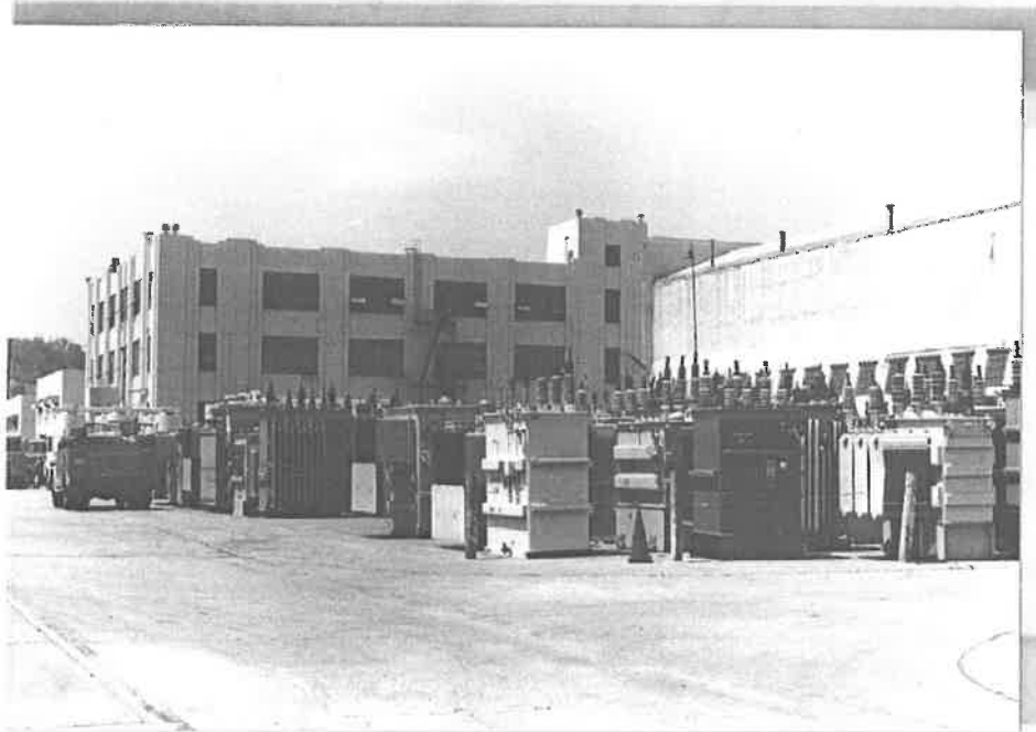
Building No. 9-N - Context.
