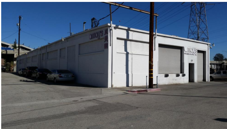
Looking northeast, Photo #105107.jpg. Photo: ICF International, 11/7/2014
