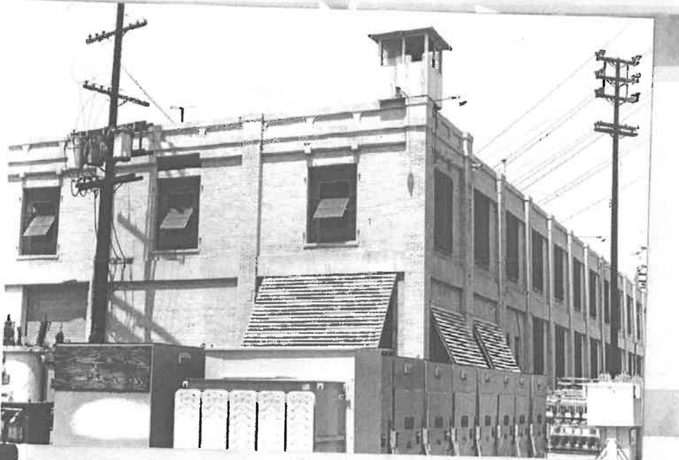
Building No. 11-E - Contributing
