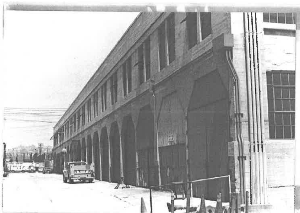
Building No. 3-SE - Contributing
