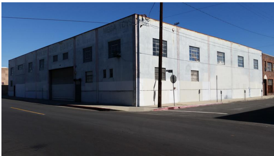
Looking northeast, Photo #110926.jpg. Photo: ICF International, 11/7/2014
