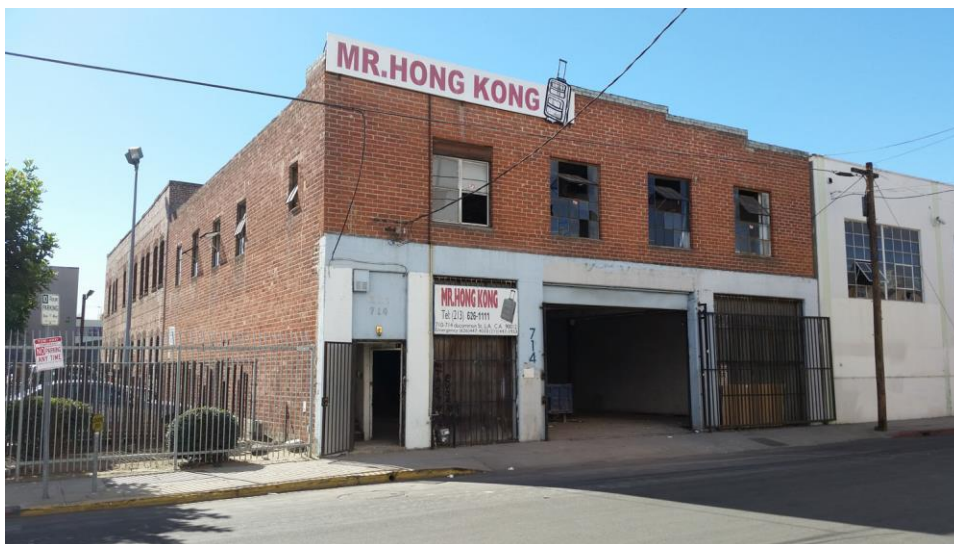
Looking southwest, Photo #110503.jpg. Photo: ICF International, 11/7/2014
