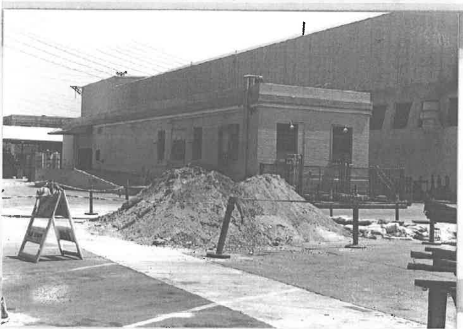
Building No. 10 (foreground), Building No. 9 (background)-SW - Contributing
