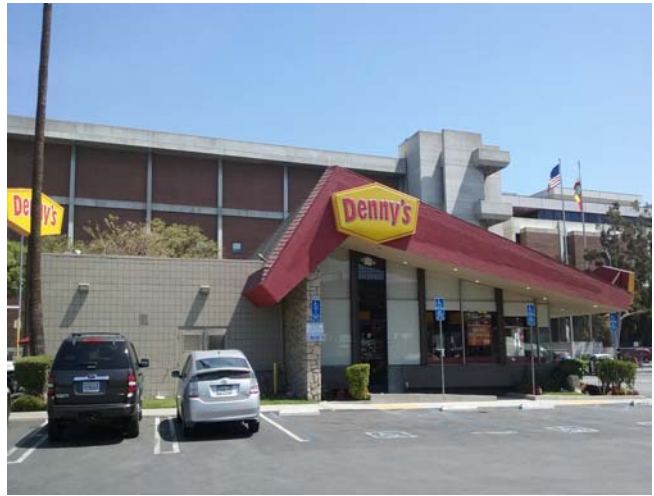
South Elevation, North View
