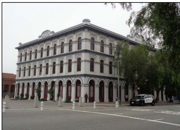
Figure 7: Pico House, camera facing south. ICF, 2018.
