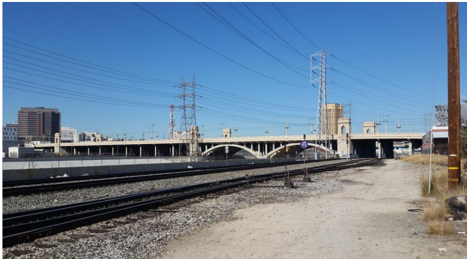
Looking northwest, Photo #113427.jpg, taken 11/7/2014
