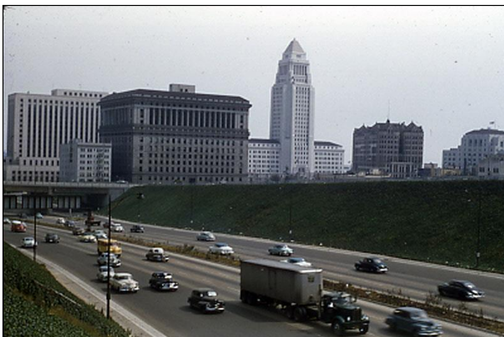
Photograph 8. US 101 Slot, Hill and Broadway, view to south-east, 1955 (LAPL No. 00110010)
