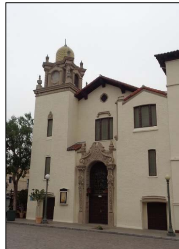
Figure 16: Plaza Methodist Church, camera facing northeast. ICF, 2018.
