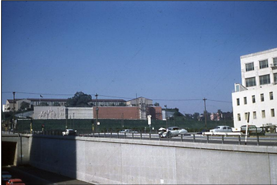
Photograph 9. US 101 Slot, Broadway and Spring, view to north-west, 1958 (LAPL No. 00110078)
