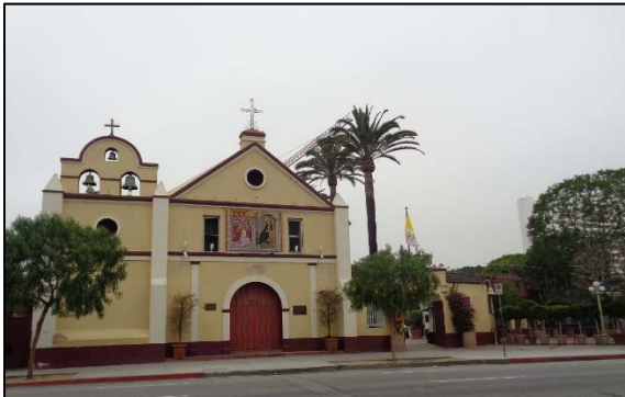
Figure 3: Old Plaza Church, camera facing west.
