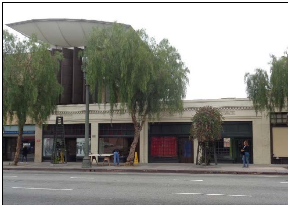
Figure 23: Hammel Building, camera facing southeast. ICF, 2018.
