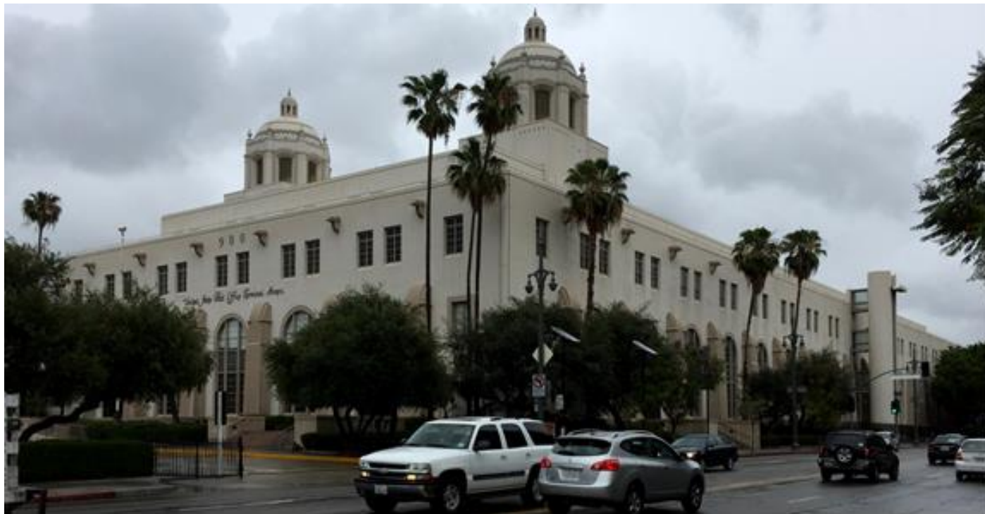
Los Angeles Terminal Annex Post Office. Camera facing NE. Photo: ICF International, June, 2015.
