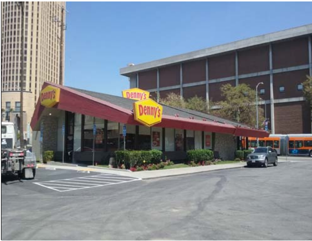
East Elevation, Northwest View
