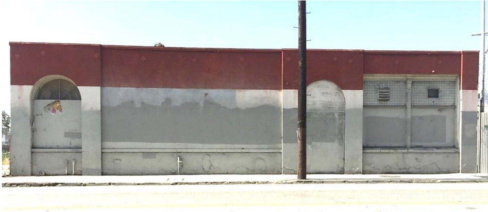
430 E. Commercial St., front elevation. Camera facing south. ICF International. July 14, 2016.
