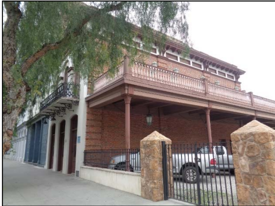
Figure 9: Masonic Hall, camera facing east. ICF, 2018.
