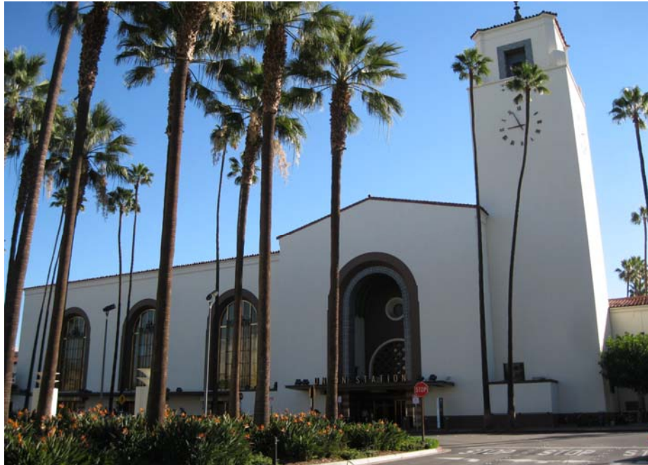
Looking east, Photo # IMG_3820.jpg. Photo: ICF International, 11/7/2014
