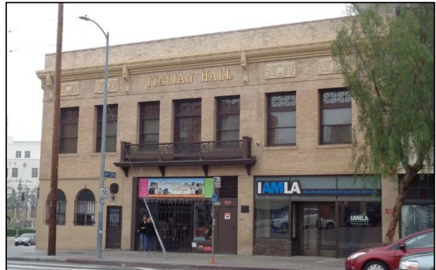
Figure 22: Italian Hall, camera facing east. ICF, 2018.
