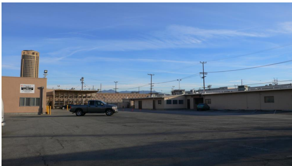
Looking north, Photo #P1030882.jpg. Photo: ICF International, 11/18/2014
