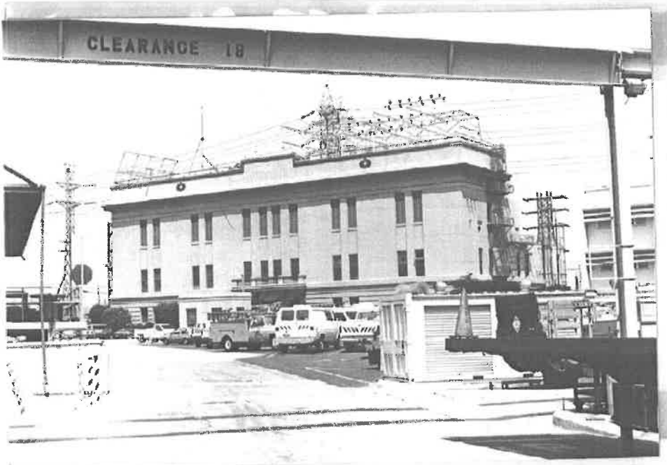
Building No. 5-SE - Contributing
