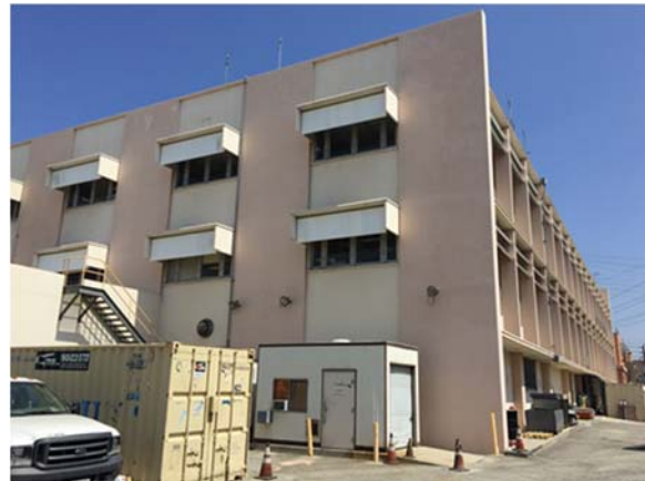
Building 7: Testing Laboratories Building, 1965, (19-176374). Camera Facing NW. Photo: ICF International, July, 2016. IMG_9162.jpg
