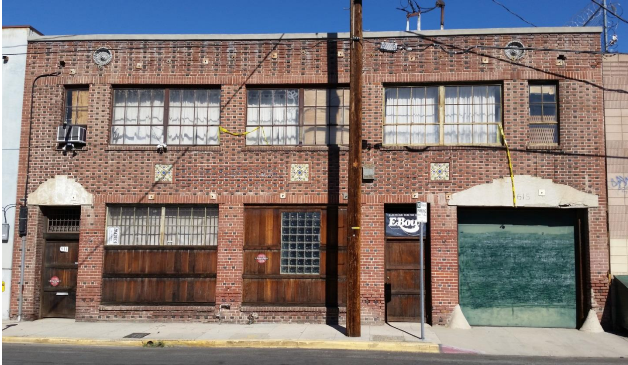
Thomas R. Barabee Store and Warehouse. Front elevation. View: N. Photo: Daniel Paul, ICF International. November, 2014.
