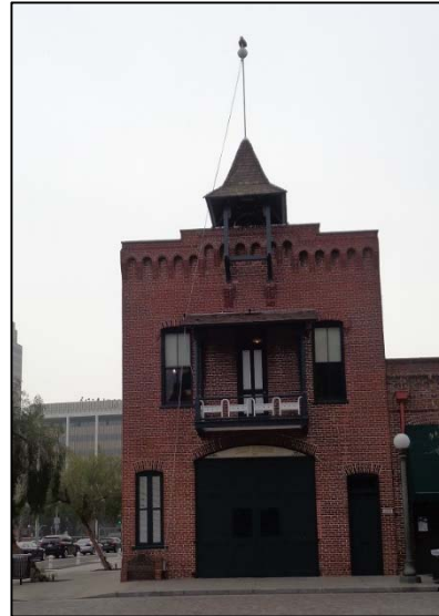
Figure 14: Plaza Firehouse, camera facing south. ICF, 2018.
