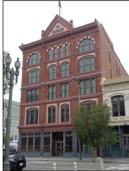
Figure 6: Vickrey-Brunswick Building, camera facing west. ICF, 2018.
