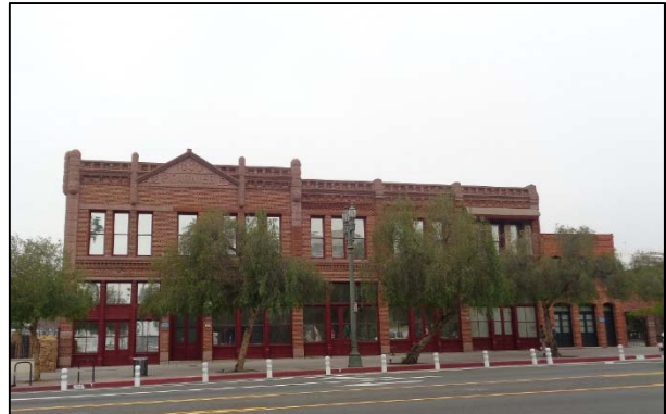
Figure 10: Garnier Building, camera facing northwest. ICF, 2018.
