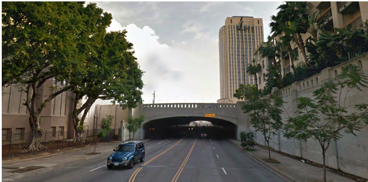
Figure 3.4-28. Key View #3b – Cesar Chavez Avenue (View Looking East toward Bridge) Existing Conditions
