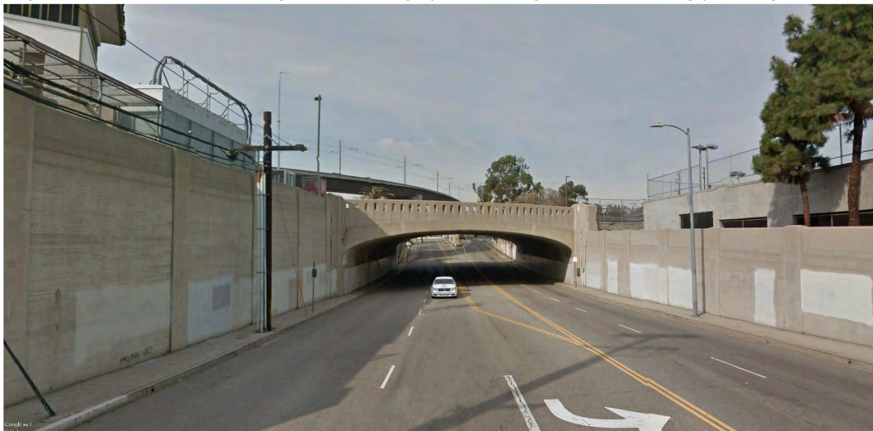
Figure 3.4-22. Key View #2a – Vignes Street Bridge (View Looking West toward Bridge) Existing Conditions
