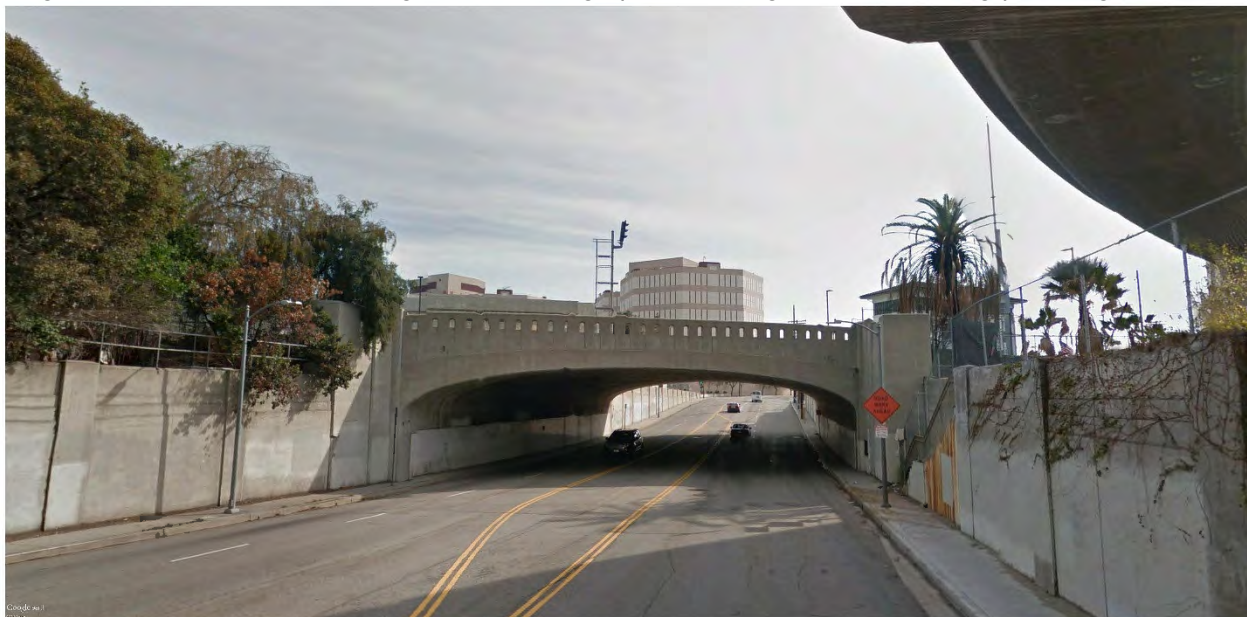
Figure 3.4-24. Key View #2b – Vignes Street Bridge (View Looking East toward Bridge) Existing Conditions
