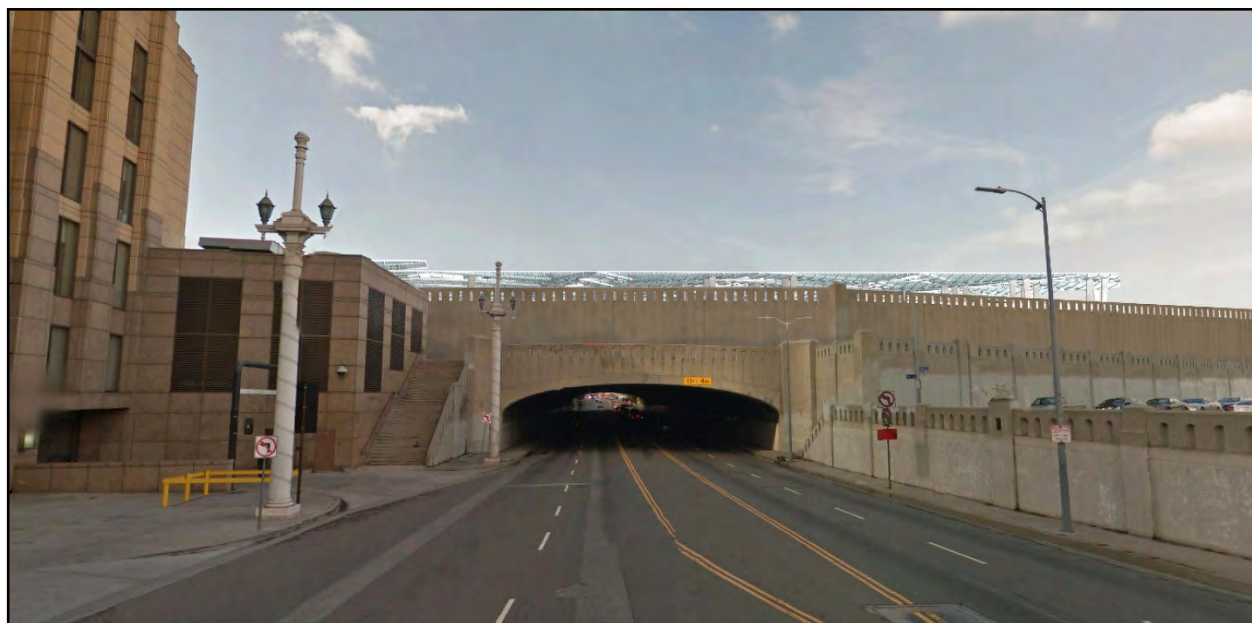
Figure 3.4-27. Key View #3a – Cesar Chavez Avenue (View Looking West toward Bridge) Post-Project Conditions
