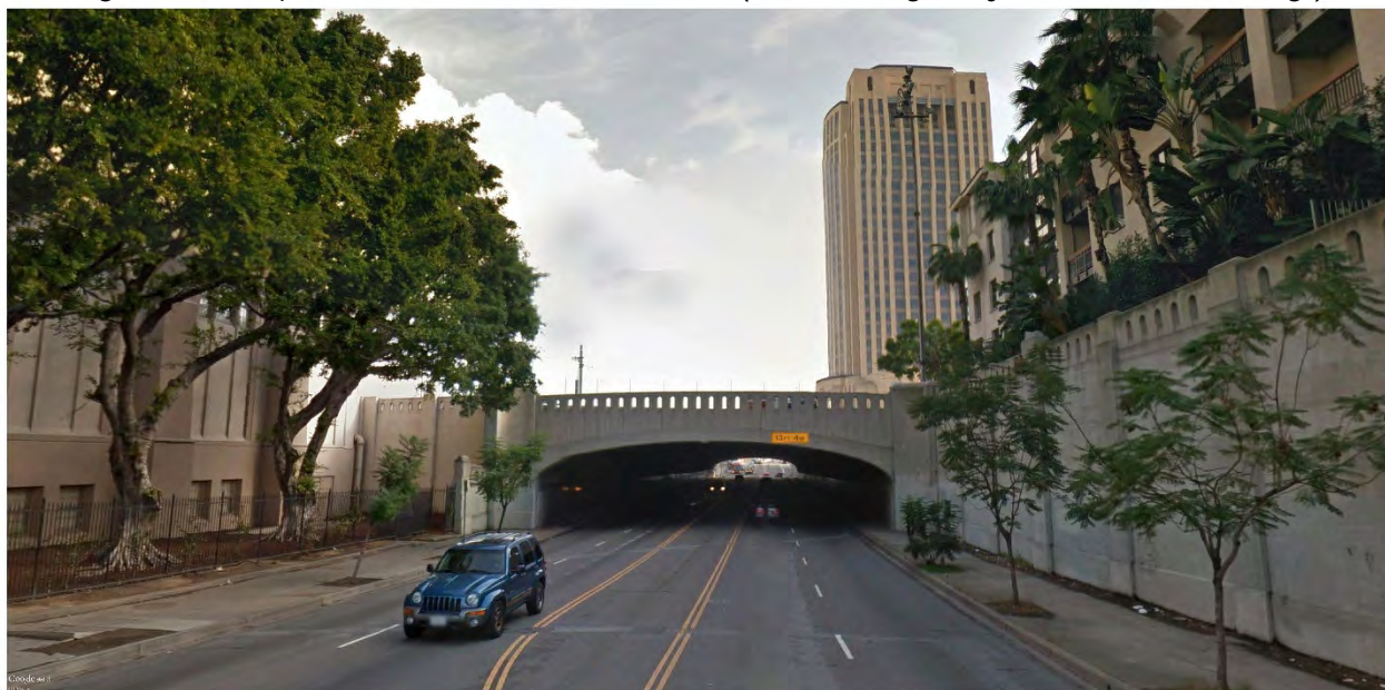
Figure 3.4-7. Key View #3b – Cesar Chavez Avenue (View Looking East from Road toward Bridge)
