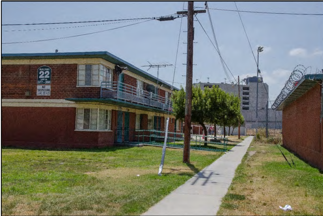
Figure 3.4-20. Key View #1b – Existing Conditions
