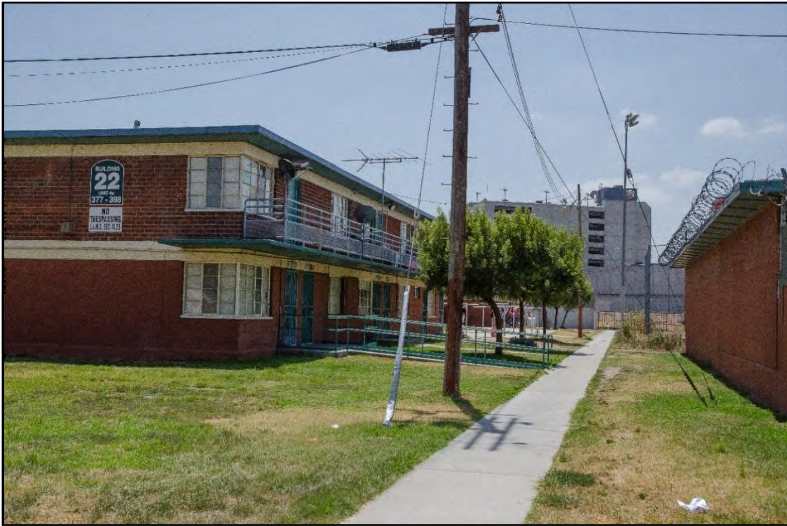
Figure 5-11. Key View #1b – Existing Condition (Retaining Wall)
