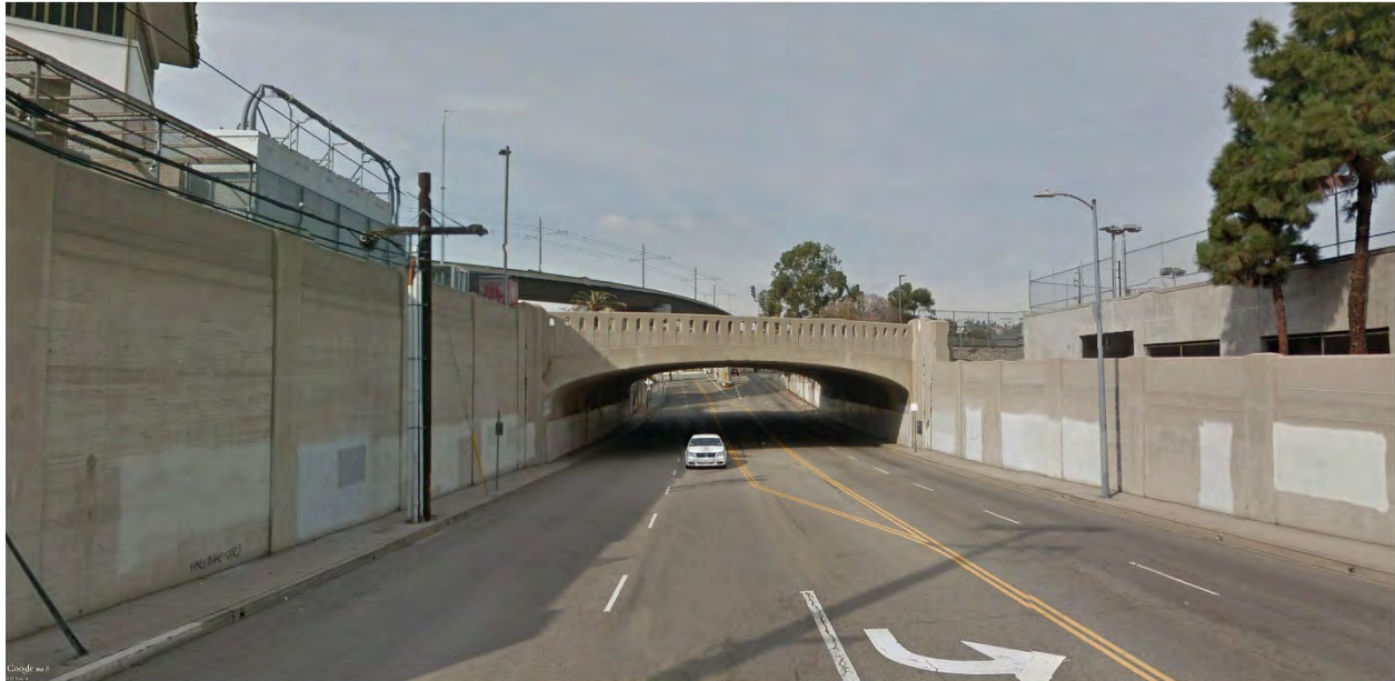
Figure 3.4-4. Key View #2a – Vignes Street (View Looking North from Road toward Bridge)
