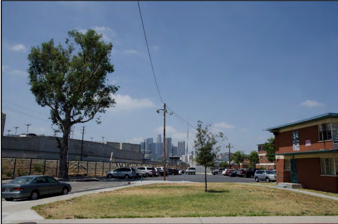
Figure 5-9. Key View #1a – Existing Condition (Retaining Wall)
