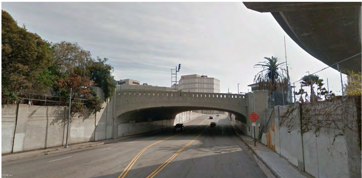
Figure 3.4-5. Key View #2b – Vignes Street (View Looking South from Road toward Bridge)
