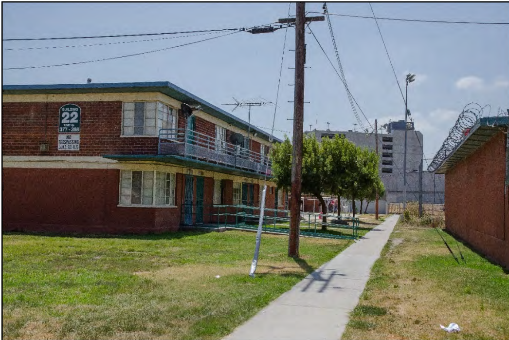
Figure 3.4-18. Key View #1b – Existing Conditions
