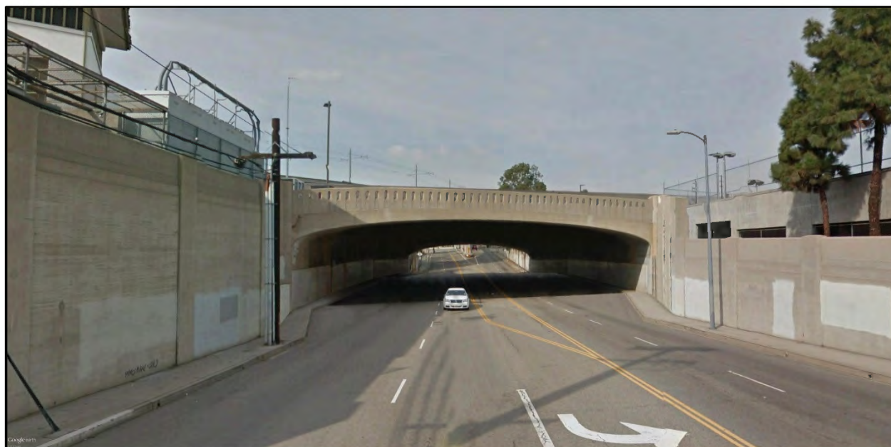
Figure 3.4-23. Key View #2a – Vignes Street Bridge (View Looking West toward Bridge) Post-Project Conditions
