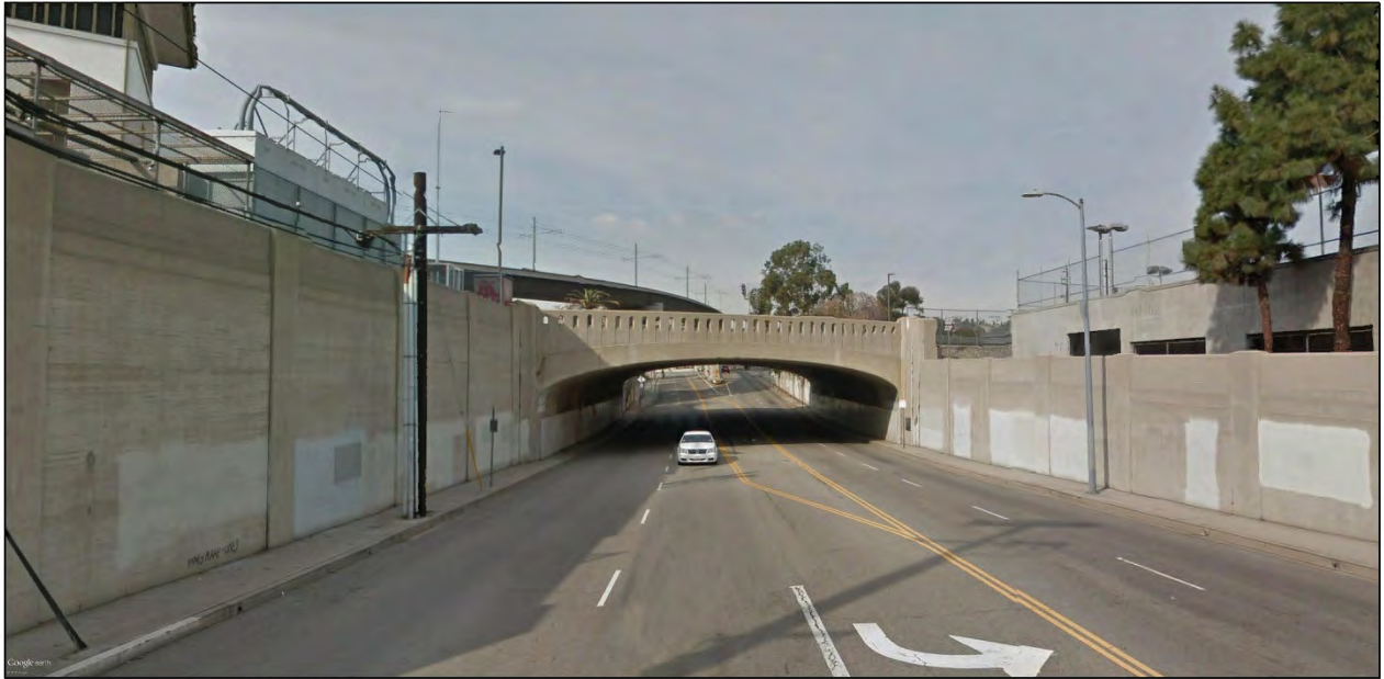
Figure 4-4. Key View #2a – Vignes Street (view looking north from road toward bridge)
