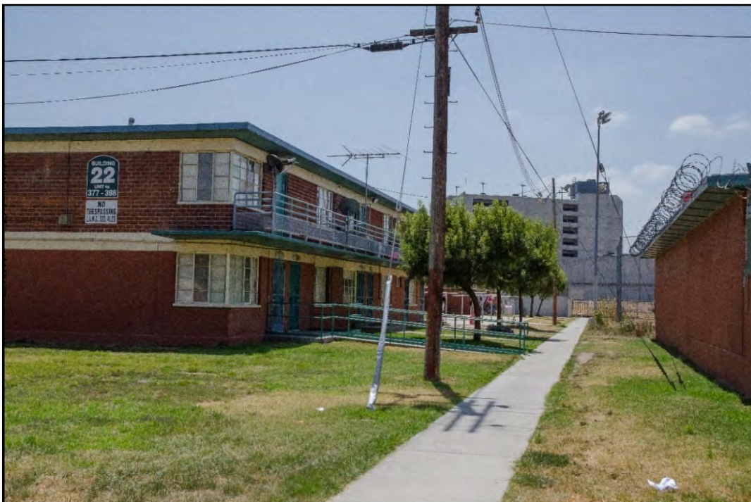
Figure 4-3. Key View #1b – William Mead Homes (view looking south from Elmira Street toward railroad right-of-way)
