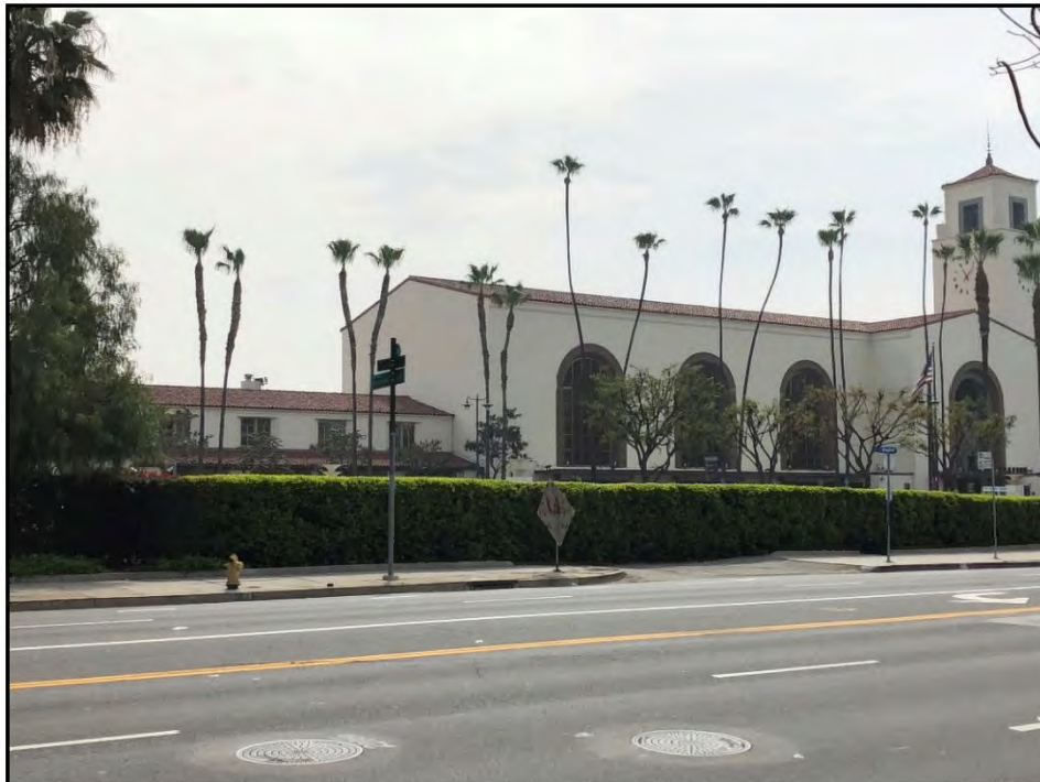
Figure 8-16. Key View #4a – Los Angeles Union Station Entrance (view looking southeast from Alameda Street toward Los Angeles Union Station) Existing Conditions
