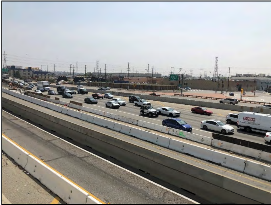
Figure 8-20. Key View #5a – US-101/Commercial Street (view looking southeast from Los Angeles Union Station toward US-101/Commercial Street) Existing Conditions
