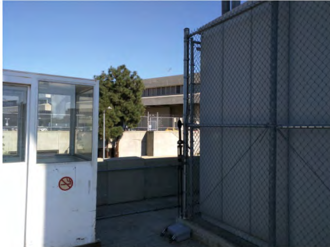
Figure B-11. Monitoring Location 2 Noise Meter, #3
