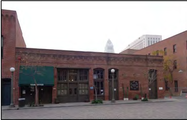
Figure 13: Hellman-Quon Building, camera facing south. ICF, 2018.
