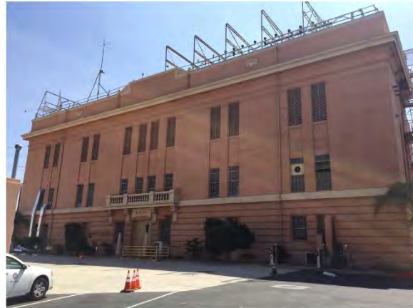
Building 5: Receiving Station A, 1925. (19-175283). Camera facing NE. Photo ICF International, July, 2016. IMG_9182.jpg
