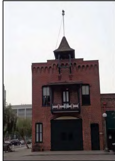
Figure 14: Plaza Firehouse, camera facing south. ICF, 2018.
