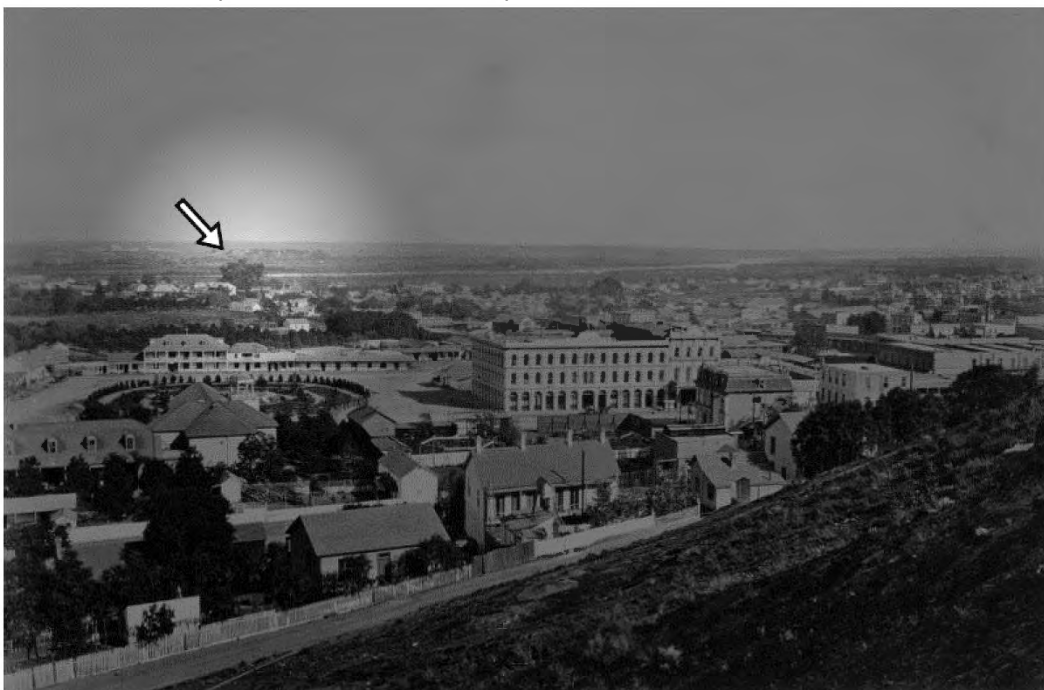
Figure 4-2. A photograph from circa 1876 shows Los Angeles Plaza, with El Aliso standing in the background (indicated by white arrow), view toward east-southeast
