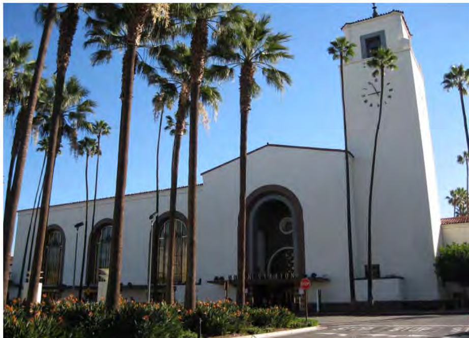
Looking east, Photo # IMG_3820.jpg. Photo: ICF International, 11/7/2014
