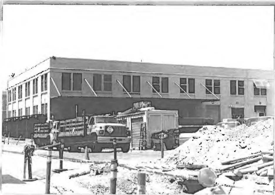
Building No. 3-N - Contributing
