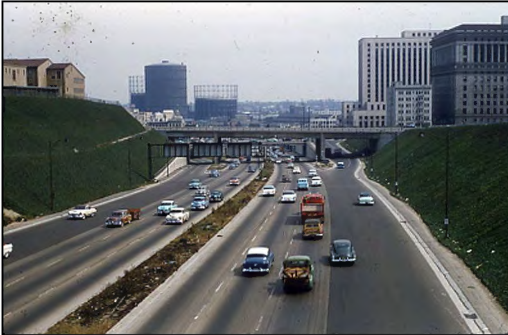
Photograph 7. US 101 Slot, Grand and Hill, view to east, 1955 (LAPL No. 00110008). [Compare to Photograph 1]
