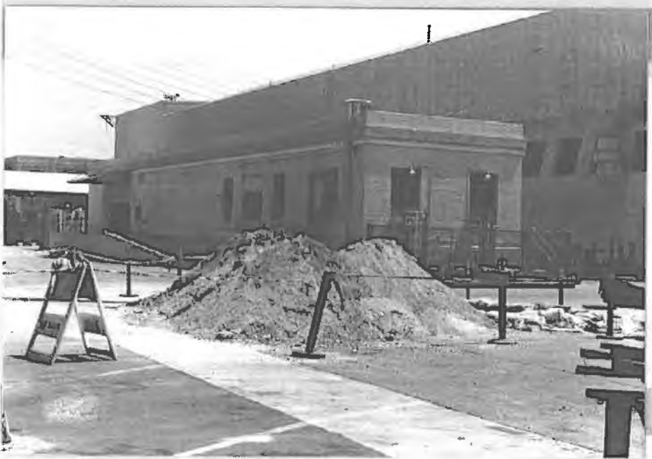
Building No. 10 (foreground), Building No. 9 (background)-SW - Contributing
