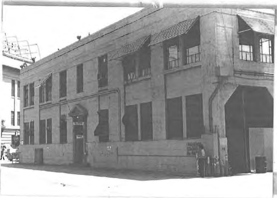
Building No. 3-W - Contributing
