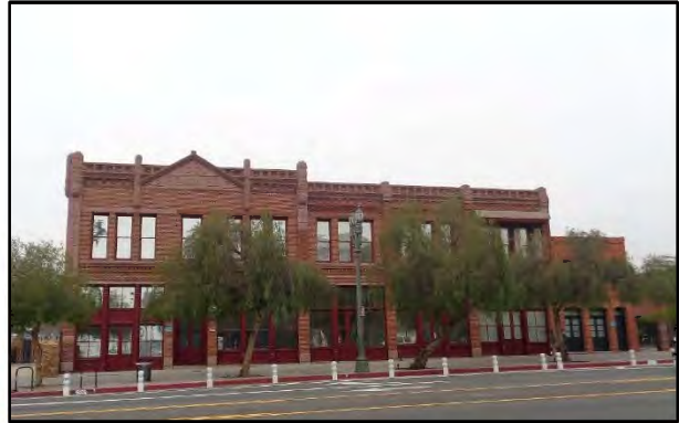
Figure 10: Garnier Building, camera facing northwest. ICF, 2018.
