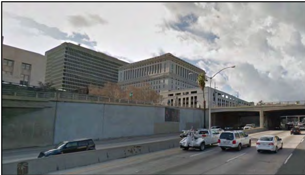
Photograph 4. US 101 Slot, US 101 Slot, Spring and Main, view to west, July 2016
