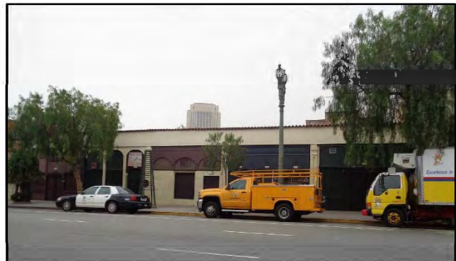
Figure 28: Jones Building, camera facing southeast. ICF, 2018.
