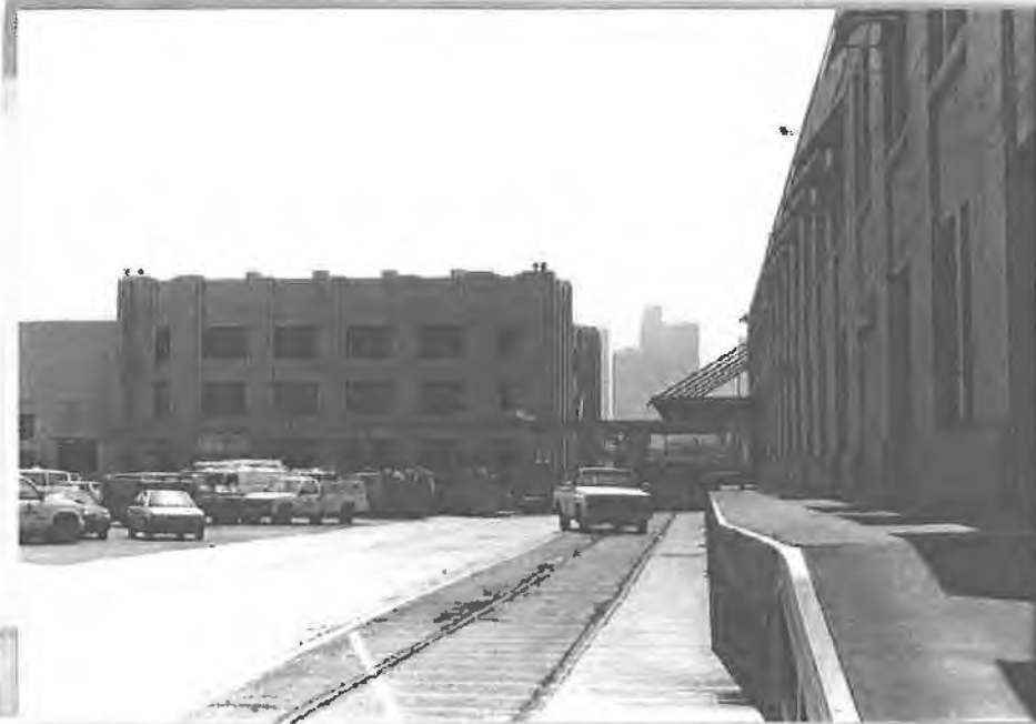
Building No. 9 (left), Building No. 3 (right)-W - Context.
