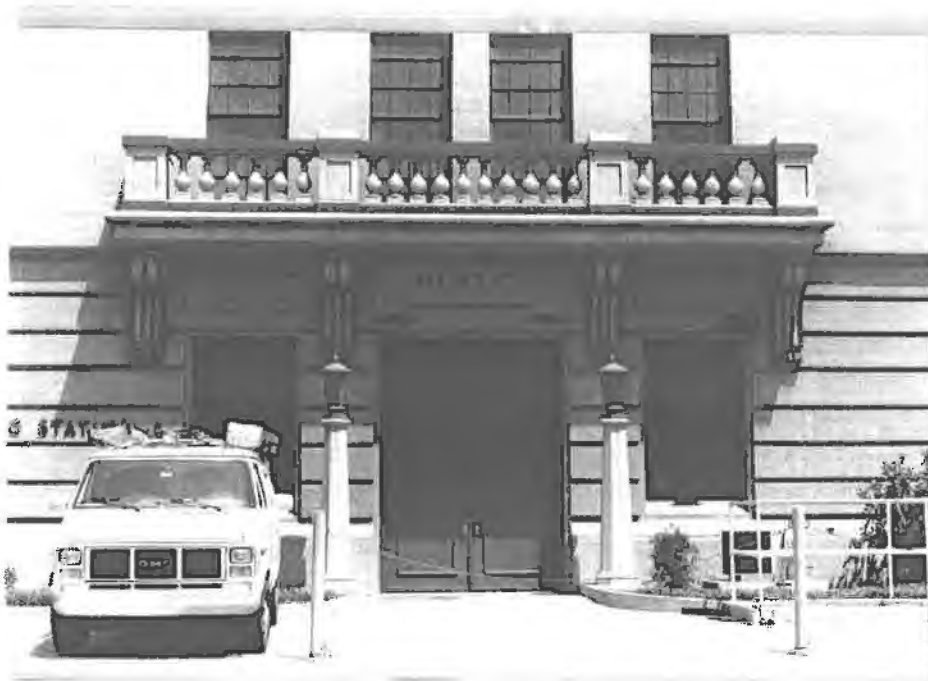
Building No. 5 (detail of entrance)-SE - Contributing
