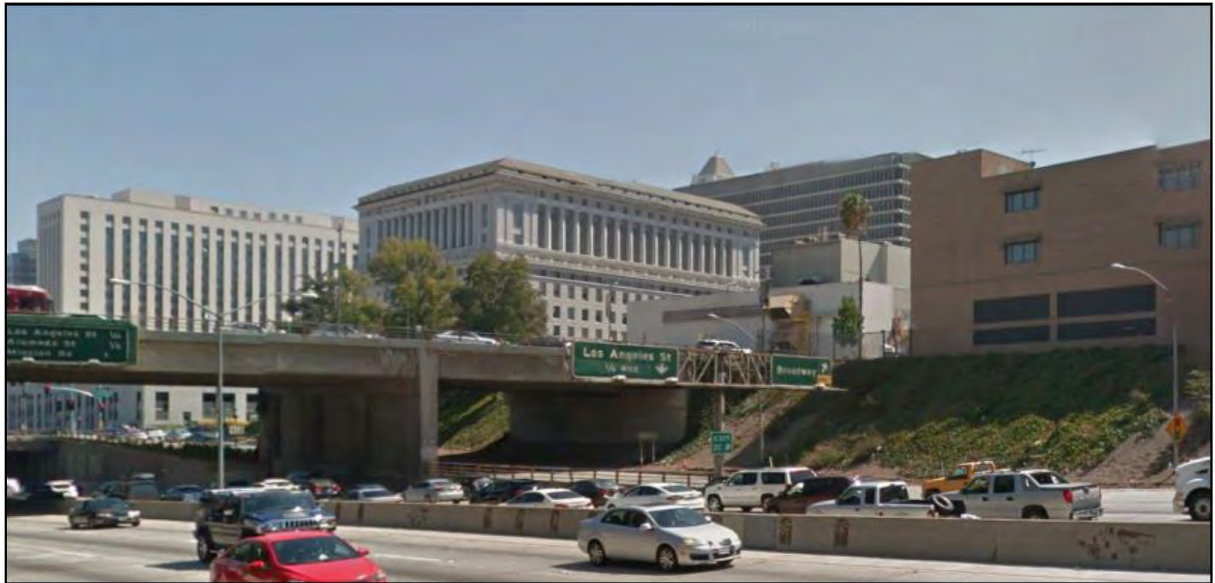
Photograph 2. US 101 Slot, Hill and Broadway, view to south-east, July 2016. [Compare to Photograph 8]
