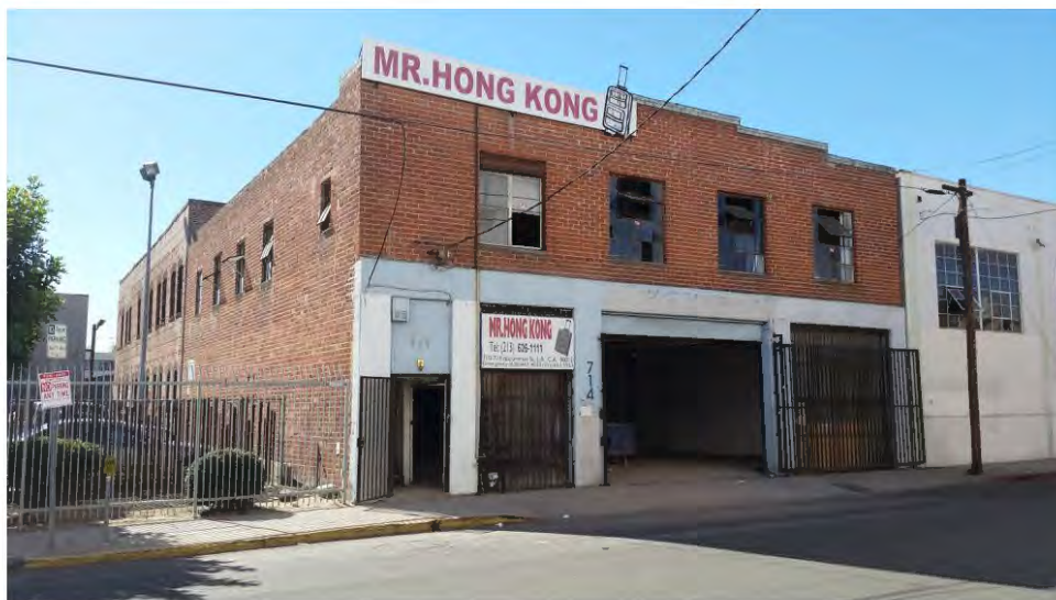
Looking southwest, Photo #110503.jpg. Photo: ICF International, 11/7/2014
