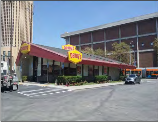
East Elevation, Northwest View
