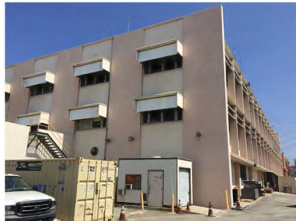
Building 7: Testing Laboratories Building, 1965, (19-176374). Camera Facing NW. Photo: ICF International, July, 2016. IMG_9162.jpg
