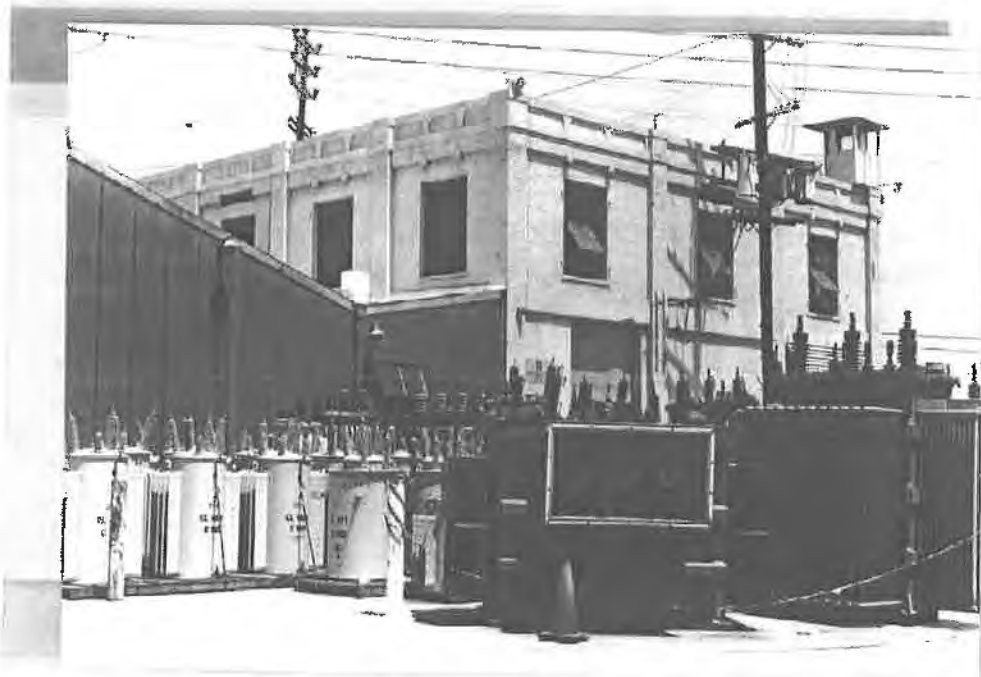
Building No. 11 (right), Building No. 11A (left)-SE - Contributing and Noncontributing, respectively
