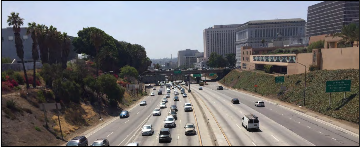
Photograph 1. US 101 Slot, Grand and Hill, view to east, July 2016. [Compare to Photograph 7]
