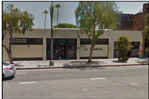
Figure 24: Pelanconi House/ Pelanconi Warehouse, North Main Street elevation, camera facing southeast. ICF, 2018.
