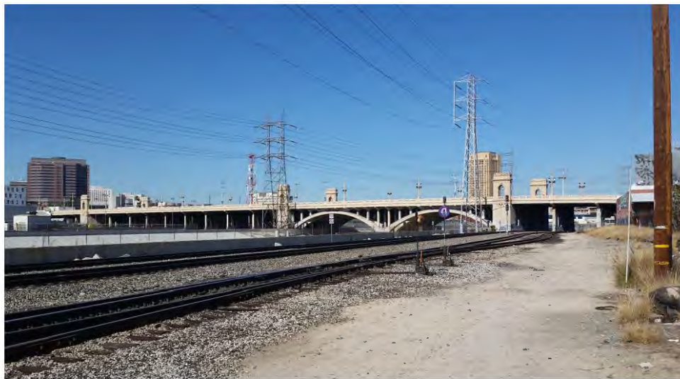
Looking northwest, Photo #113427.jpg, taken 11/7/2014
