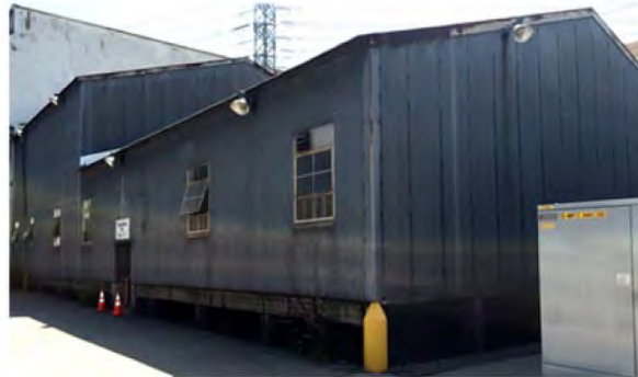
Building 11A: Transformer Test Building, 1961, (19-176372). Camera facing NE. Photo ICF International, July, 2016. IMG_9118.jpg
