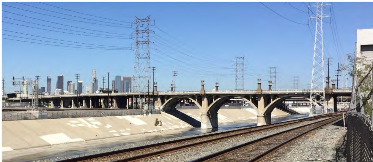
Looking northwest, Photo #7111, 04/12/2016
