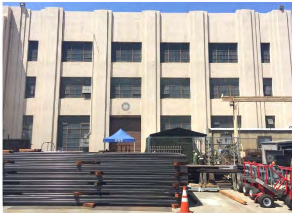
Building 9: Electrical Repair Shop, 1935/1937. (19-175284). Camera Facing S. Photo: ICF International, July, 2016. IMG_9276.jpg
