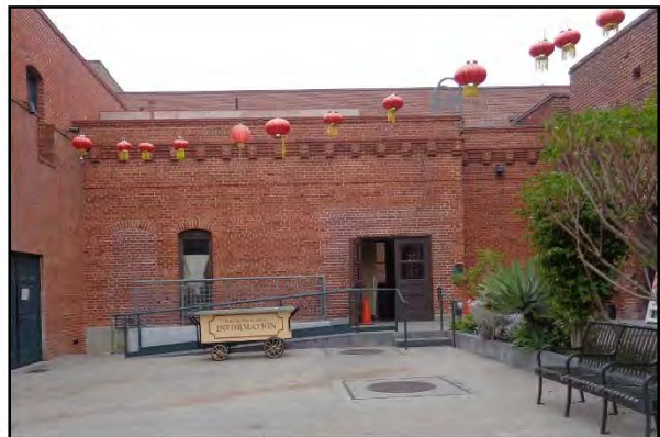
Figure 12: Turner Building, rear elevation, camera facing northeast. ICF, 2018.
