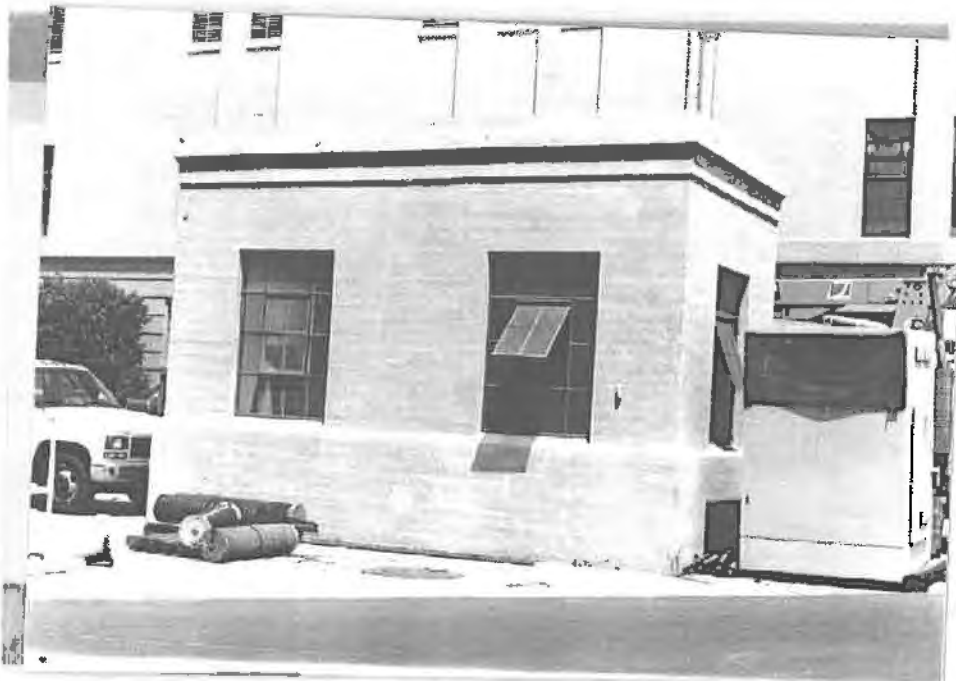
Hoist House-NE - Contributing
