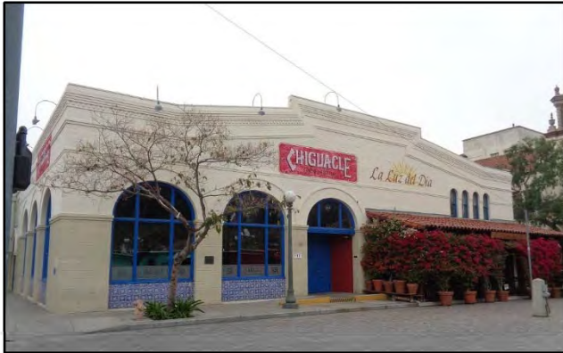
Figure 29: Jones-Simpson Building, camera facing north. ICF, 2018.
