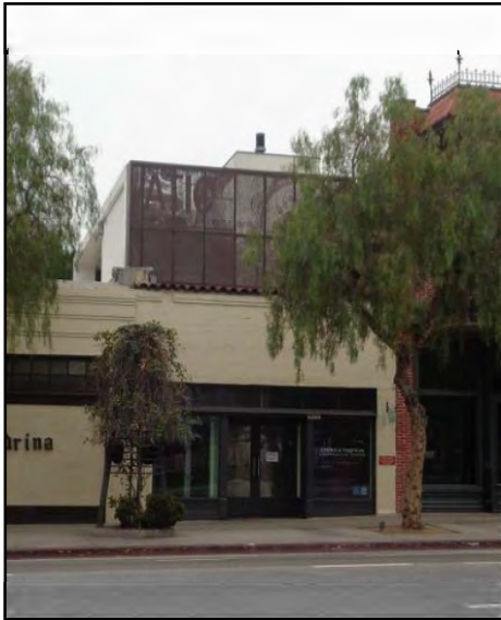
Figure 25: Gibbs Brothers Electric Company, camera facing southeast. ICF, 2018.
