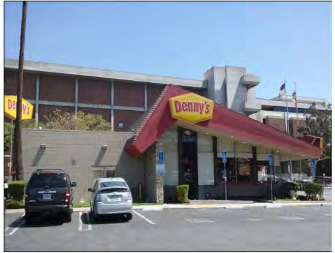
South Elevation, North View
