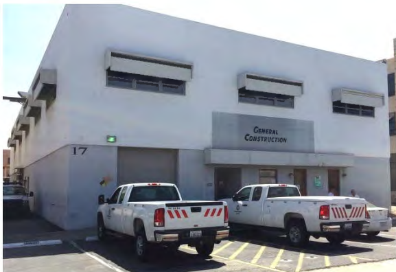
Building 17: Station Maintenance Building, 1963, (19-176373). Camera Facing SW. Photo: ICF International, July, 2016. IMG_9076.jpg
