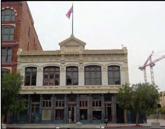
Figure 5: Plaza House, camera facing northwest. ICF, 2018.
