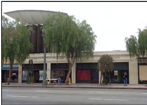
Figure 23: Hammel Building, camera facing southeast. ICF, 2018.
