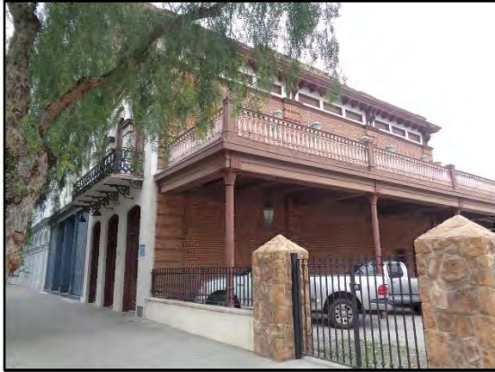
Figure 9: Masonic Hall, camera facing east. ICF, 2018.
