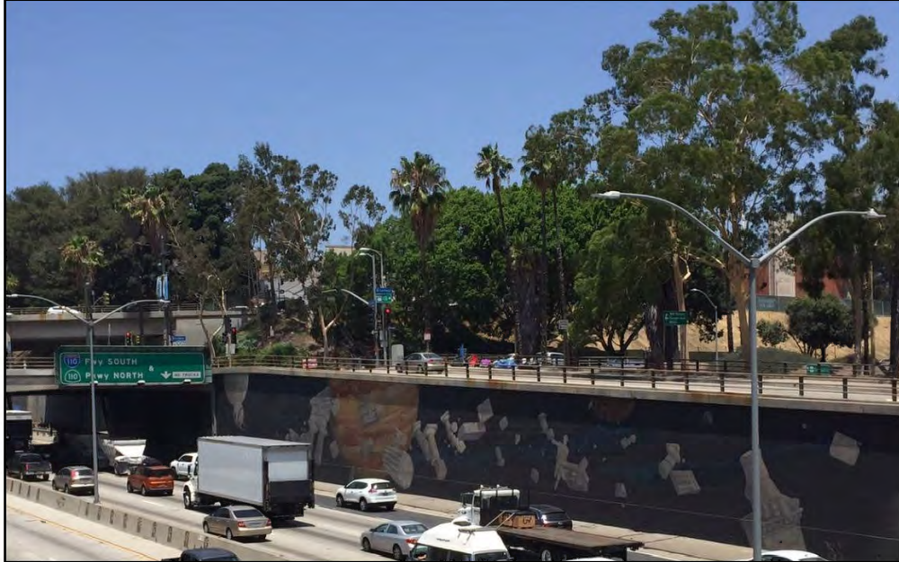
Photograph 3. US 101 Slot, Broadway and Spring, view to north-west, July 2016. [Compare to Photograph 9]
