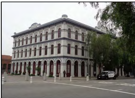
Figure 7: Pico House, camera facing south. ICF, 2018.
