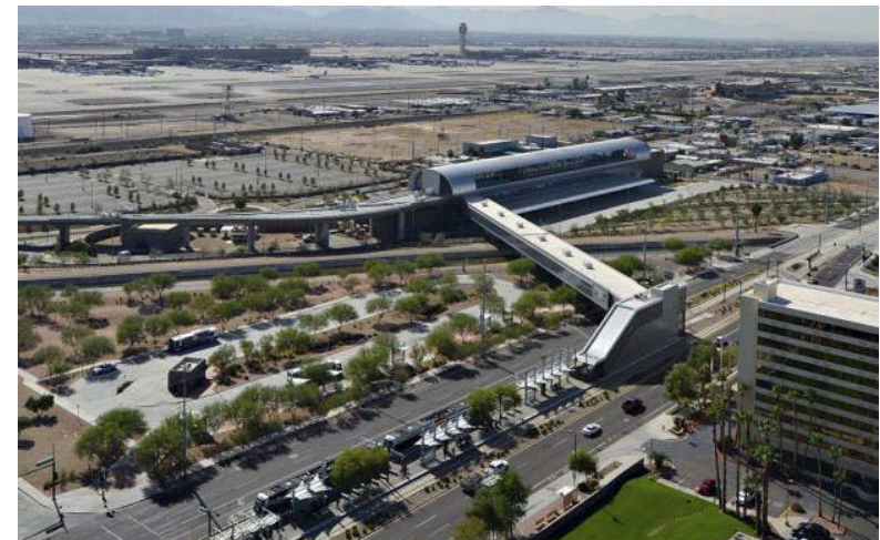
Phoenix SkyTrain Connection to Metro Light Rail & Bus Plaza
