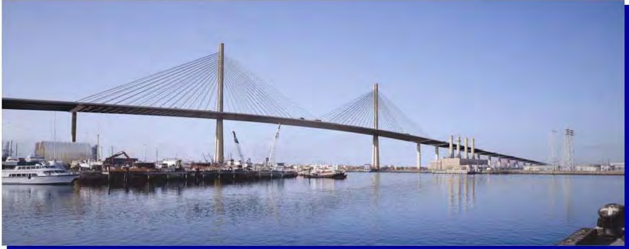
Single Mast Tower
