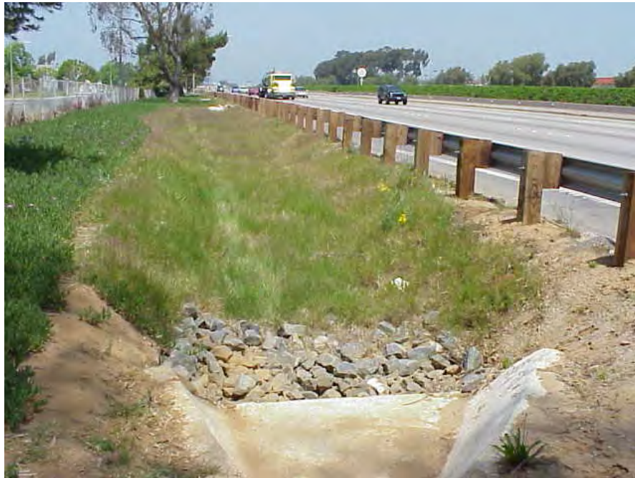
Exhibit 2.2.1-4 Typical Biofiltration Swale
