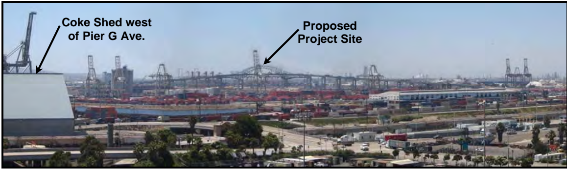
Exhibit 2.1.7-2 Viewpoint 1 – View to the Northwest from the Port Administration Building
