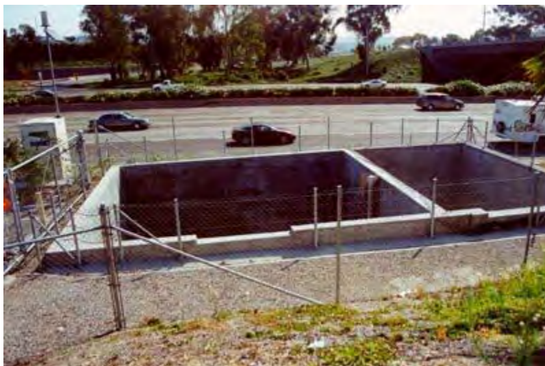
Exhibit 2.2.1-5 Typical Media Filter (Austin Sand Filter)
