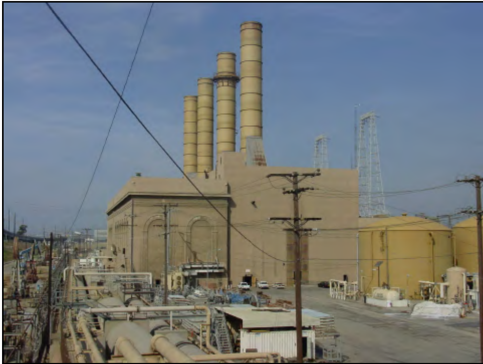
Exhibit 2.1.8-1 Photograph of Edison Power Plant No. 3
