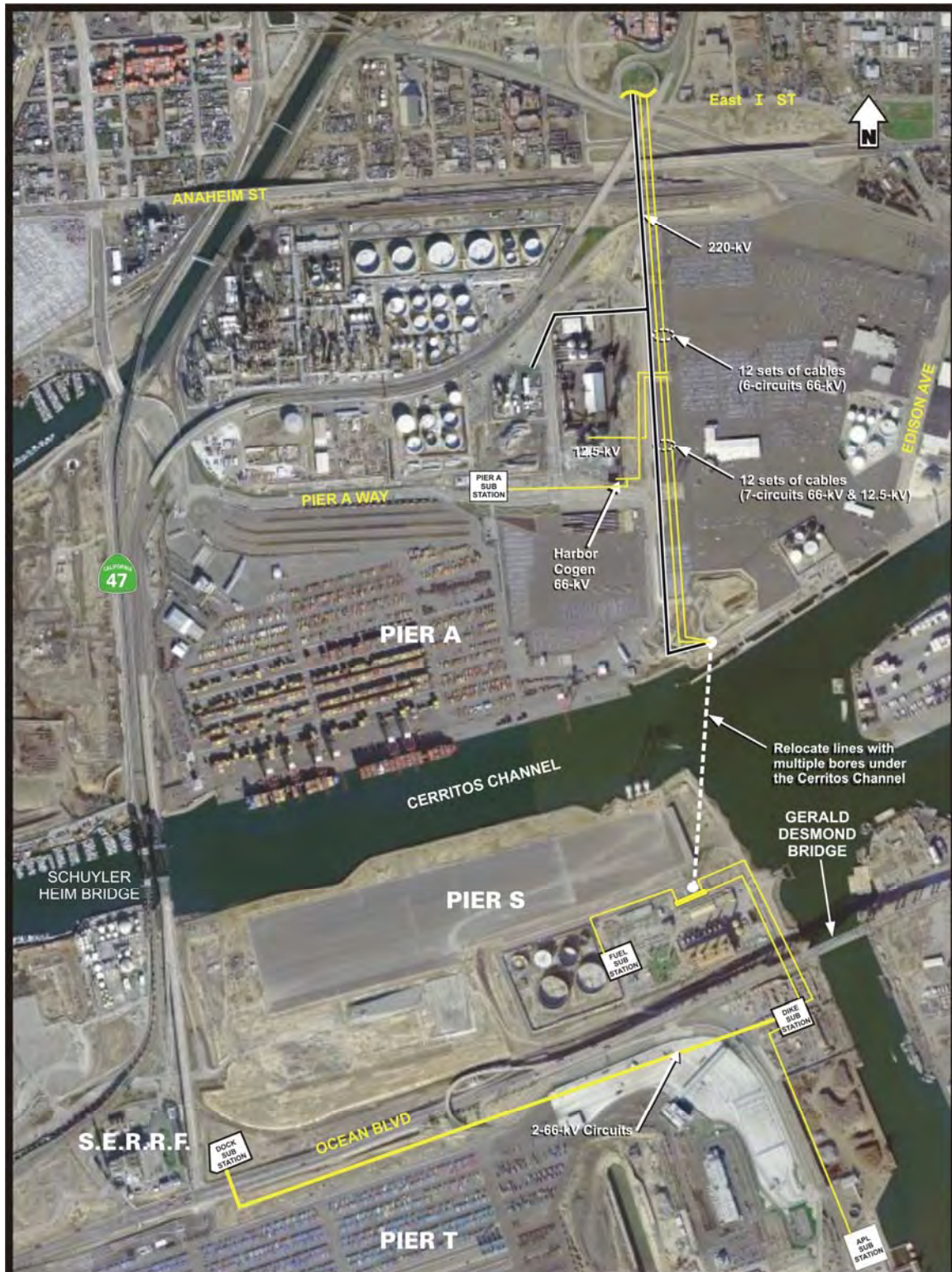
Figure 3 Under the Cerritos Channel
