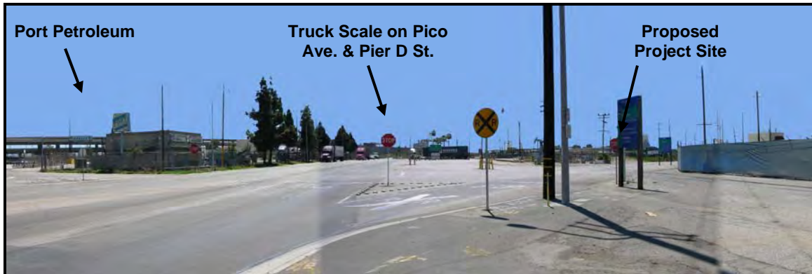
Exhibit 2.1.7-4 Viewpoint 3 – View to the South on Pico Avenue North of Pier D Street
