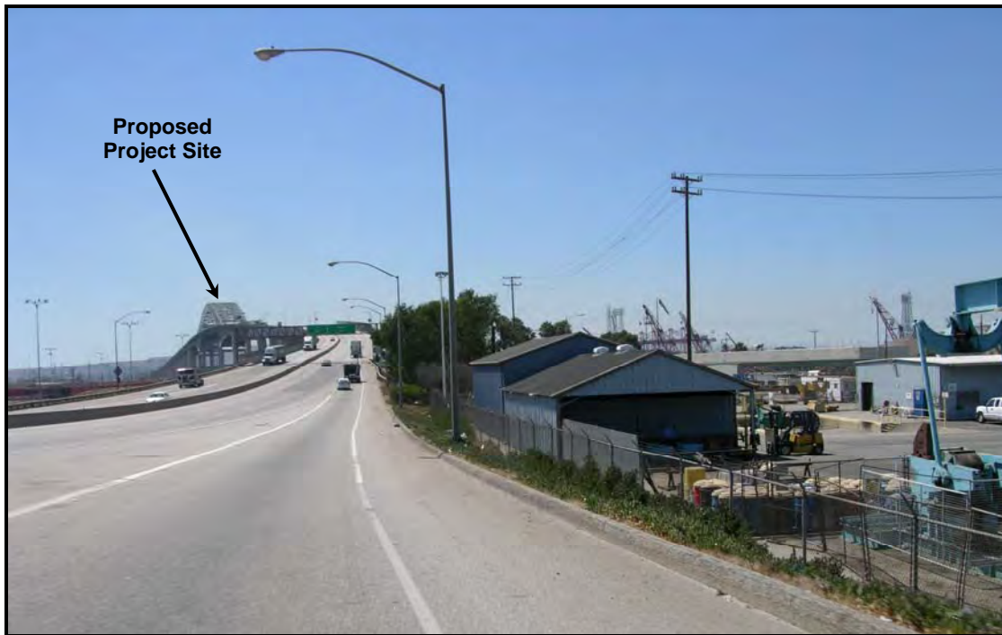
Exhibit 2.1.7-10 Viewpoint 9 – View to the West on Pico Avenue On-Ramp to Ocean Boulevard
