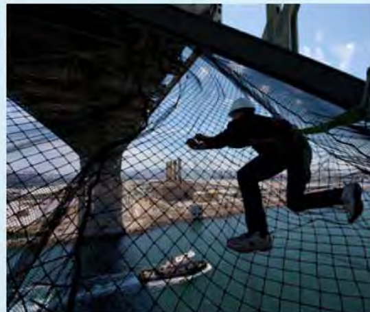
A worker repairs netting (known as a “diaper”) below the bridge that stops broken pieces of concrete from falling.
