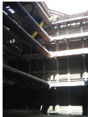
Soldier Piles and Lagging With Cross Bracing, Mariachi Plaza, Gold Line
