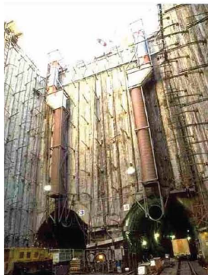
Secant Pile Walls, Barnsdall Shaft, Hollywood
