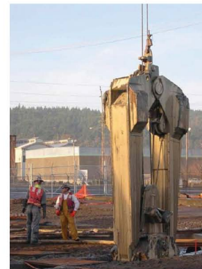
Slurry Wall Excavation, Portland, OR
