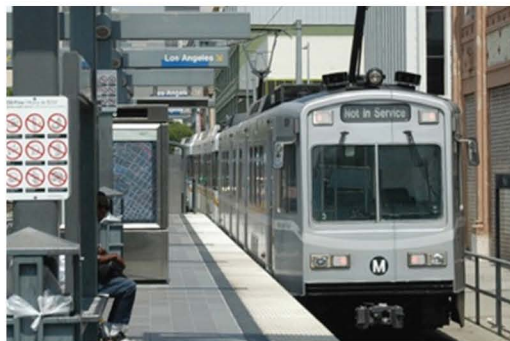
Figure S-13 Example of Light Rail Transit (LRT)
