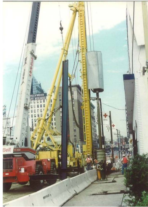
DEEP SOIL MIX WALL EQUIPMENT, HOLLYWOOD AND VINE STATION
