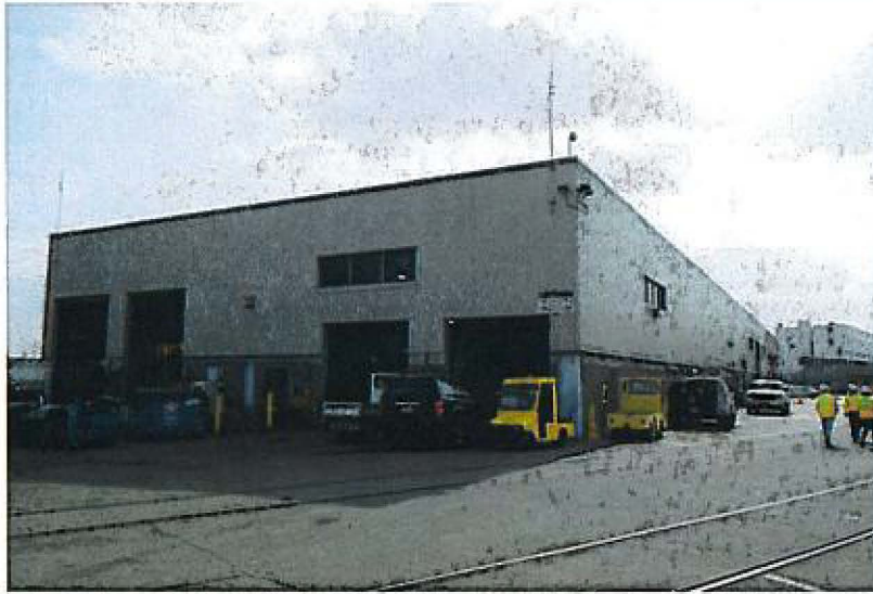
Plate 10. Overview of the central portion of the Project Area where P-19-002563 was previously encountered, view south, December 6, 2016, SAM_4502.
