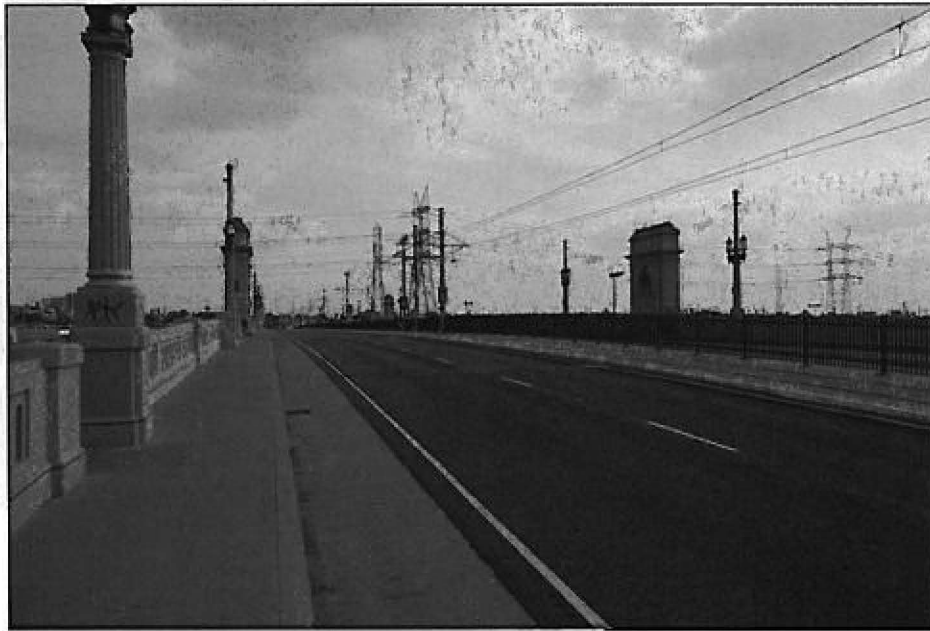
Photograph 1. Overview of top deck of First Street Bridge from north side, view southeast, December 6, 2016, SAM_4558.
