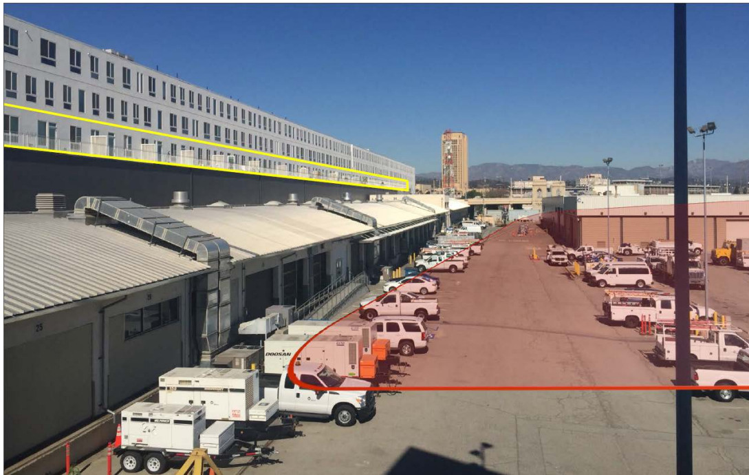
Figure 2. Relationship Between OSF Resident Balconies (Yellow Polygon) and Approximate Proposed Turnback Facility Site (Red Polygon)
