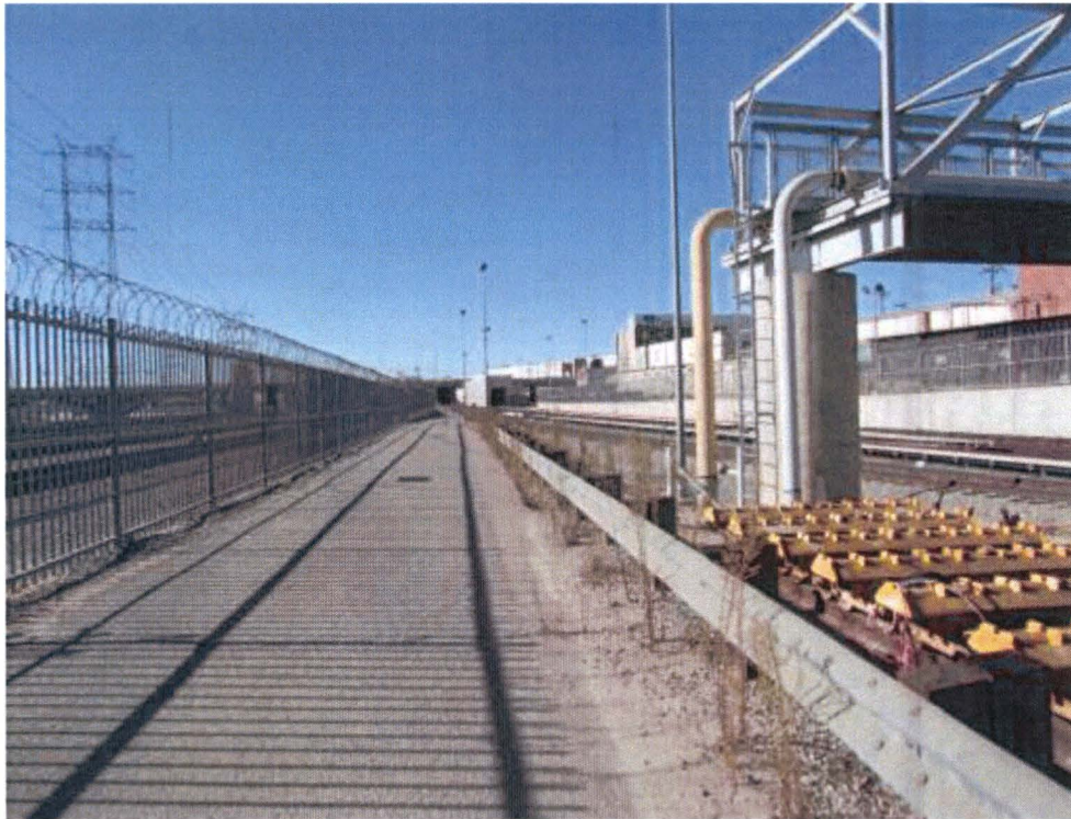
View facing south along Metro Division 20 access road (facing rail car wash in background). Two high-pressure natural gas pipelines are shown passing via an overhead structure over tracks (right).
