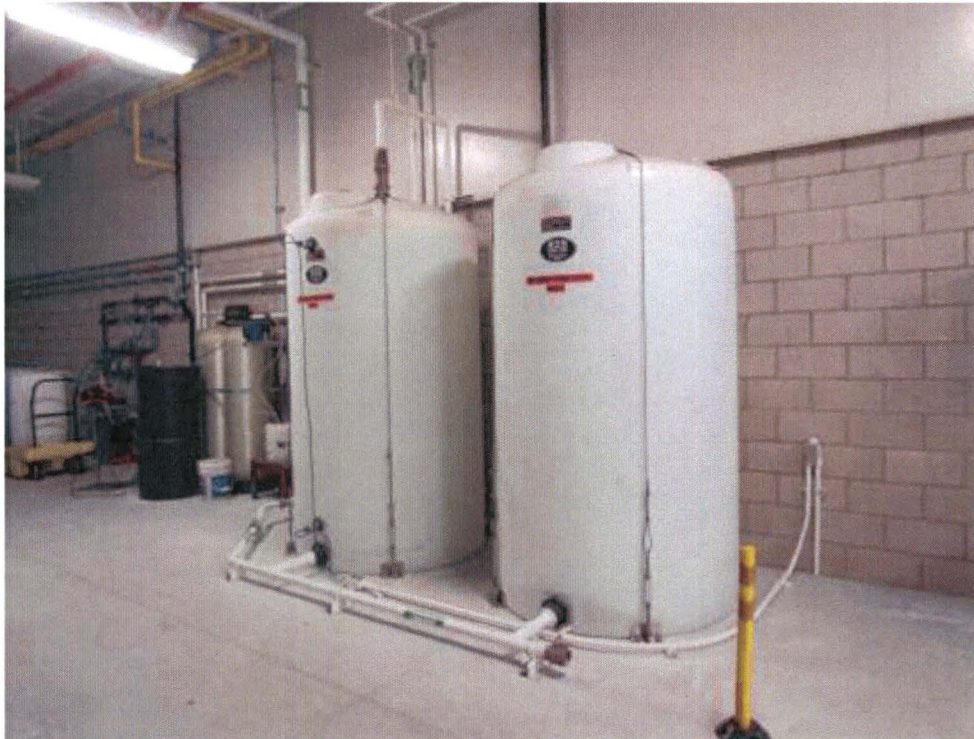
Softener system located inside the Metro Division 20 rail car wash building.
