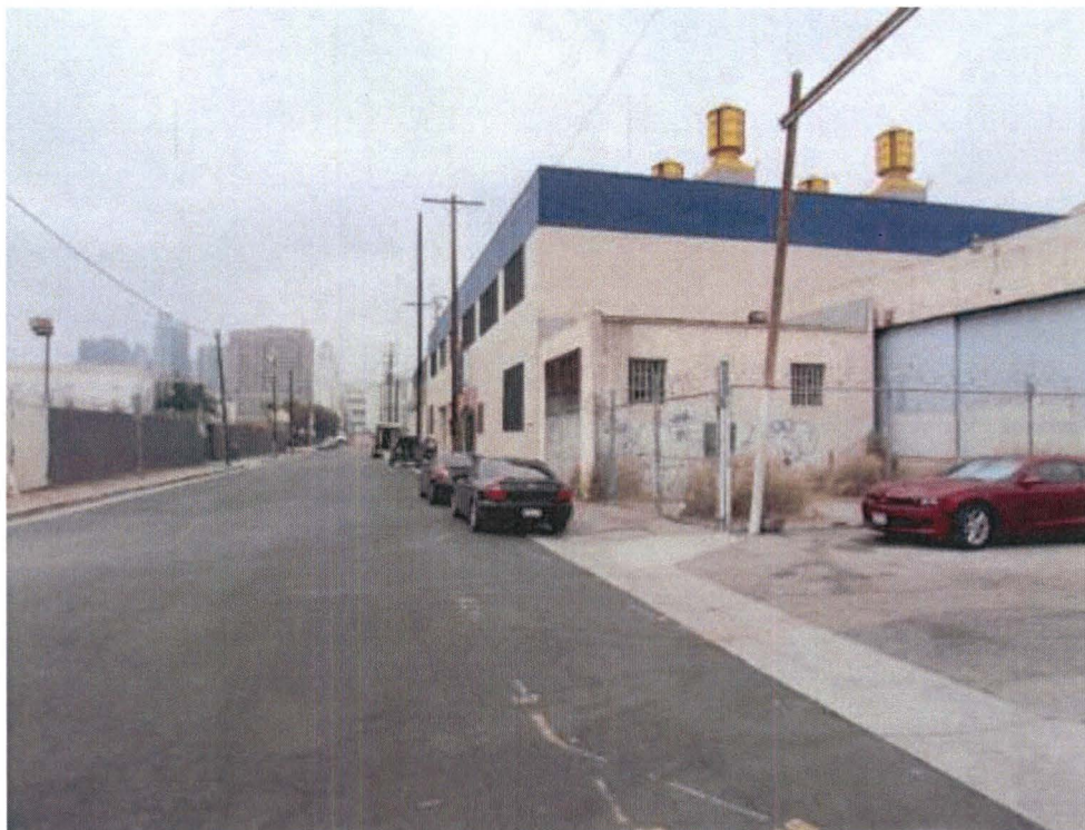
View facing west along Commercial Street at the northern end of the Site (right). Adjoining industrial facilities to the north are shown right.
