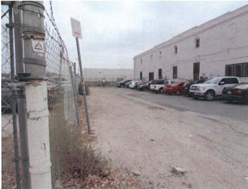
View facing east at Banning Street. The National Ice & Cold Storage facility is north (left) and the Site building at 1001 East 1 st Street is shown south (right).
