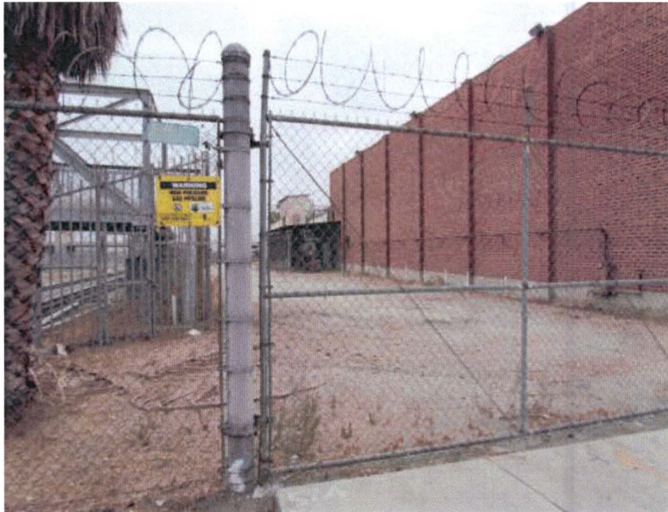
View facing south from Jackson Street behind the National Ice & Cold Storage facility. The high-pressure natural gas line structure over the tracks (left) crosses behind this facility.
