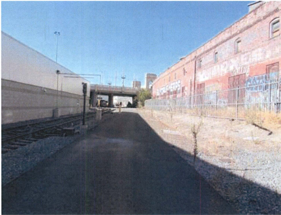
View facing south between the Metro Division 20 rail car wash building and on-Site building located between Banning Street and 1 st Street (shown in background).
