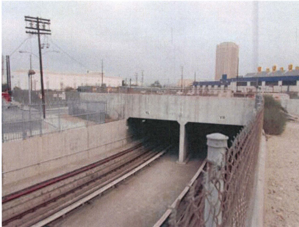
View north of the Metro Red and Purple Line subway portal.
