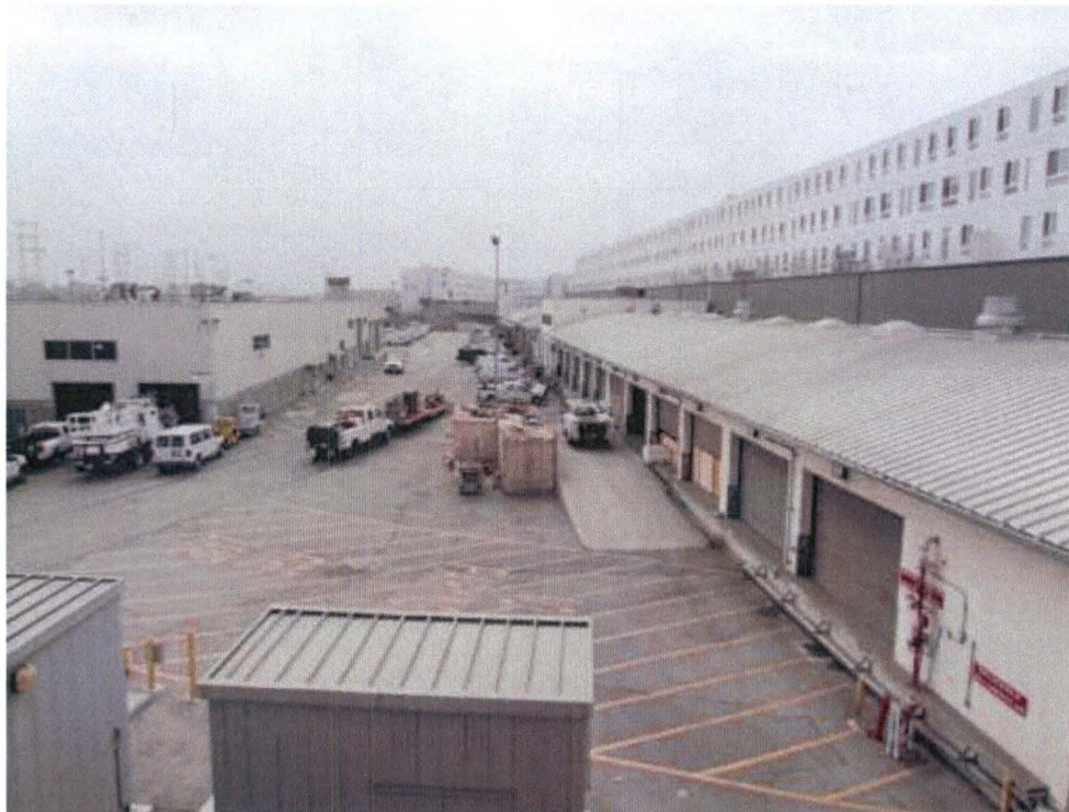
View facing south from 1 st Street at Metro Division 20 Facility. Building 61A is shown right; Building 61B is shown left.
