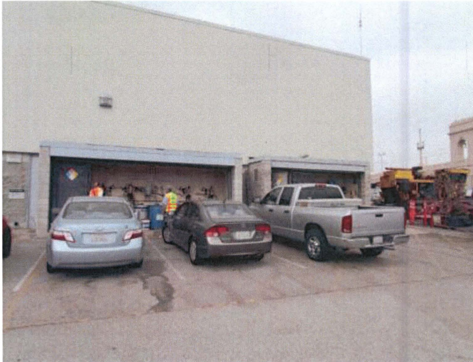
View of the hazardous materials storage area and battery charging station located outside the northeastern corner of Metro Division 20 Building 61 B.
