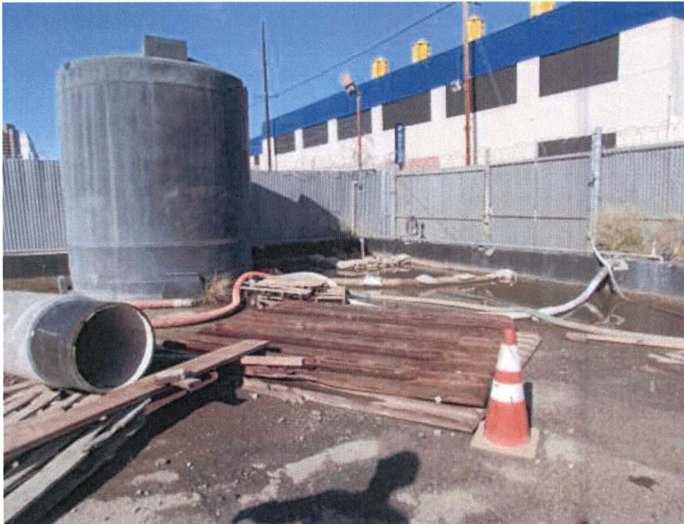
View of northwestern corner of Metro Temporary Storage Lot (840 East Commercial Street). AST shown contains flood water that is being drained to the street curb and gutter system.
