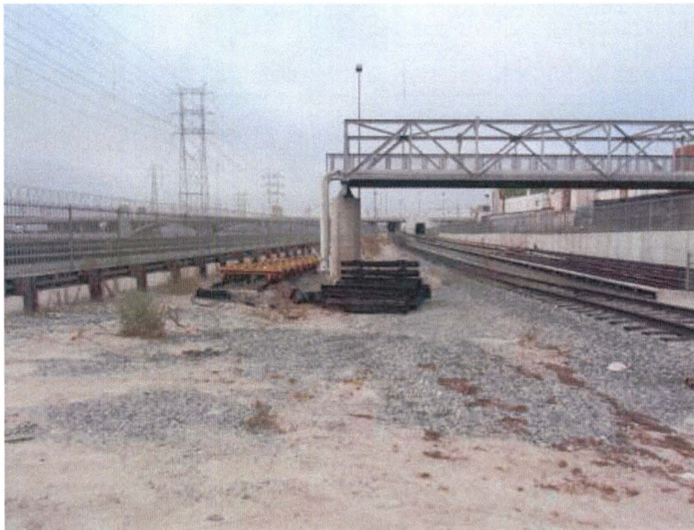
View facing south at Metro Red and Purple Line tracks and high-pressure natural gas pipeline structure over tracks.
