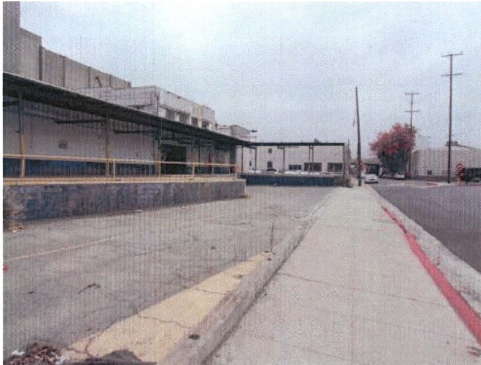
View facing south along Center Street from near the southern portion of the National Ice & Cold Storage facility. The Site building at 1001 East First Street (just south of Banning Street) is shown in background.
