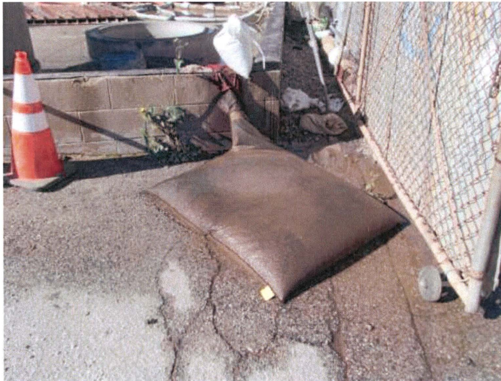
View of a "D-Watering Bag" through which water from the AST on the northwest corner of the property filters through prior to being discharged to the curb and gutter system.
