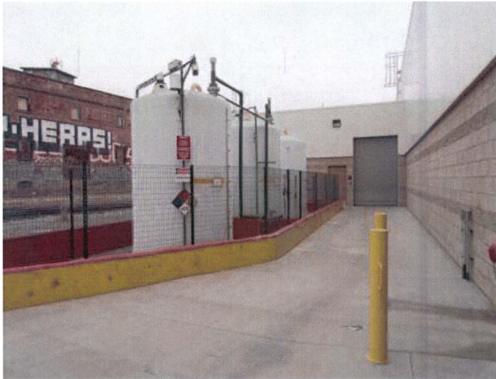
View of aboveground storage tanks outside the southwestern portion of the rail car wash building. The tanks contain acid soap and a cleaner foaming agent. One tank is empty.
