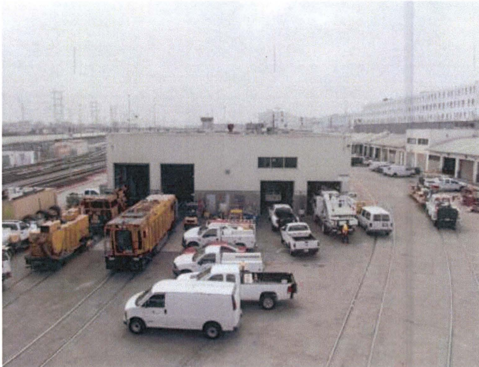
View of Metro Building 61B facing south from 1 st Street. Repair shop service bays are shown at northern end of building. Rail spurs are shown on Site.
