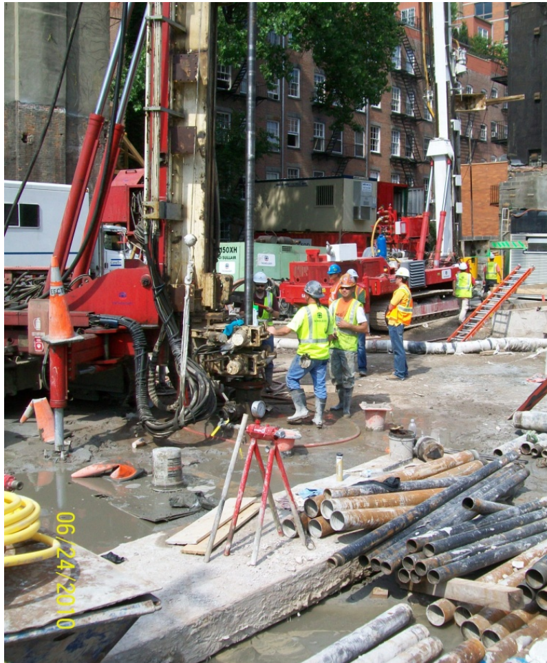
Figure 4-8: Surface Jet Grouting Operation
