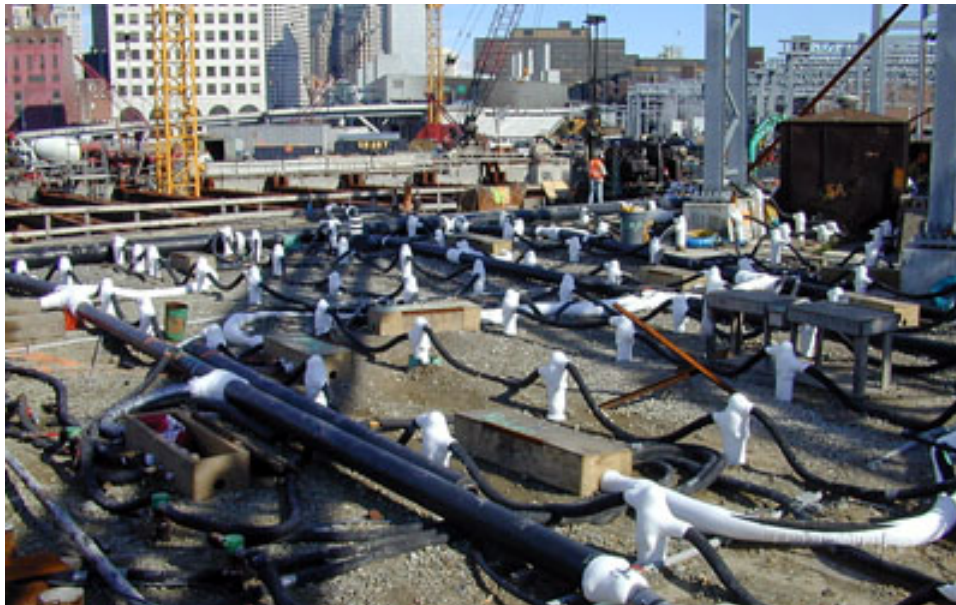
Figure 4-12: Ground Freezing Operation
