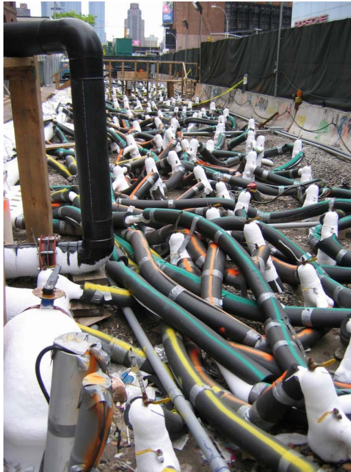
Figure 4-13: Freeze Pipe Array
