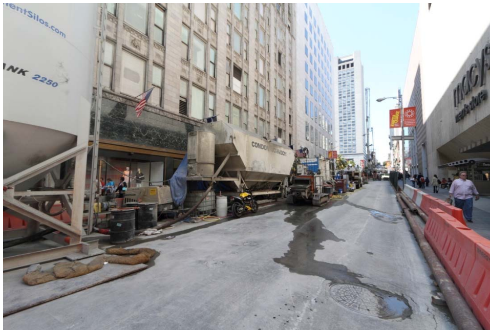
Figure 4-7: Staging for Jet Grouting Operation
