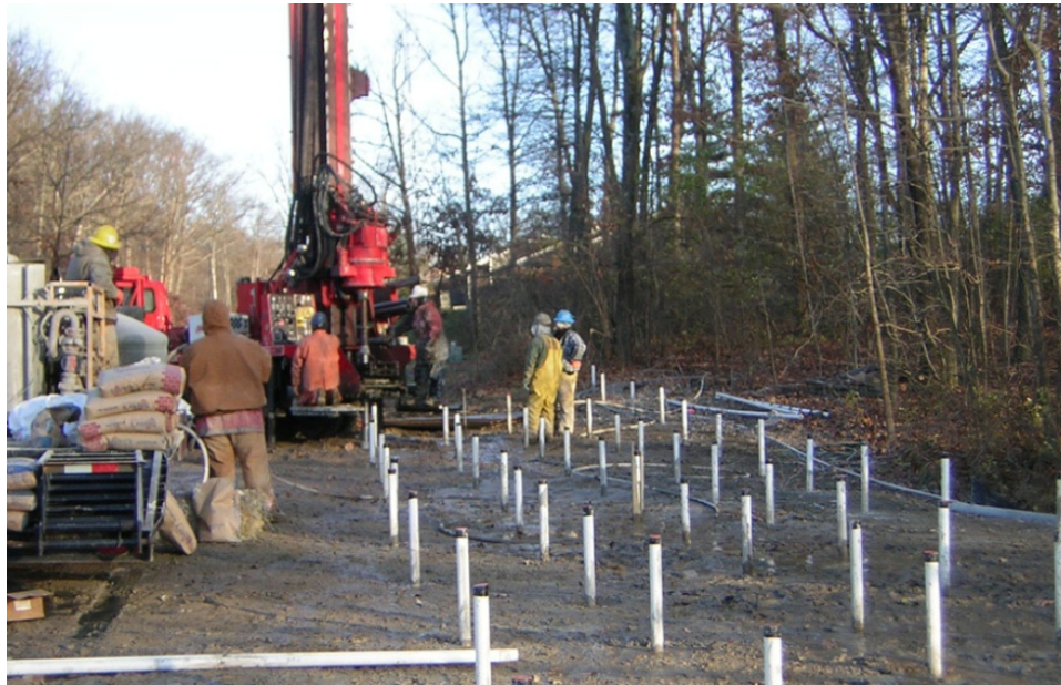
Figure 4-4: Permeation Grouting from Surface
