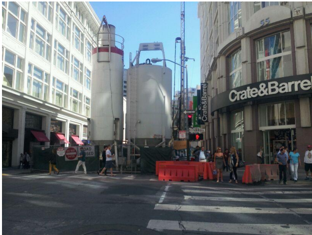
Figure 2.2-15: Grouting Equipment and Impacts (San Francisco, MUNI LRT Tunneling, 2013)
