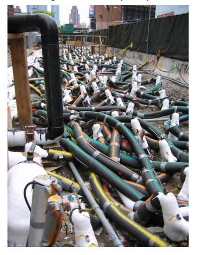
Figure 4-13: Freeze Pipe Array
