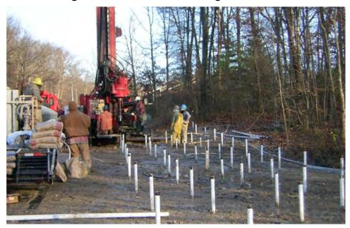
Figure 4-4: Permeation Grouting from Surface
