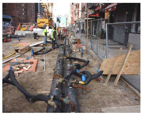
Figure 4-12: Ground Freezing Operation
