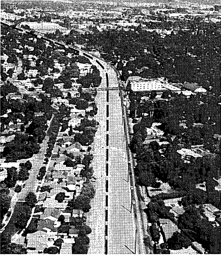
Air view looking east along the Topham SP right-of-way between White Oak and Reseda. Topham Street runs parallel to the railroad R.O.W. in this area.
