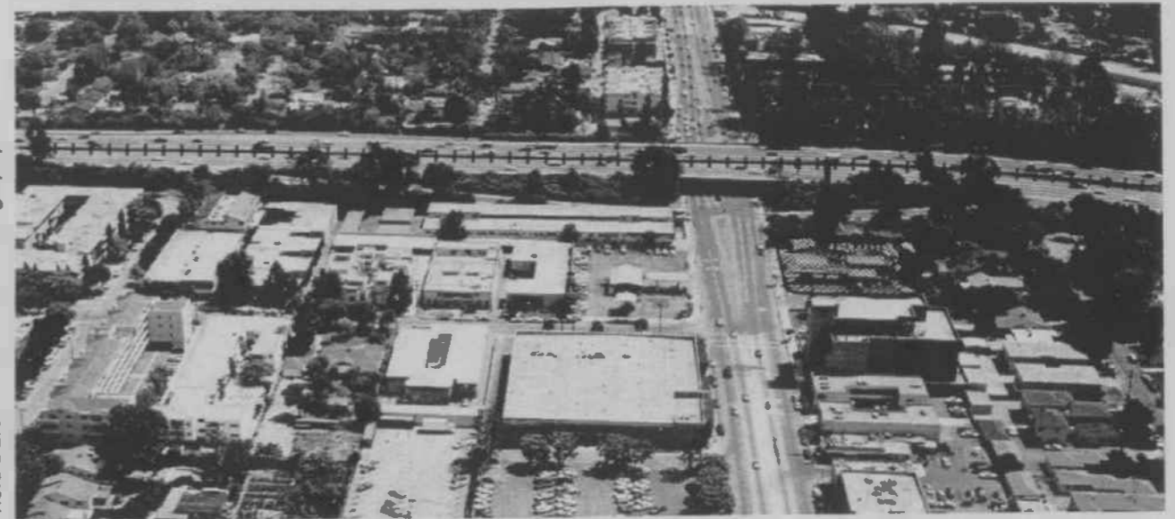
View looking South along Laurel Canyon Boulevard at the Ventura Freeway. Due to the need for station access and Kiss & Ride facilities, a gas station and one home would be displaced.
