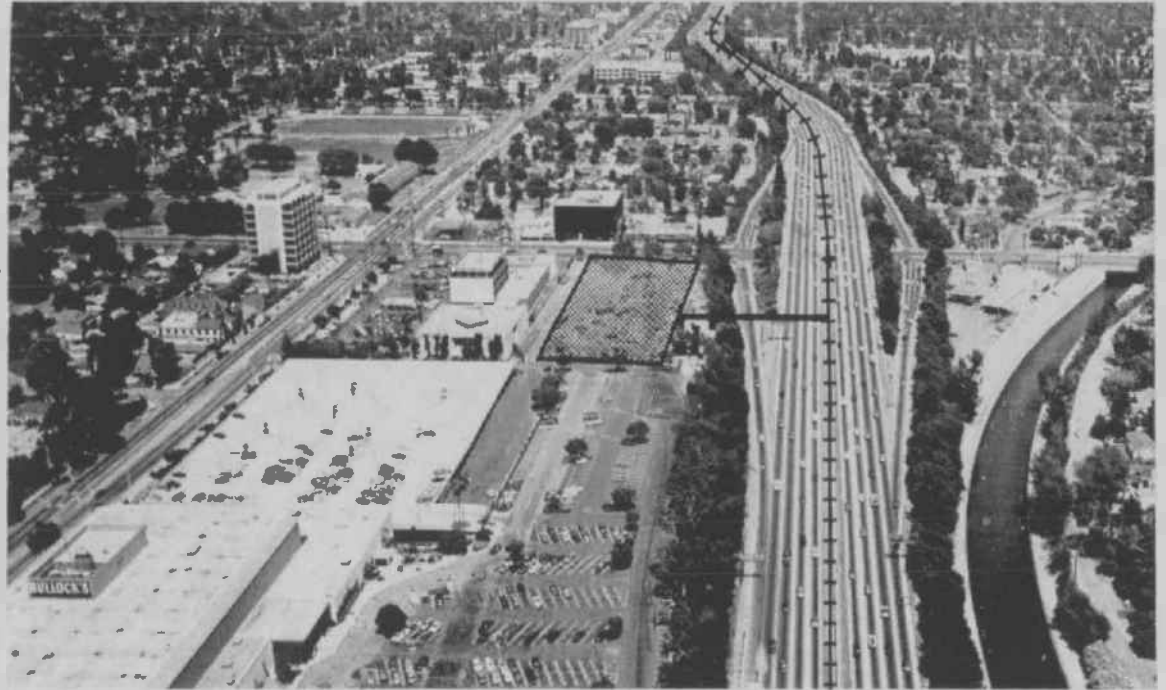
View looking East along the Ventura Freeway at Woodman Avenue. A parking structure for 500 cars would be used to provide station parking in what is now surface parking lots for the Fashion Square Shopping Center, seen along Riverside Drive on the left of the photo.
