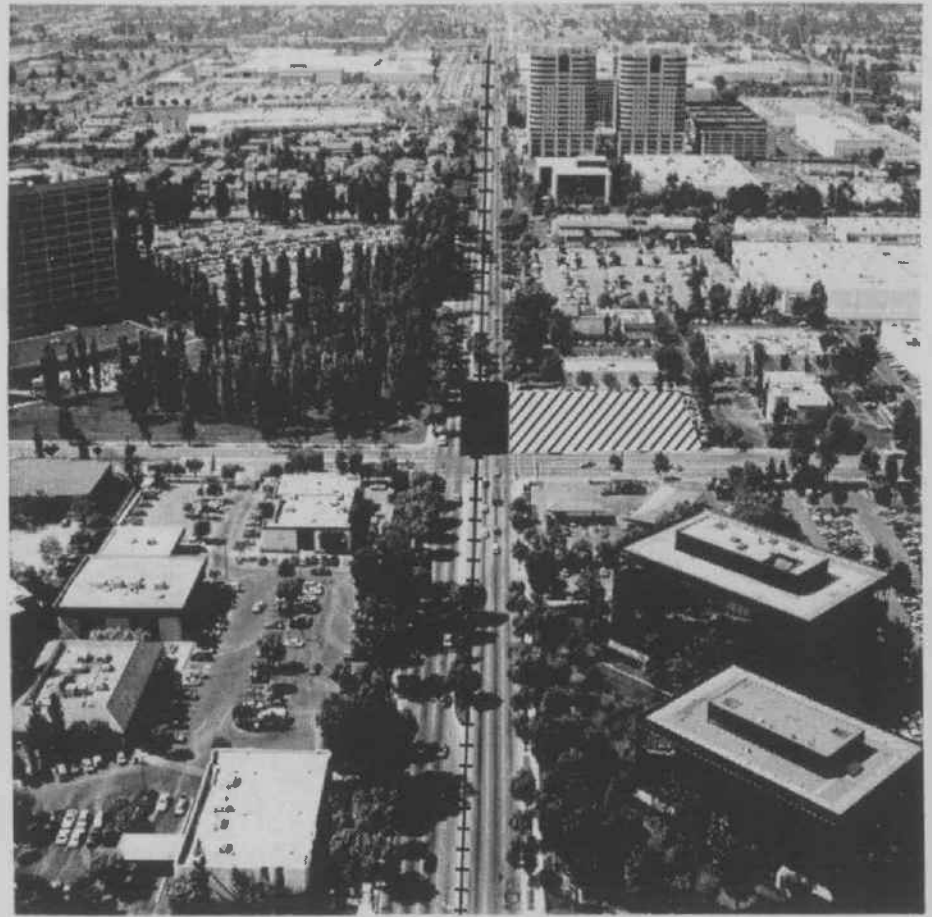
View look north along Canoga Avenue at Oxnard Street. Gas stations are located on the northeast and southeast corners of this intersection while a commercial bank is located on the southwest corner. The heavily landscaped area on the northwest corner is part of the Blue Cross office complex seen at the left of the photo. This station site is near the geographic center of the Warner Center high-rise development area.
