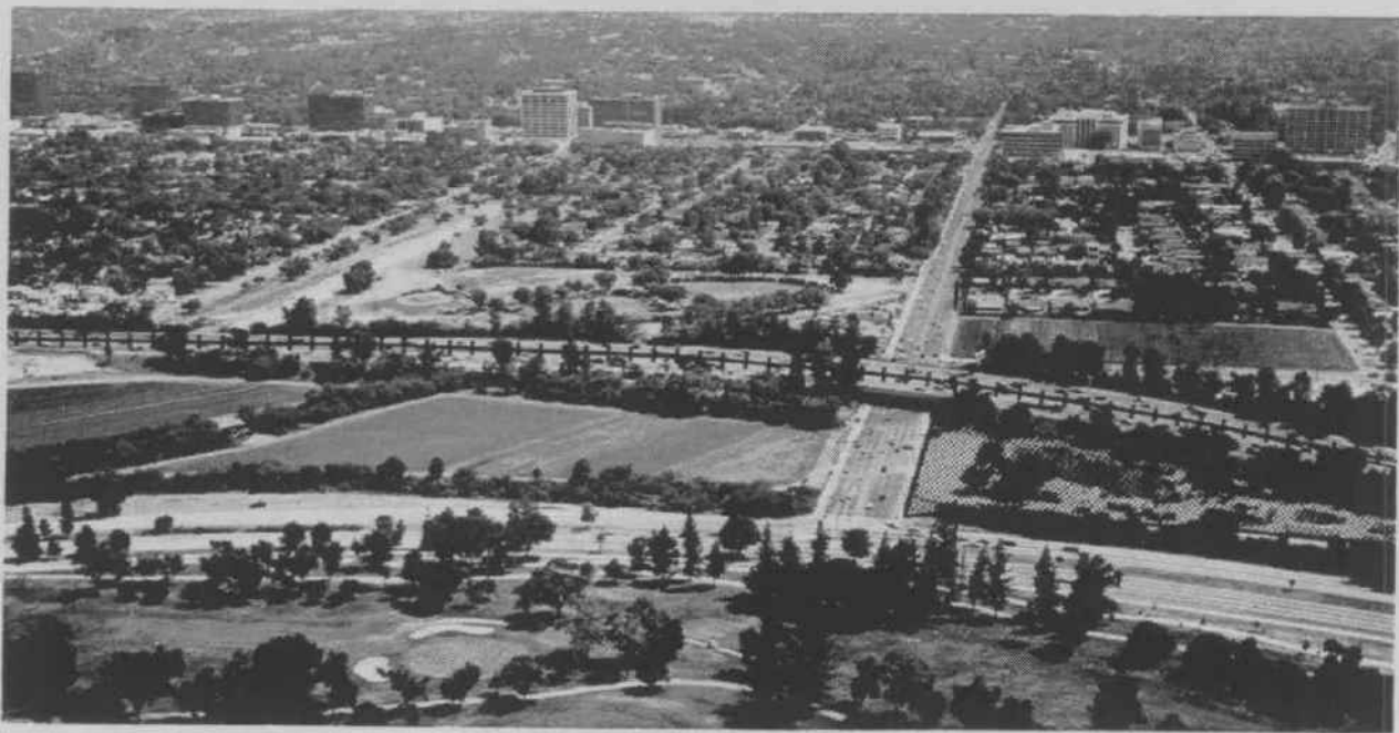
View look south along Hayvenhurst Avenue from above the Sepulveda Basin. The proposed station parking lot would displace a commercial produce vendor (Tapia Brothers).
