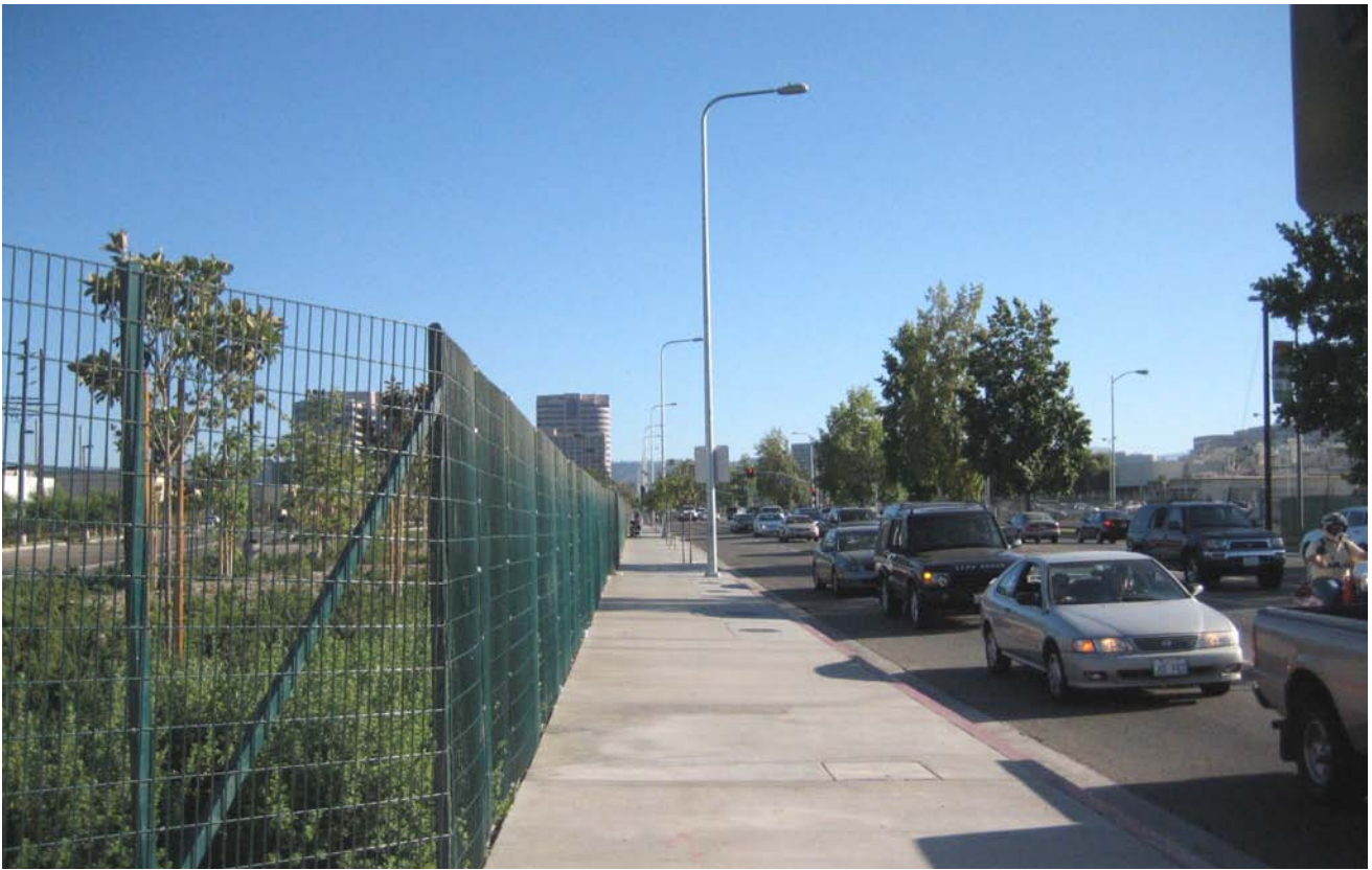
The park-and-ride lot for the existing MOL Canoga Station screened from Canoga Avenue by a fence and landscaping
