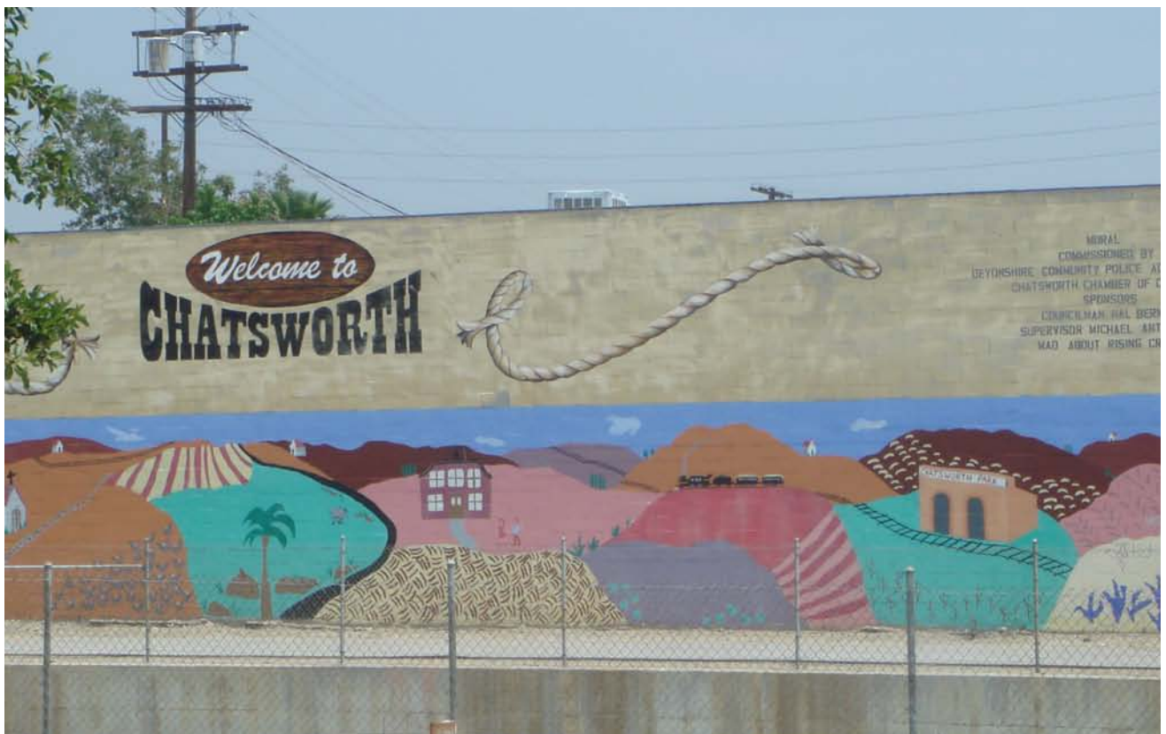
View of the Brown's Canyon Wash and the mural on the concrete wall
