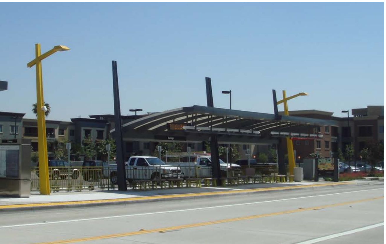
View of the existing MOL Busway in the foreground, the park-and-ride lot in the middle ground, and the Archstone Warner Center Apartments in the background
