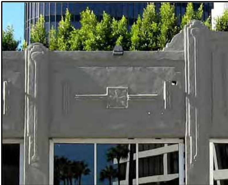
Bas-relief panel over windows on east elevation.
