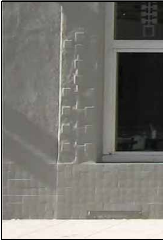
Decorative element on east elevation of the subject building.
