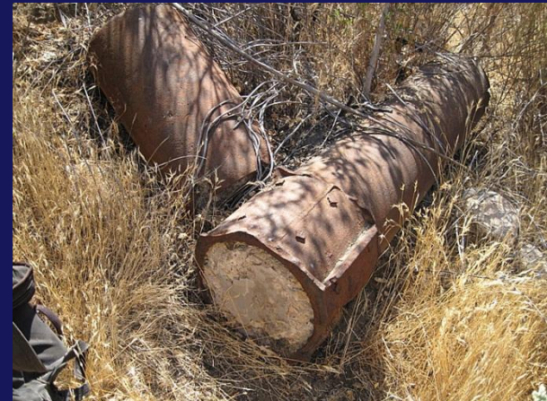
Abandoned, cemented oil well in Whitney Canyon, near Los Angeles
