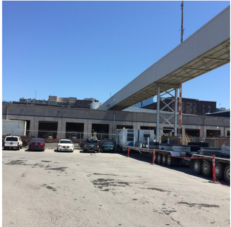
Figure 4-30. Typical Enclosed Conveyor
