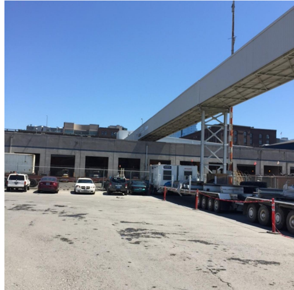
Figure 2-17. Typical Enclosed Conveyor
