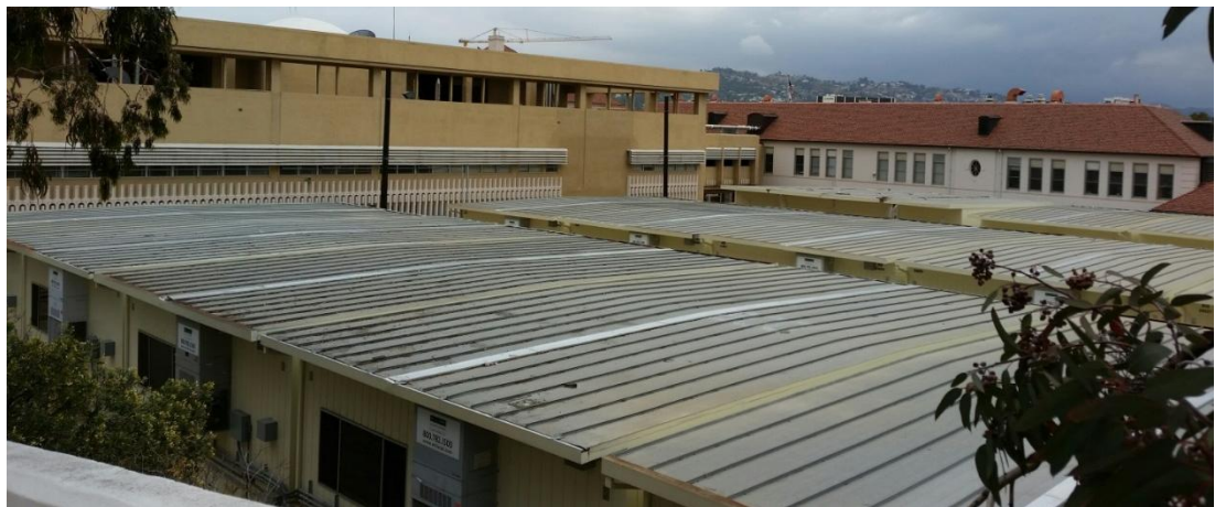
BHHS, temporary classrooms photographed May 2016
