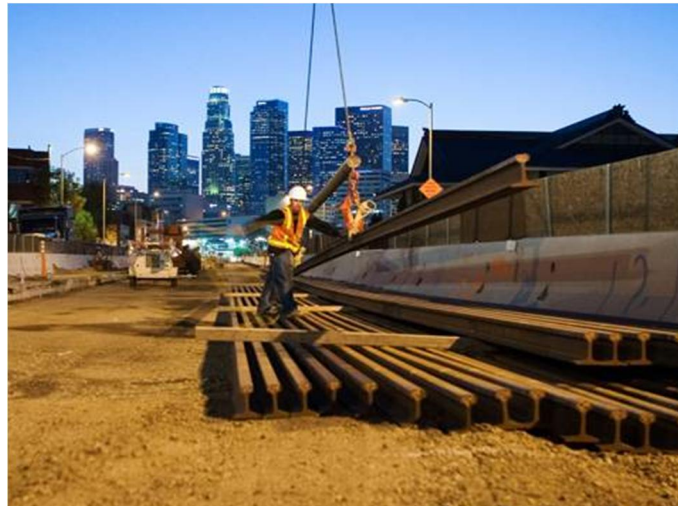
Figure 4-25. Off-Street Construction Area on Metro's Gold Line Eastside Extension
