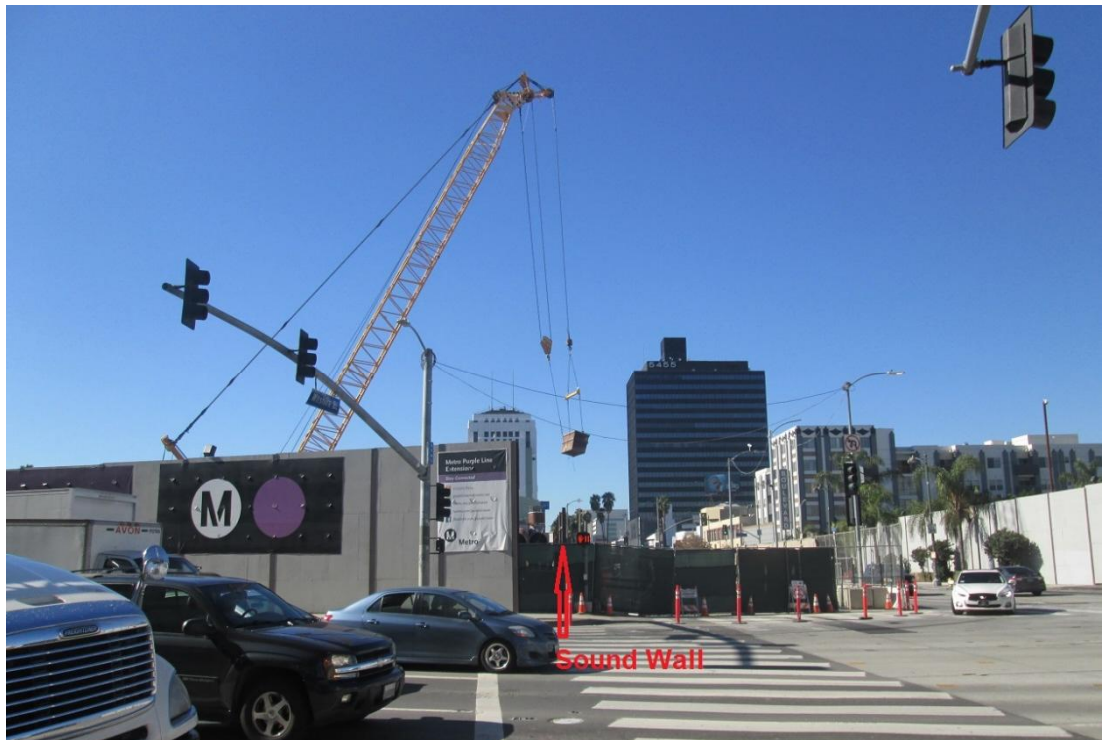
Figure 4-29. Crane at the Wilshire/La Brea Muck Shaft
