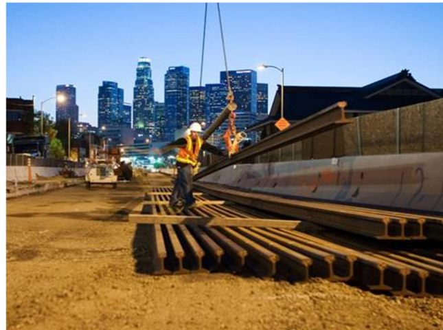
Figure 4-26. Off-Street Construction Area on Metro’s Gold Line Eastside Extension
