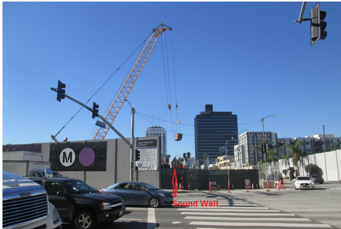
Figure 4-30. Crane at the Wilshire/La Brea Muck Shaft
