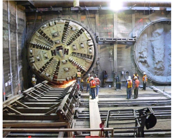
Figure 4-24. Twin Tunnels on Eastside Extension
