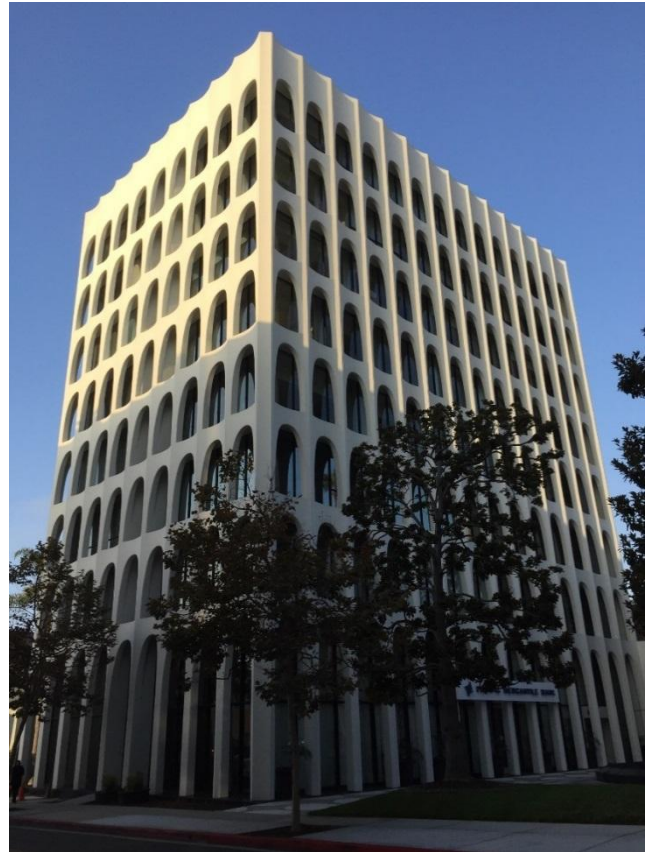
Figure 5-2. Perpetual Savings Bank Building
