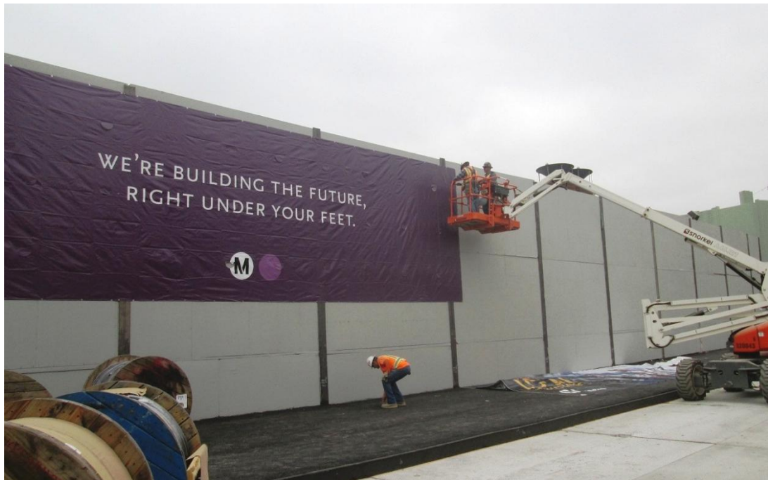
Figure 2-16. Typical 20-foot Noise Barrier at Construction Staging Areas
