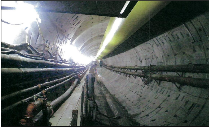
Figure E-7. Typical TBM Tunnel during Construction
