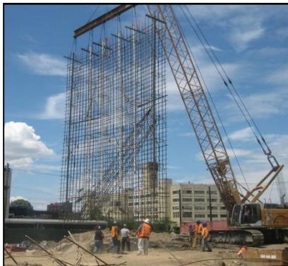
Figure E-4. Rebar Cage for Typical Slurry Wall Panel
