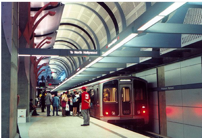
Figure 2-40: Existing Metro HRT Train and Station
