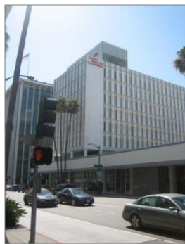
Figure 4-72. Union Bank Building
