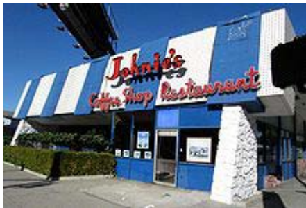
Figure 4-67. Johnie's Coffee Shop exterior in 2007
