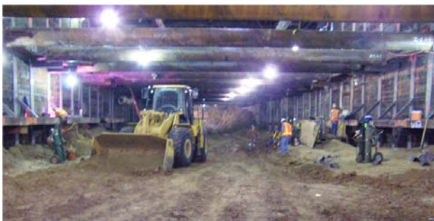
Figure 4-83. Construction Activities below Concrete Decking
