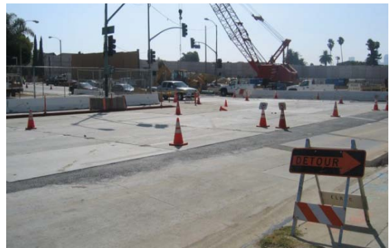
Figure 4-82. Concrete Decking on Street
