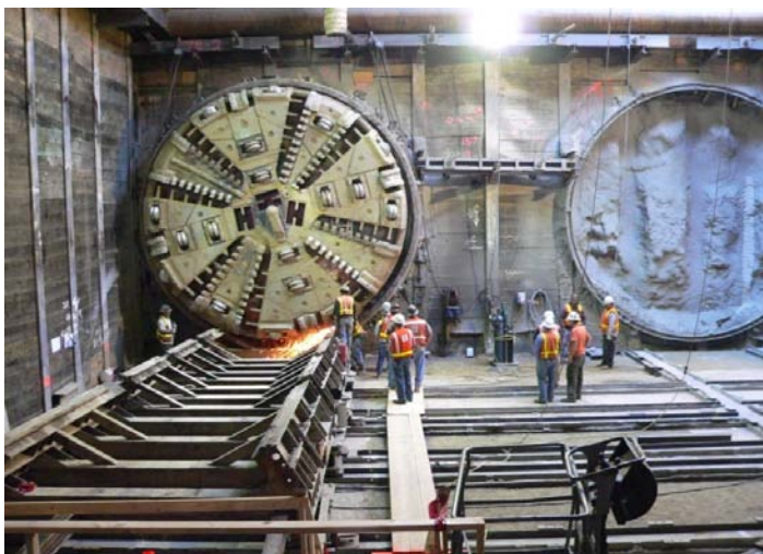
Figure 4-77. Twin Tunnels on Eastside Extension
