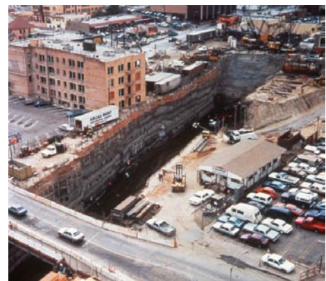
Figure 4-84. Off-Street Station Box Excavation
