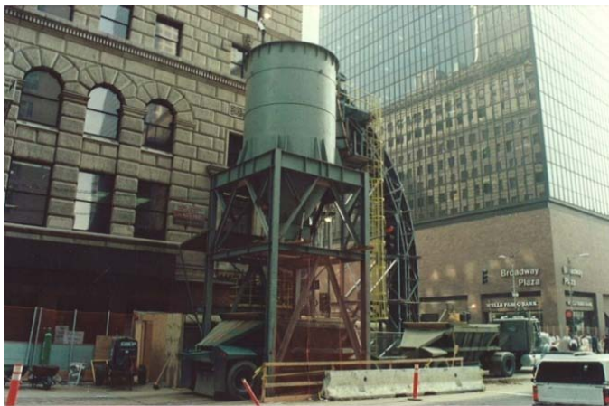
Figure 4-86. On Street Construction Area Used for 7 th /Metro Station
