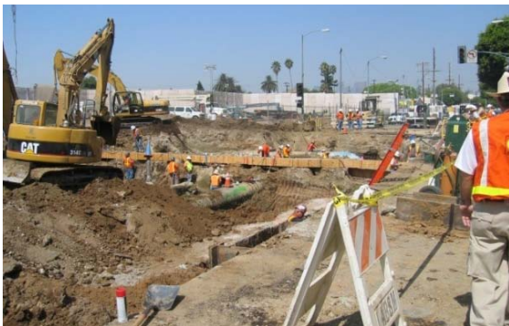
Figure 4-81. Typical Street Excavation
