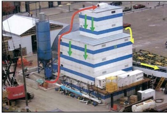
Figure 4-21: Typical Slurry Treatment Facilities (Stacked Configuration)
