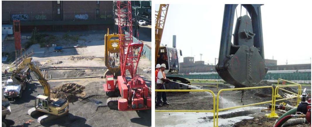
Figure 4-6: Typical Slurry Wall Panel Excavation
