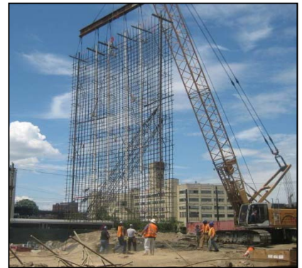
Figure 4-7: Rebar Cage for Typical Slurry Wall Panel
