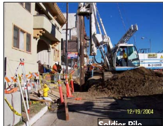
Figure 4-3: Drilling for Soldier Pile Installation
