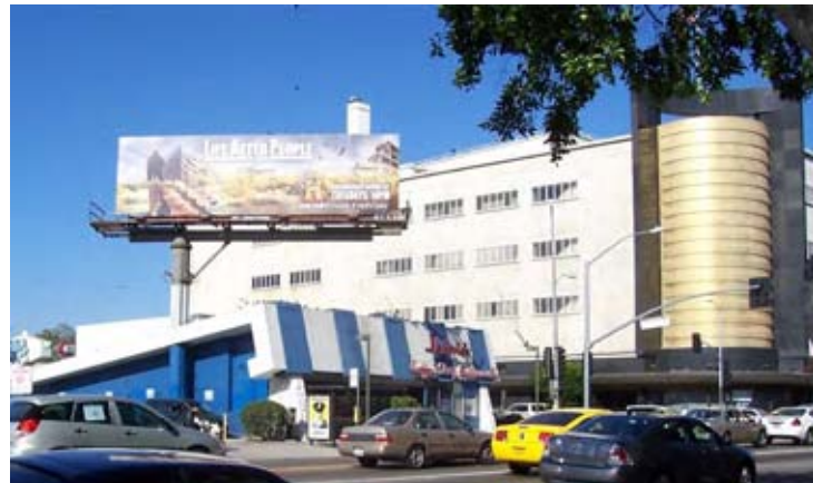
Figure 4-6. View of Johnie’s Coffee Shop and May Company at Wilshire Boulevard and S. Fairfax Avenue
