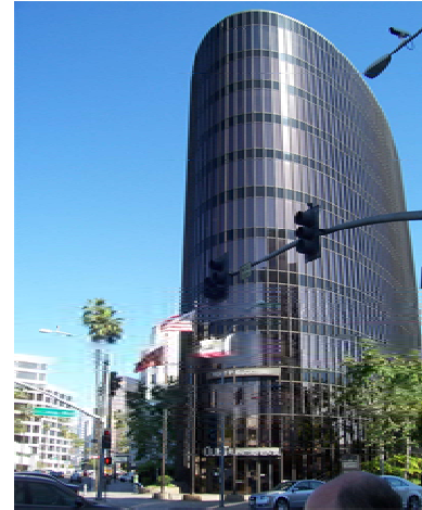
Figure 4-8. View of the Flynt building at Wilshire Boulevard and S. La Cienega Boulevard
