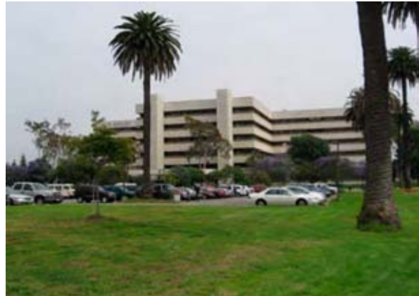
Figure 4-18. View looking south toward the VA Hospital and parking lot
