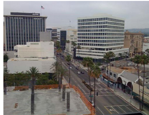
Figure 4-10. View looking west on Wilshire Boulevard
