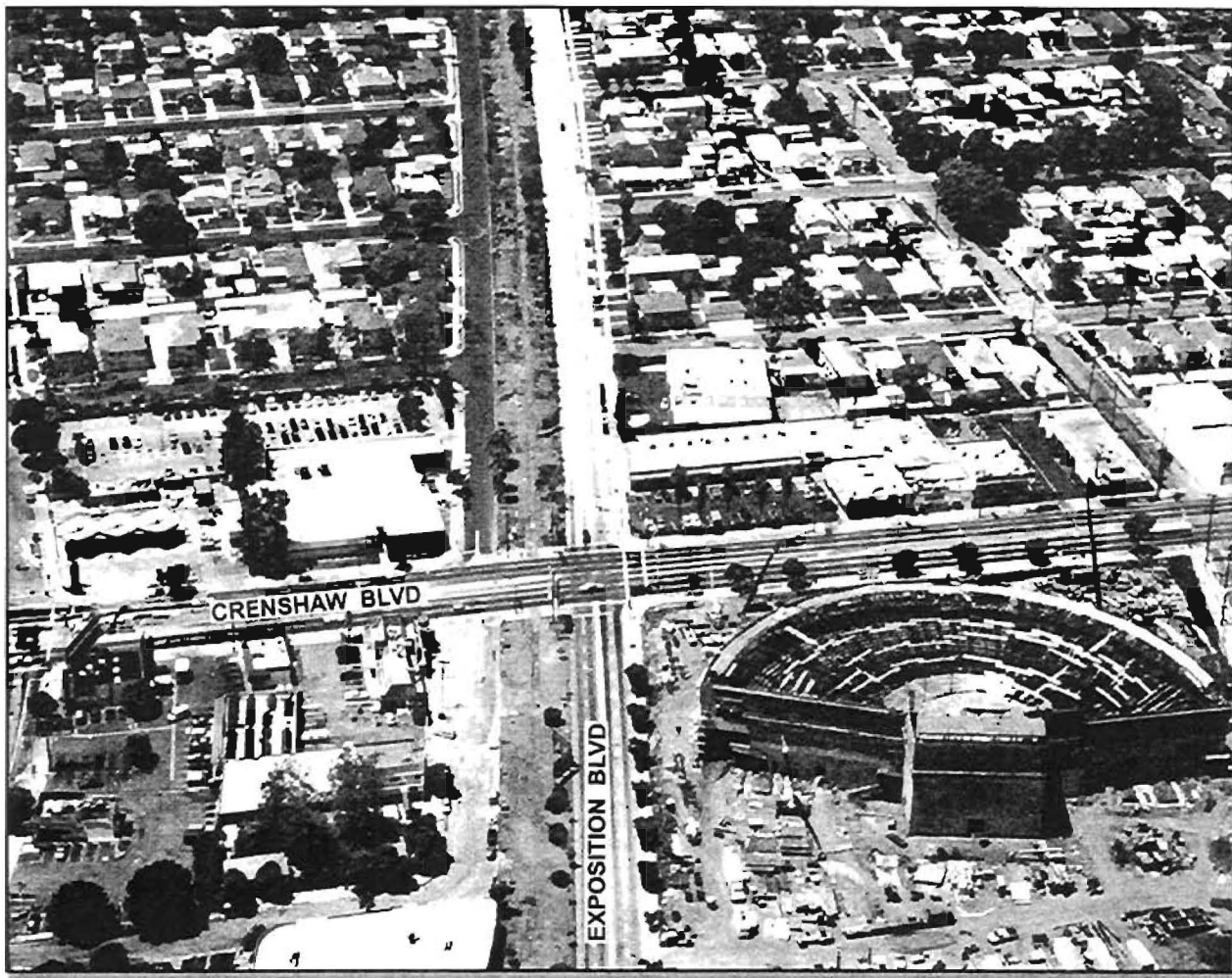
Looking West Along Exposition Boulevard at Crenshaw Boulevard
