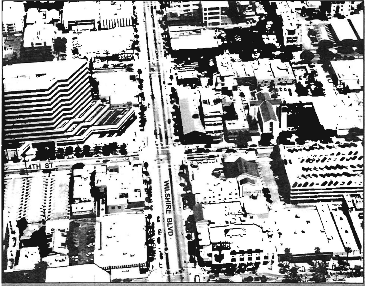
Looking East Along Wilshire Boulevard near 4th Street in Santa Monica
