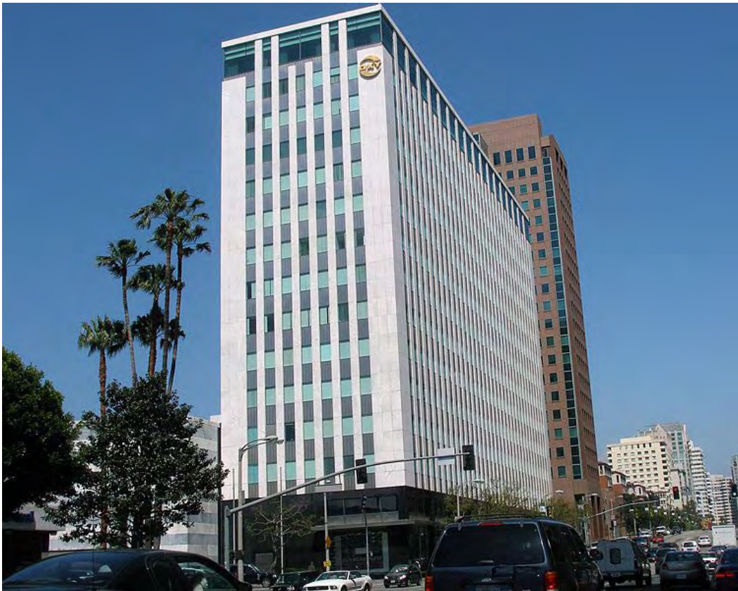
Figure 14: Kirkeby Building Westwood (Occidental Petroleum Headquarters)
