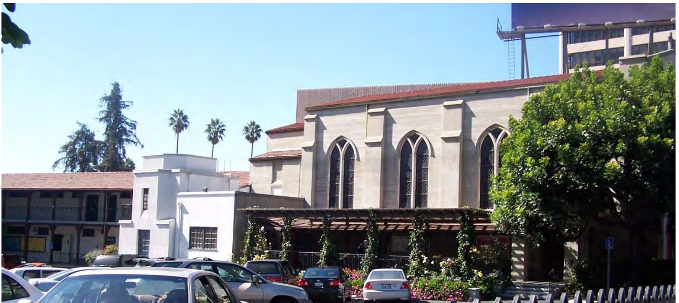
Figure 2: East elevation of Church and later addition, view southwest.
