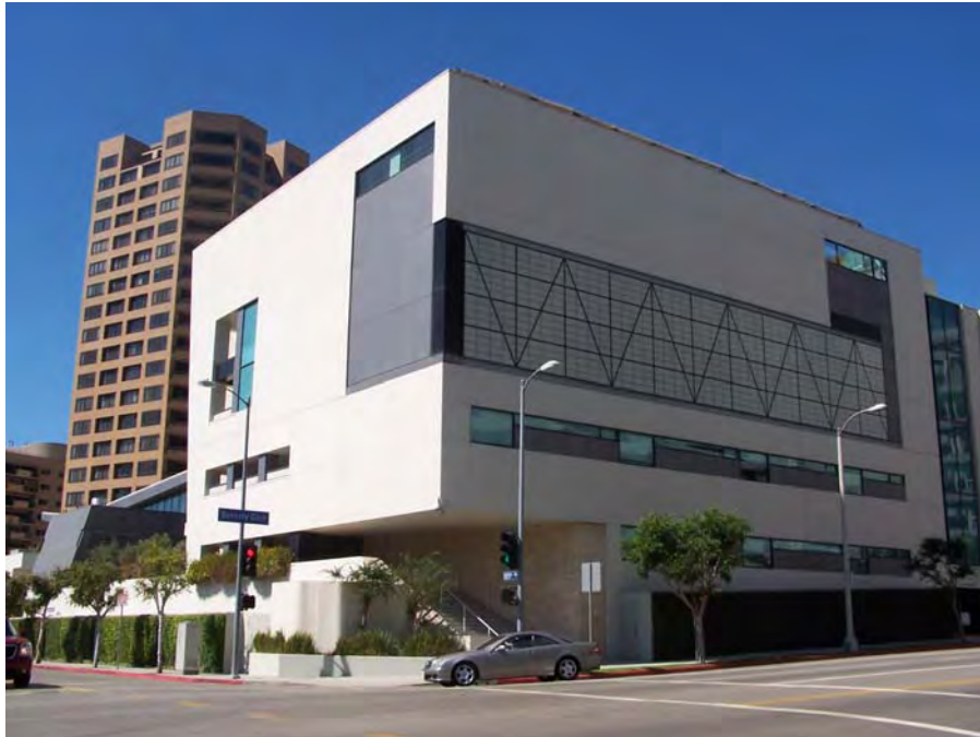
Figure 3: View northwest, 1998 addition.
