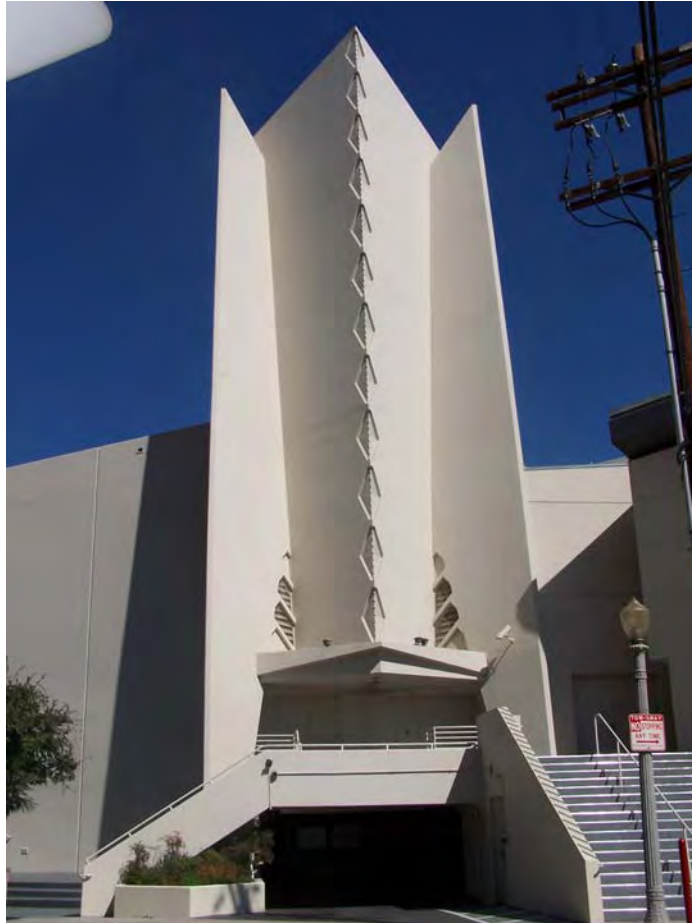
Figure 1: The original primary entrance to the Sinai Temple, located on the west elevation, view northwest.
