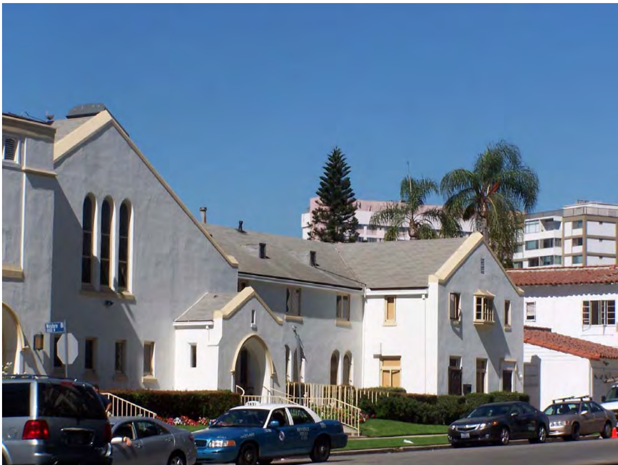
Figure 1. East elevation, view northwest.
