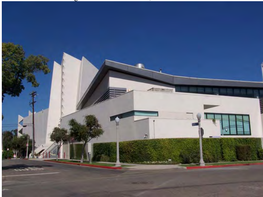
Figure 4: View north/northeast, 1998 addition.
