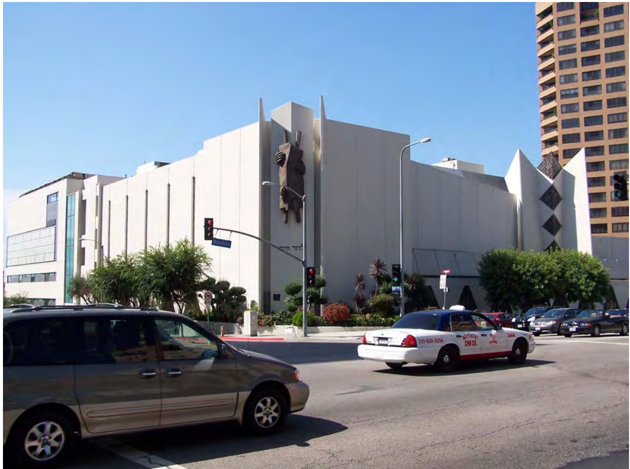
Figure 2: View southwest, original building (right), 1968 addition (center), 1998 addition (left).
