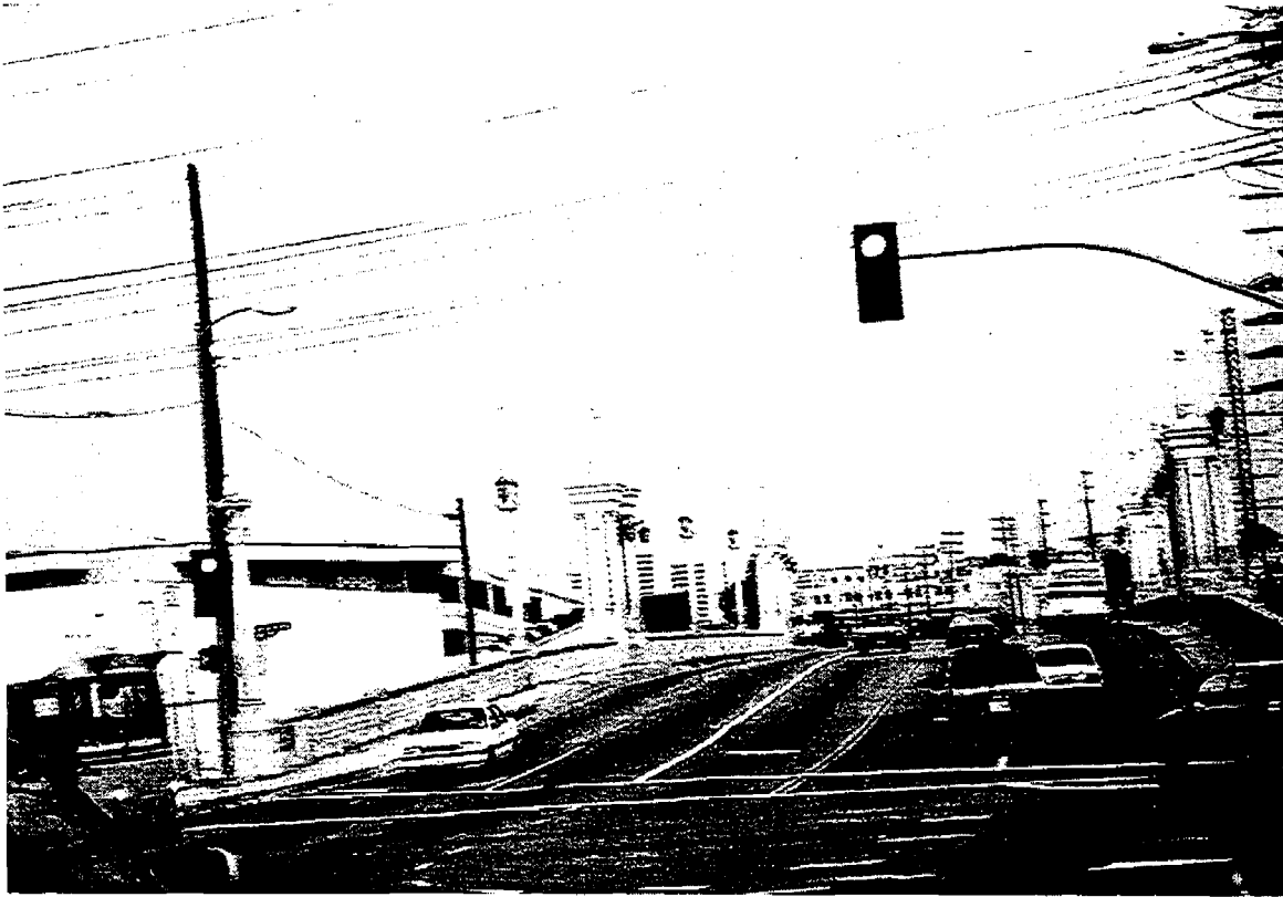
Figure 5-51: Macy Street Viaduct
