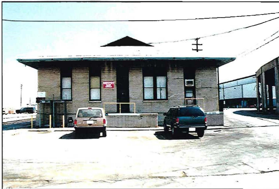
Master mechanic and supervisor's offices
