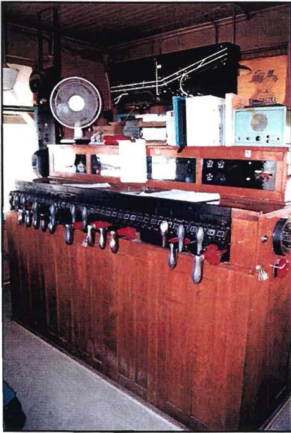
G-R-S electric interlocking machine, 1906 model, Redondo Junction Tower
