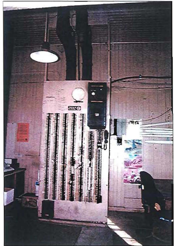
Lower floor interior, Redondo Junction Tower
