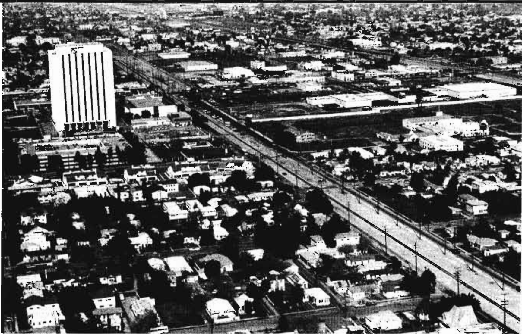
Bird's eye view of the SPTC right-of-way looking north at downtown Compton in 1984.
