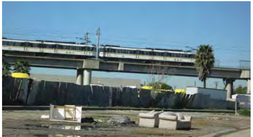
Littered vacant land east of Slauson Station
