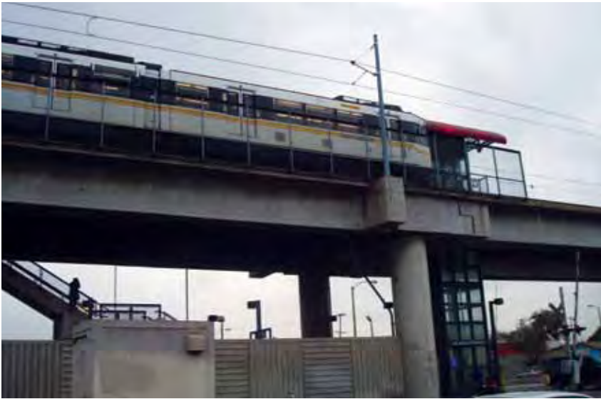
View along the east side of Slauson Station
