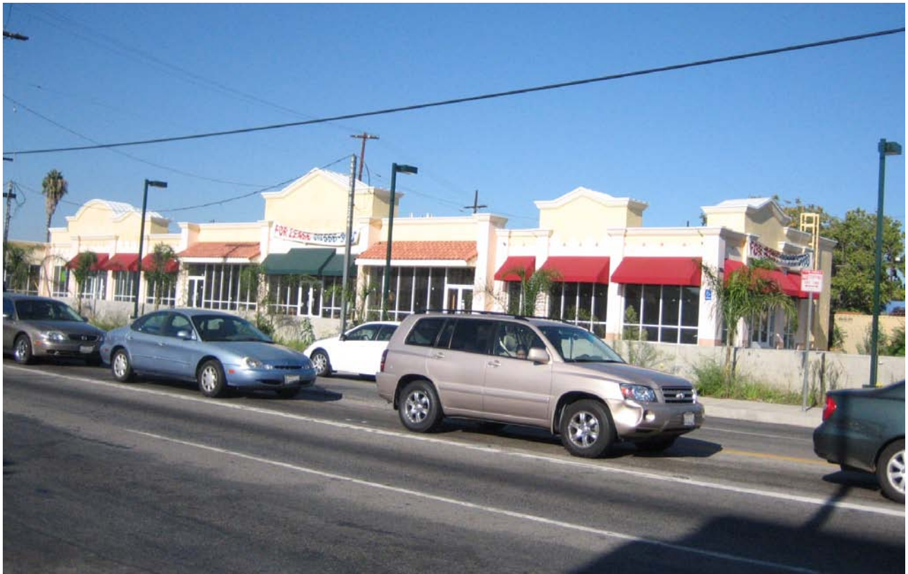
Potential location of the Northbound Station near Sherman Way for the Canoga On-Street Dedicated Bus Lanes Alternative
