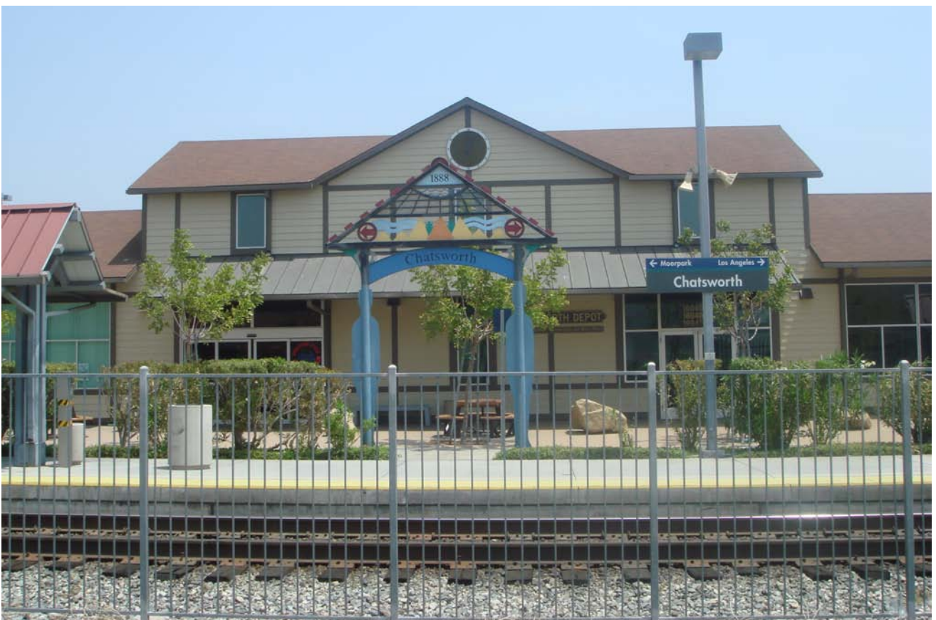
View of the Chatsworth Metrolink Station looking east of the railroad tracks
