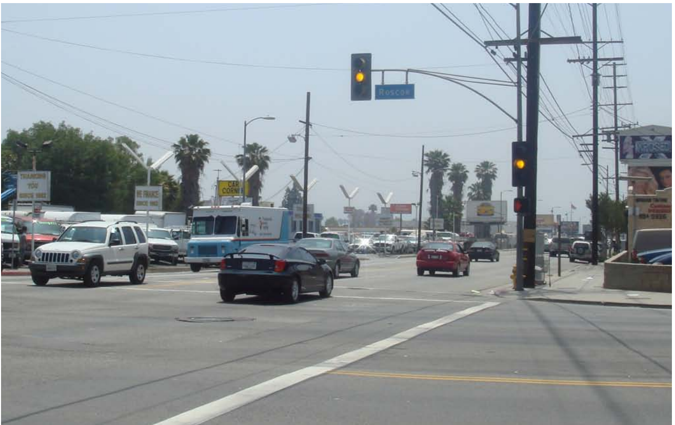
The maze of overhead wires on Canoga Avenue at the Roscoe Boulevard intersection
