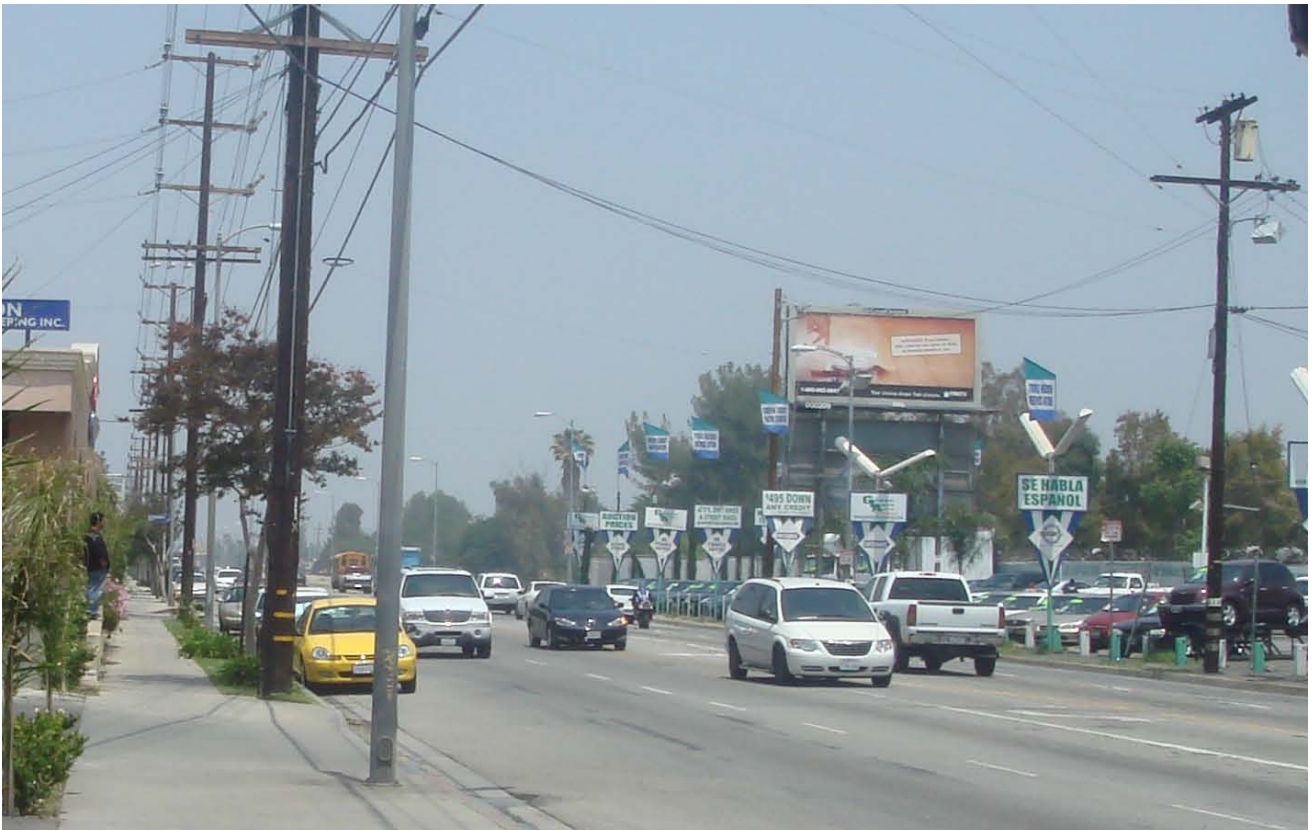
Potential site of the Northbound Station at Roscoe Boulevard for the Canoga On-Street Dedicated Bus Lanes Alternative
