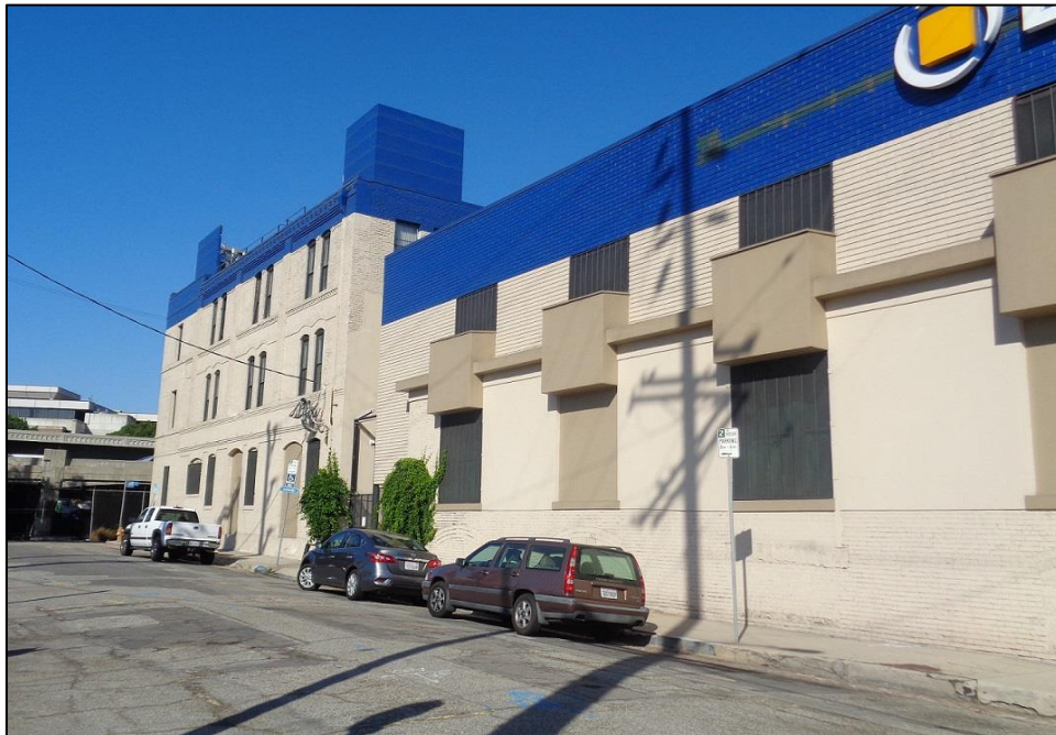
Photo: The northwest corner of the building is to the left of frame. ICF, September 2017.
