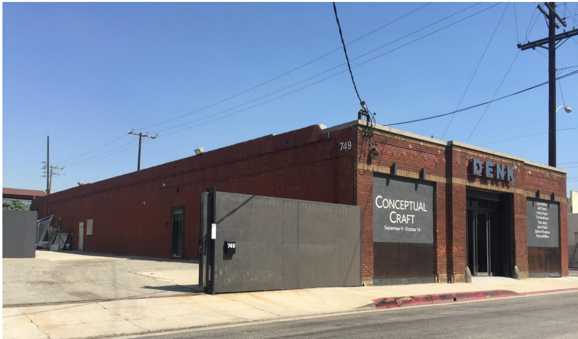
Overview of south-west corner. View to north-east. ICF, 2017.
