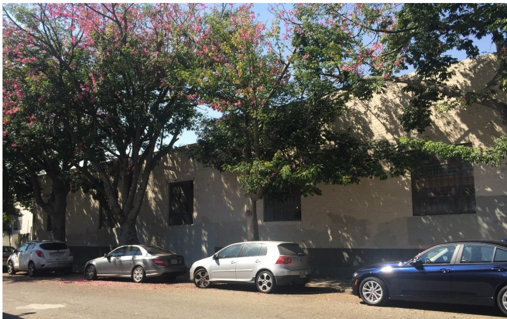
Overview of east elevation. View to west. ICF, 2017.
