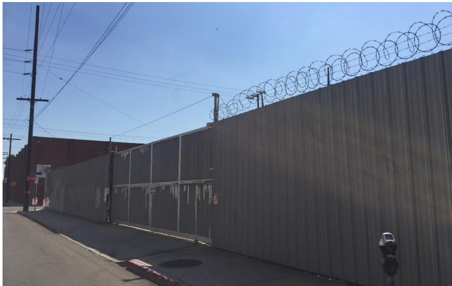
Overview of north elevation. View to south. ICF, 2017.
