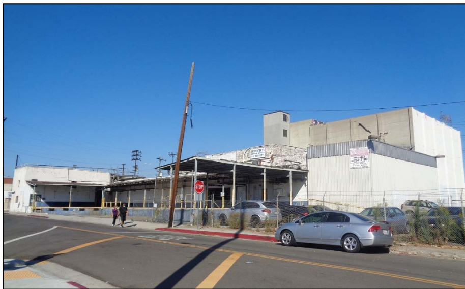
Figure 3.3.7 View of the National Ice and Cold Storage Facility from Center Street
