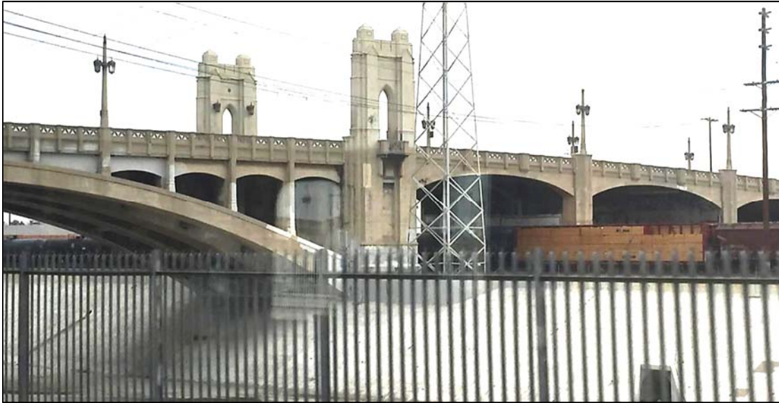
4 th Street Viaduct, camera facing northeast. ICF, August 11, 2016
