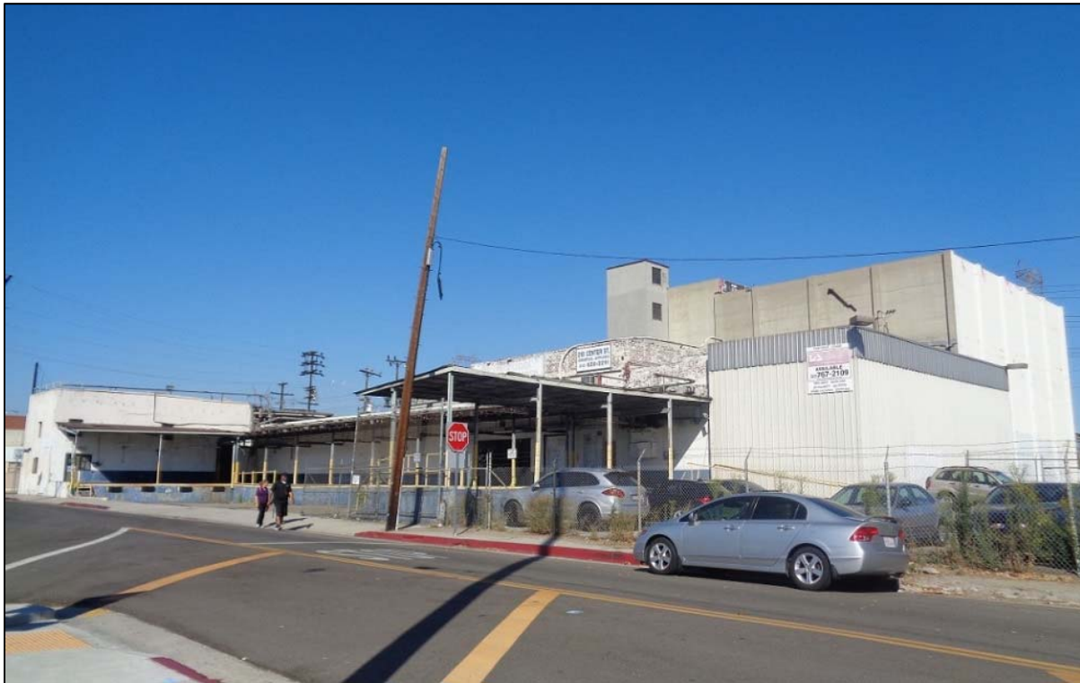
Figure 2: National Ice and Cold Storage Facility, primary elevation. View northeast. ICF, 2017.
