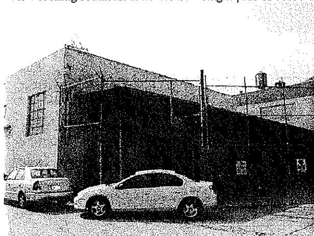
View looking southwest at c1940s ancillary building.
