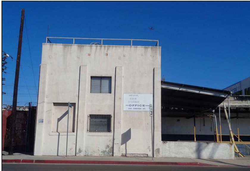
Figure 4: National Ice and Cold Storage Facility, primary elevation, detail of Engine Room. View east. ICF, 2017. Detail of the National Ice and Cold Storage facility buildings:
