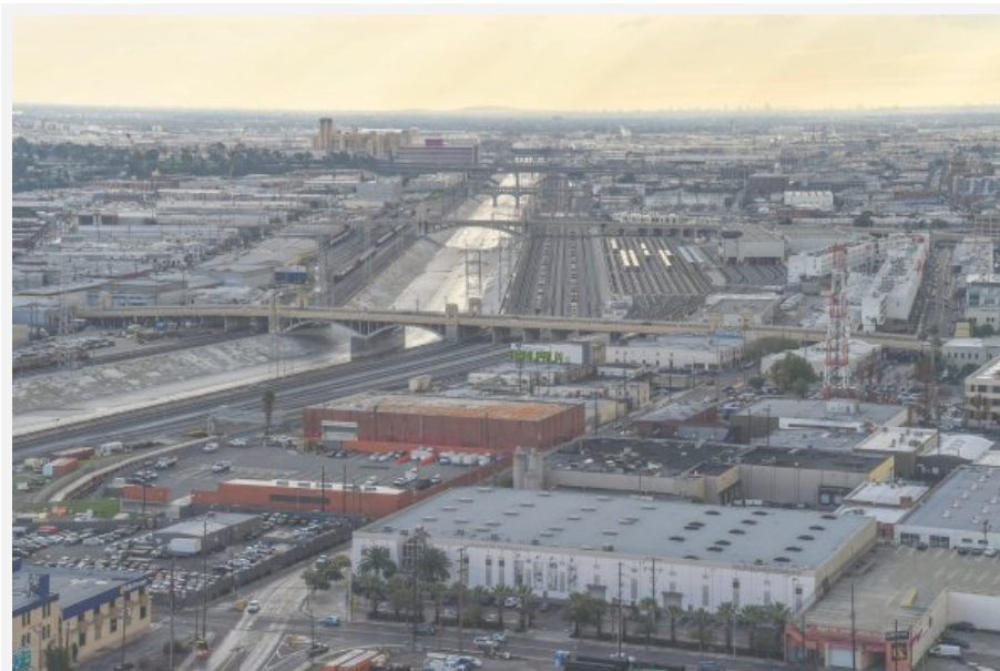
A view of the rail yards for the Red/Purple Line subway and the entrance to the tunnel at bottom left. Photo by Steve Hymon/Metro.
