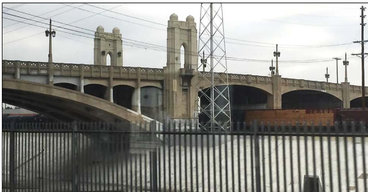
Figure 3.3.2 View of the 4 th Street Bridge from Mission Road
