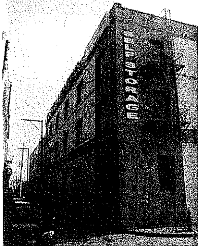
View looking southeast at northeast facing façade of c1899 building.
