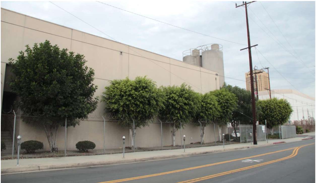
Figure 3.1.6 View Across Center Street from LAPD Viertel's Central Division Police Garage
