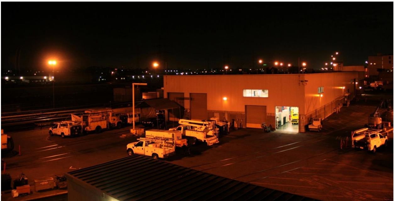
Figure 3.1.24 View of Existing Division 20 Rail Yard Night Lighting from the 1 st Street Bridge (Facing South)
