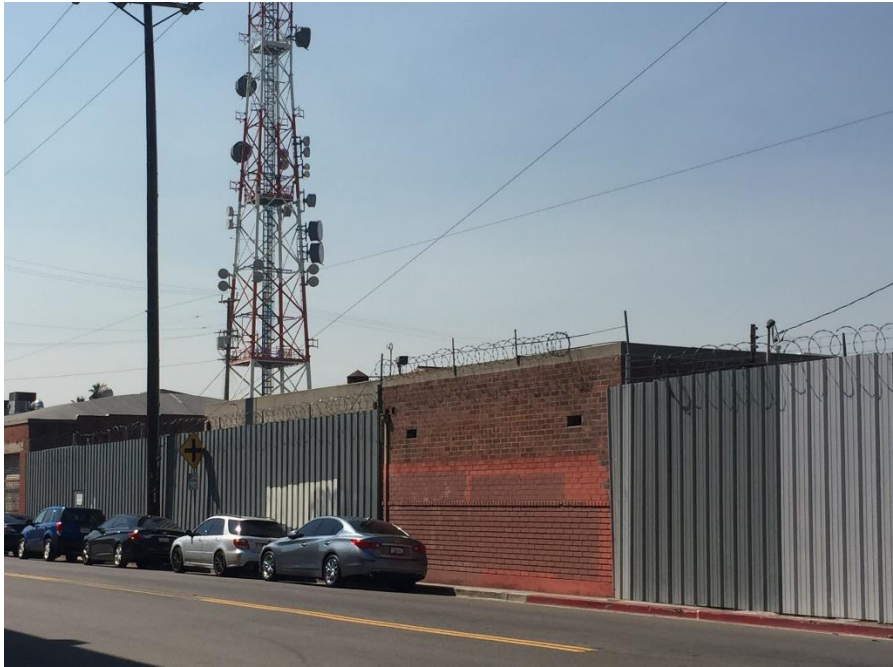
Overview of east elevation. Showing concrete-block and brick buildings. ICF, 2017.
