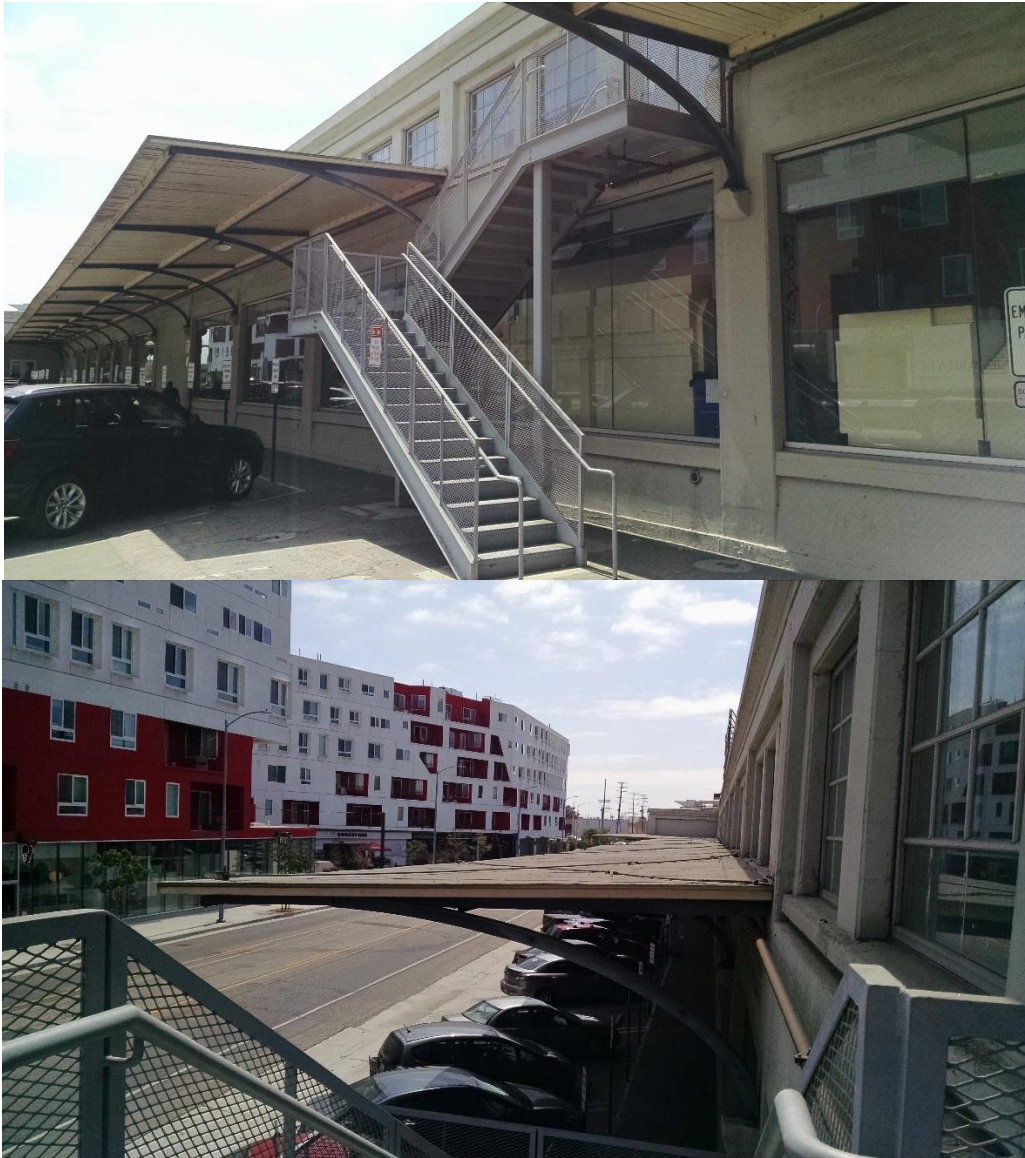
Figure B-1: Site ST-3, Sci-ARC, Top of Stairs Measurement Position
