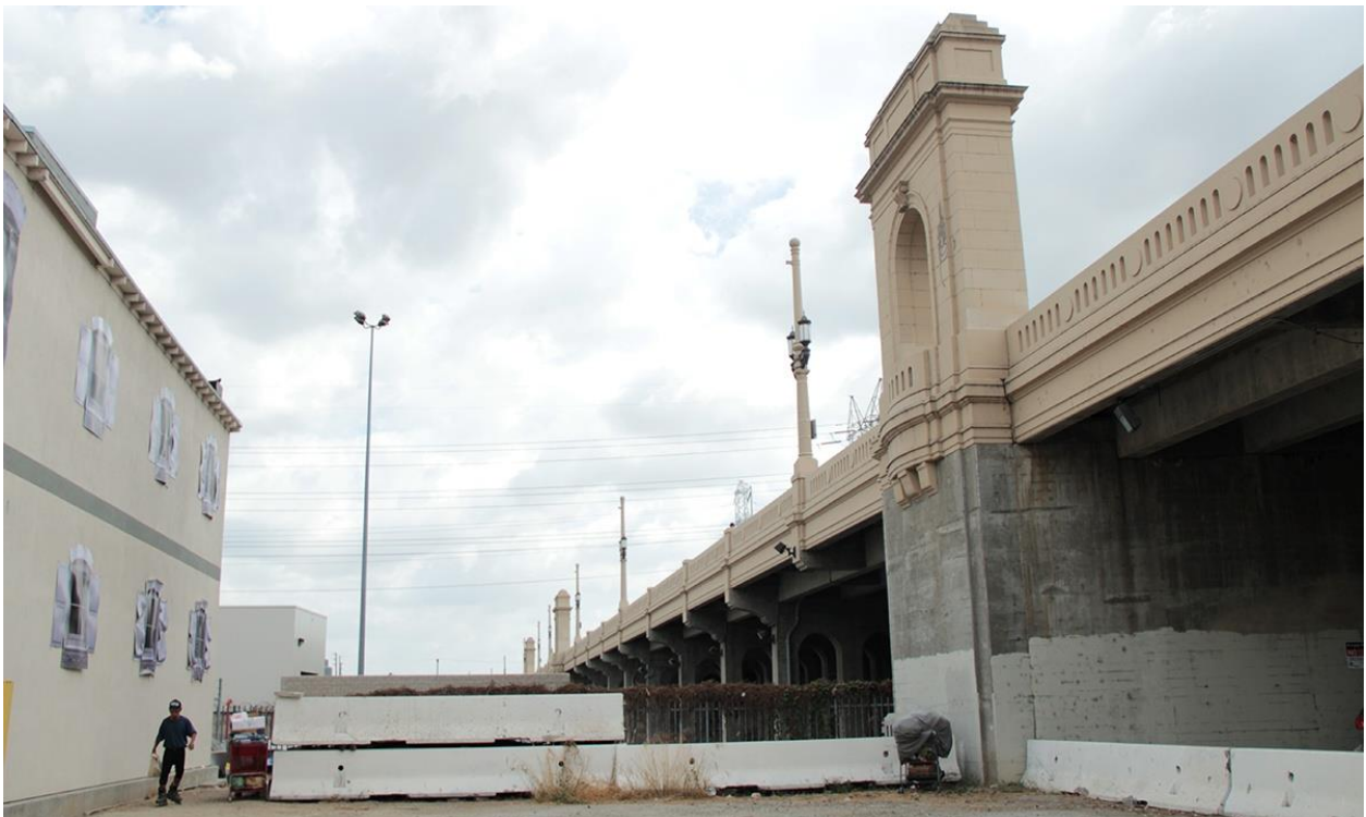
Figure 3.1.17 View of the 1 st Street Bridge from Center Street
