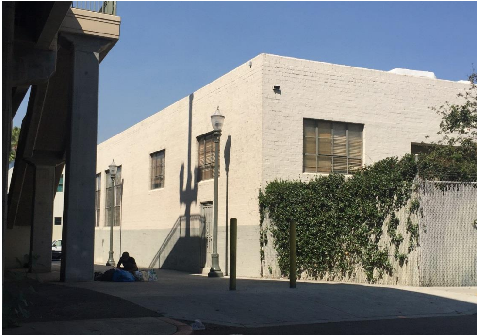
Overview of south-east elevation. View to north-west. ICF, 2017.
