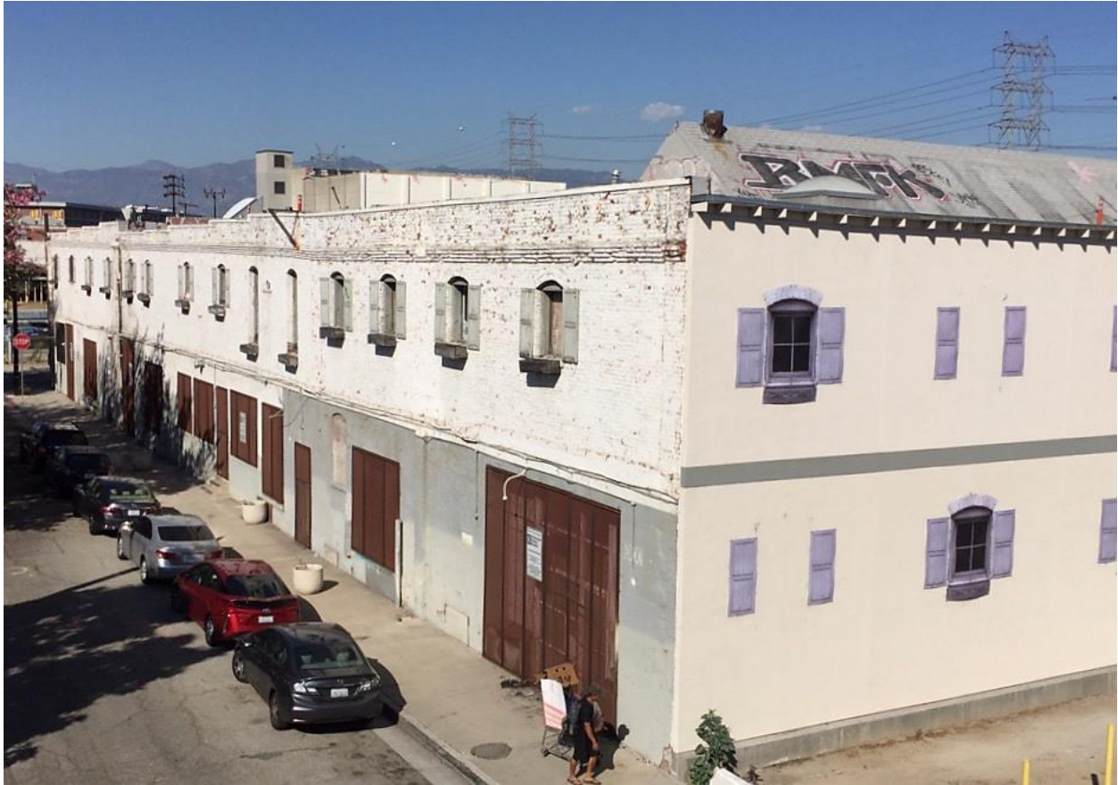
Lysle Storage Company/Citizens Warehouse, showing truncated south elevation to right of frame. View: NE. Photo: ICF. September, 2017.
