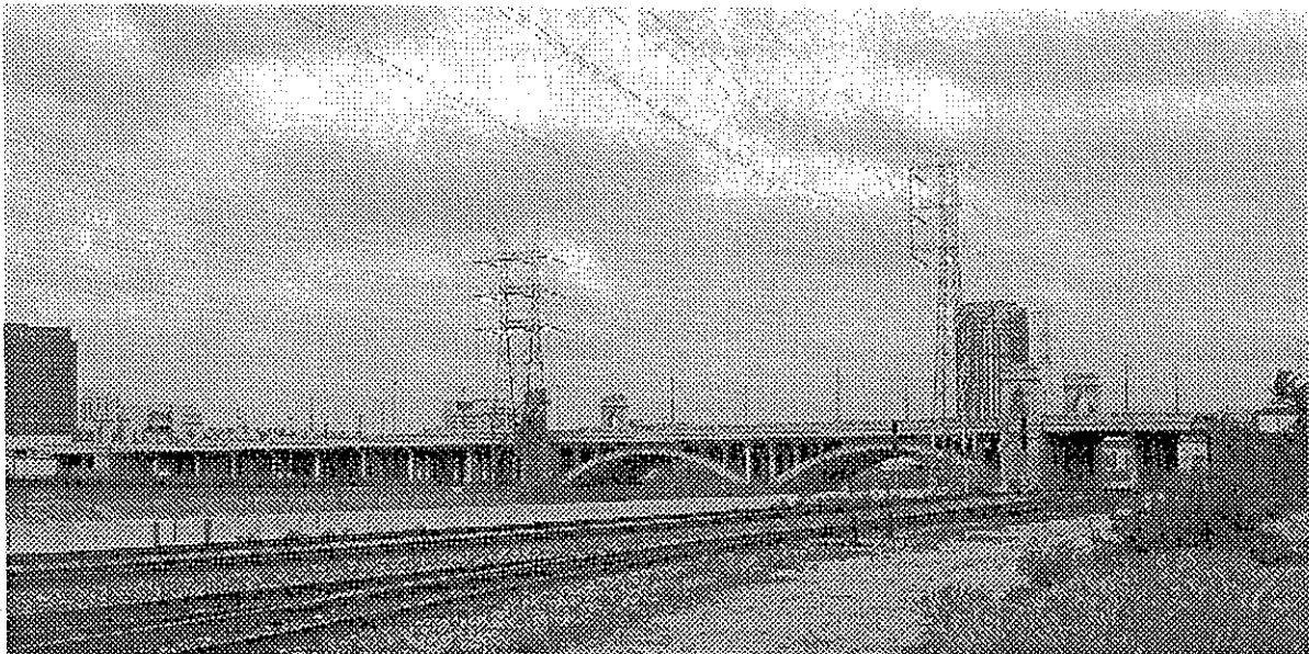
1st Street Viaduct, looking northwest.
