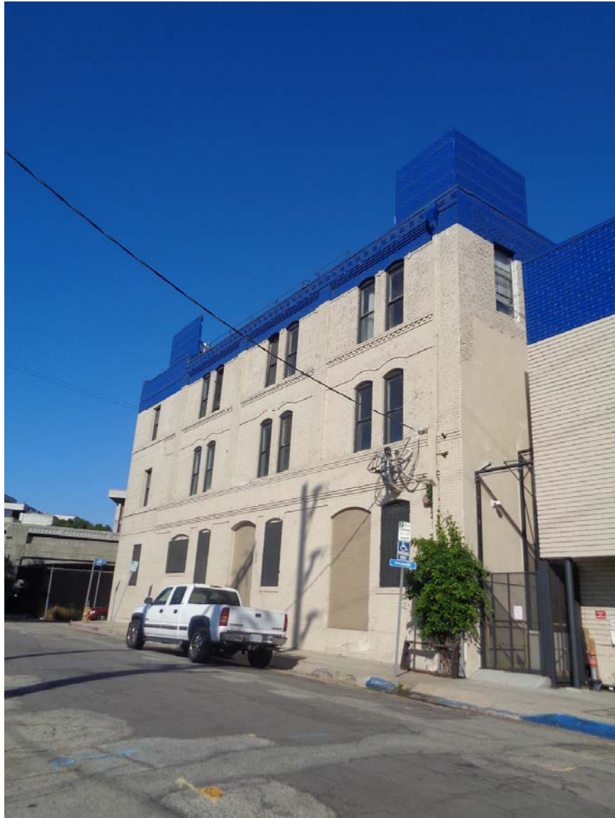
Khan-Beck Co./ Friedman Bag Company, detail of northwestern portion identified by SurveyLA in 2016, camera facing northeast. ICF, September 27, 2017.
