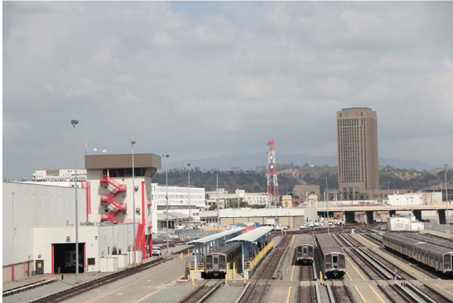
View of 1 st Street Bridge from 4 th Street Bridge
