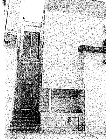
View looking southeast at 2-story corridor between c1899 and 1906 buildings.
