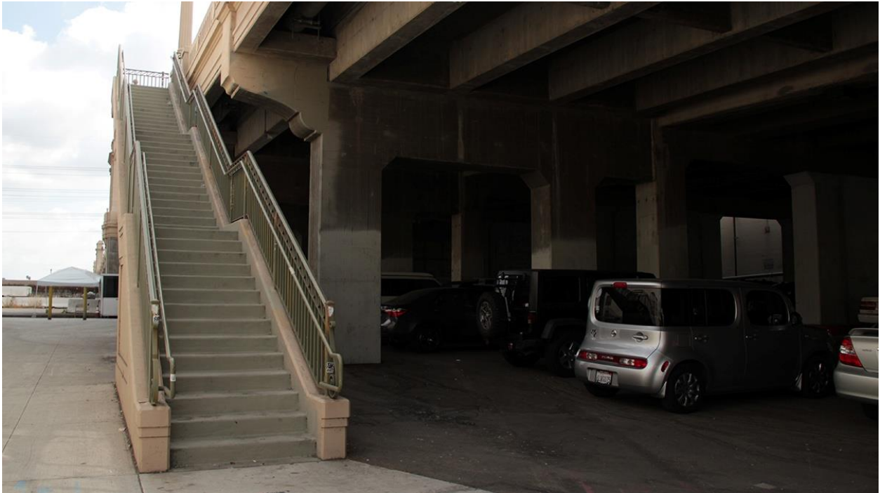
Figure 3.1.18 View of the 1 st Street Bridge Pedestrian Access from Center Street
