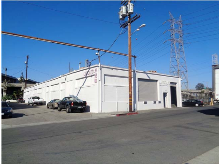
Primary and west elevation of Amay's Bakery and Noodle. View: NE. Photo: ICF, September 27, 2017.
