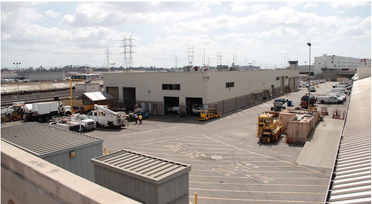
Figure 3.1.21 View of the Future Storage Tracks (Southern) from the 1 st Street Bridge
