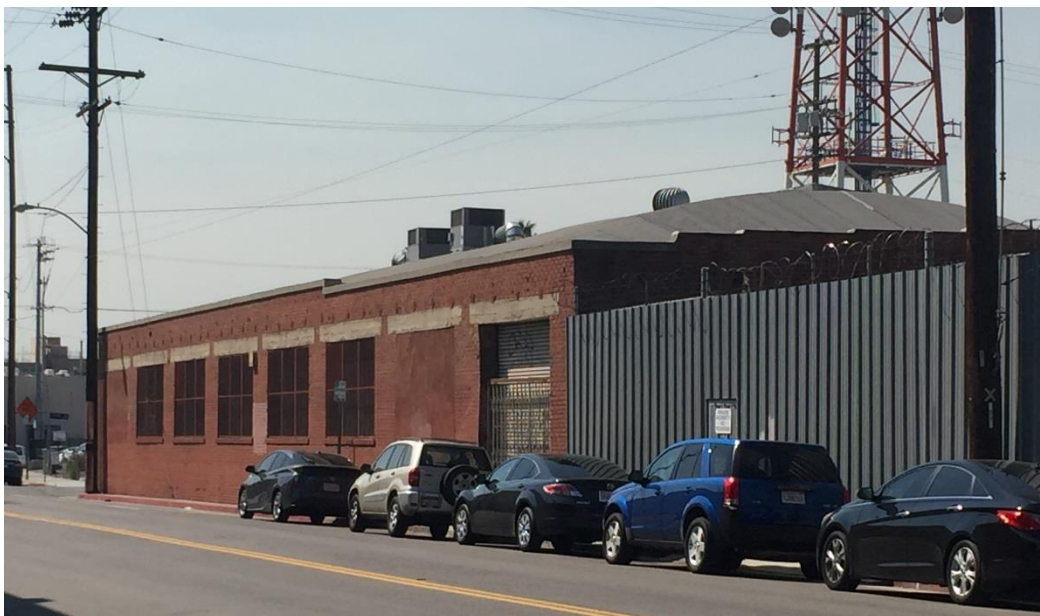
Overview of east elevation. View to south-west. ICF, 2017.
