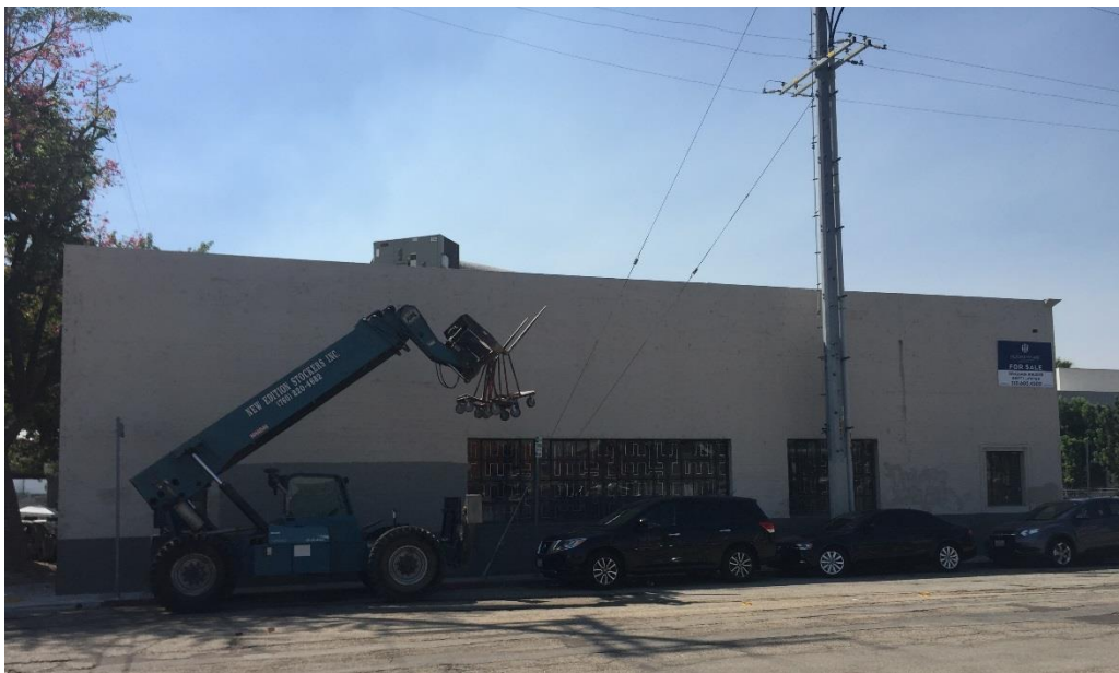
Overview of north elevation. View to south. ICF, 2017.
