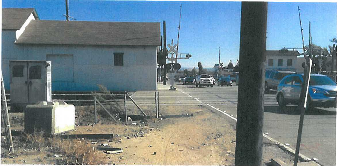
Pedestrian travel crosses the tracks directly, and uses a dirt path adjacent to Garey Avenue, north of the crossing.
