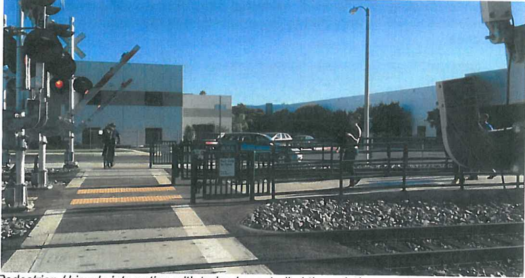
Pedestrian / bicycle interaction with trains is controlled through the use of gates.
