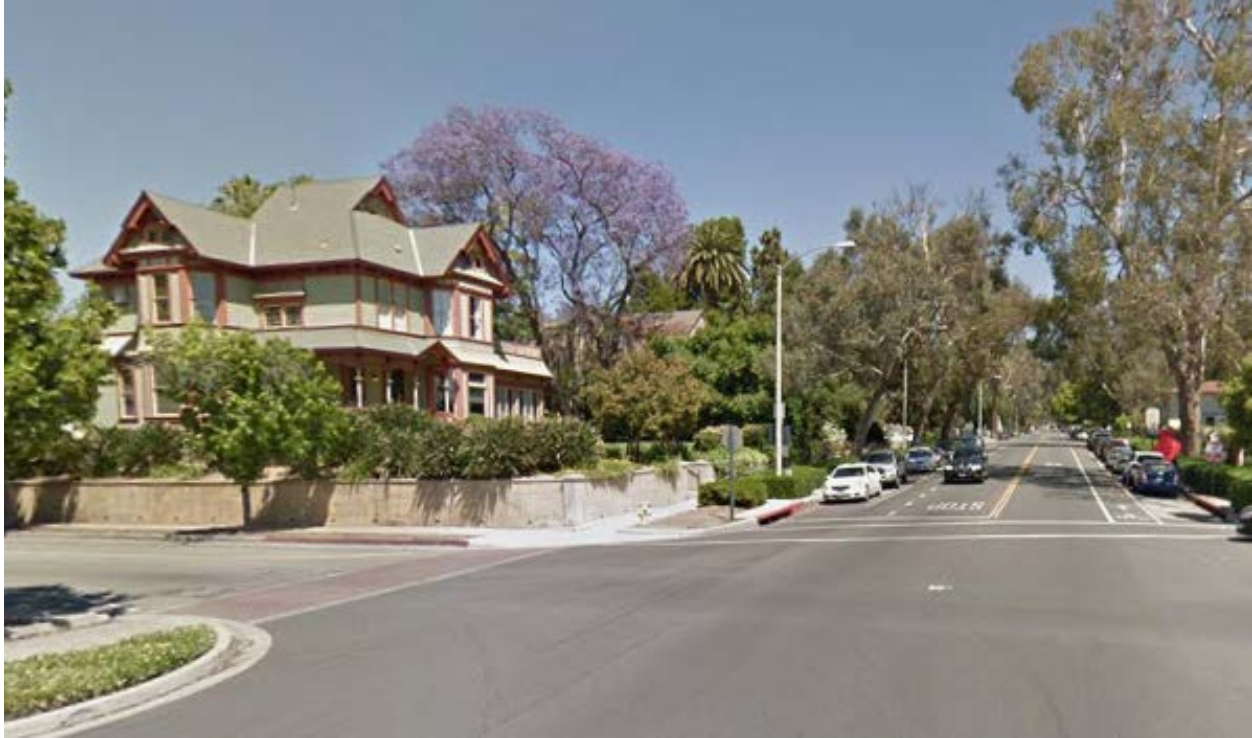
Figure 4.6-11. 105 N. College Avenue (south and east elevations facing the reconfigured parking facility)
