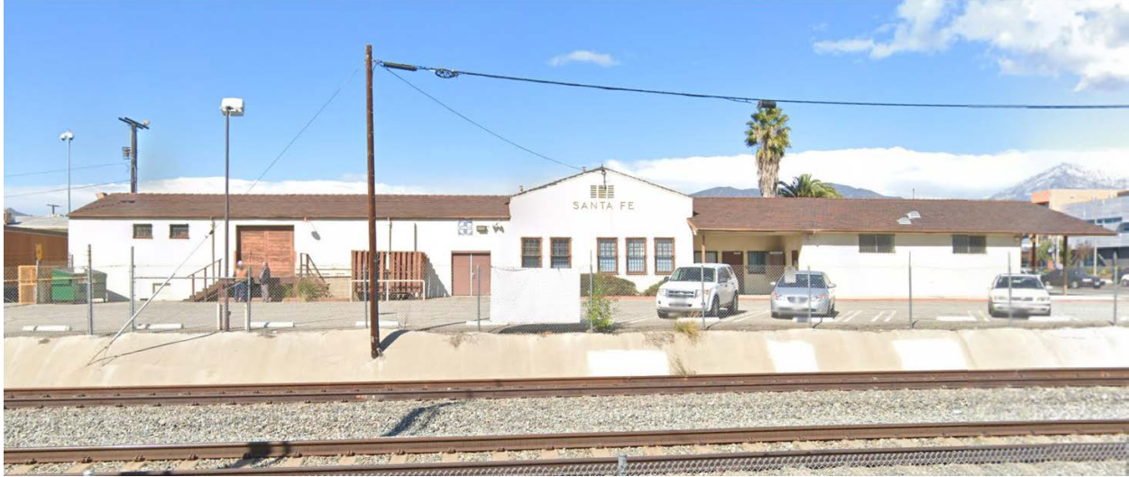
Figure 4.6-10. Santa Fe North Pomona Station (south elevation facing the reconfigured parking facility), 2701 N. Garey Avenue, Pomona
