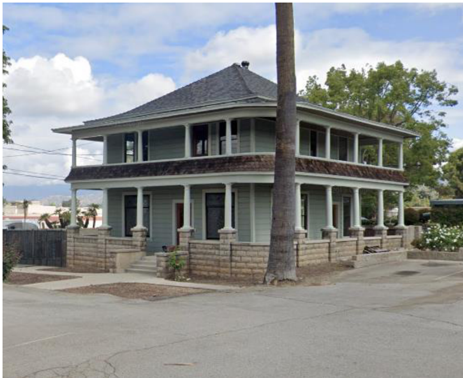
Figure 4.6-6. William T. Michael Residence, 219 E. Arrow Highway, San Dimas
