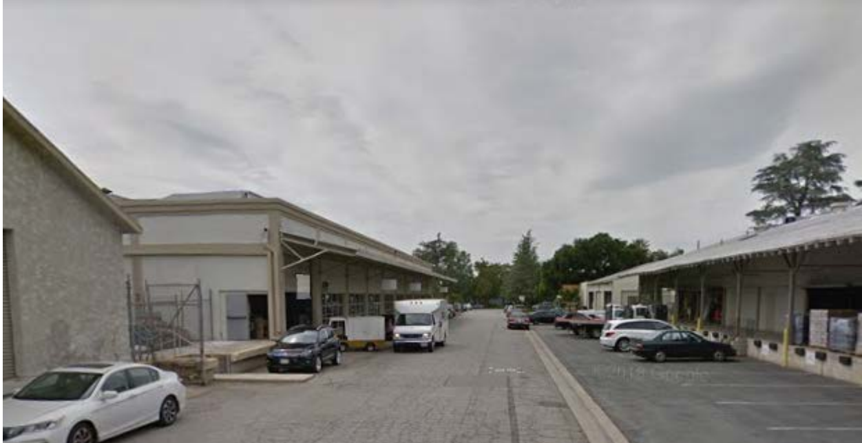
Figure 4.6-9. La Verne Citrus Packing District, view west from the F Street and 1st Street intersection, view toward 2247-2275 1st Street (right) and 2230 1stStreet (right), La Verne
