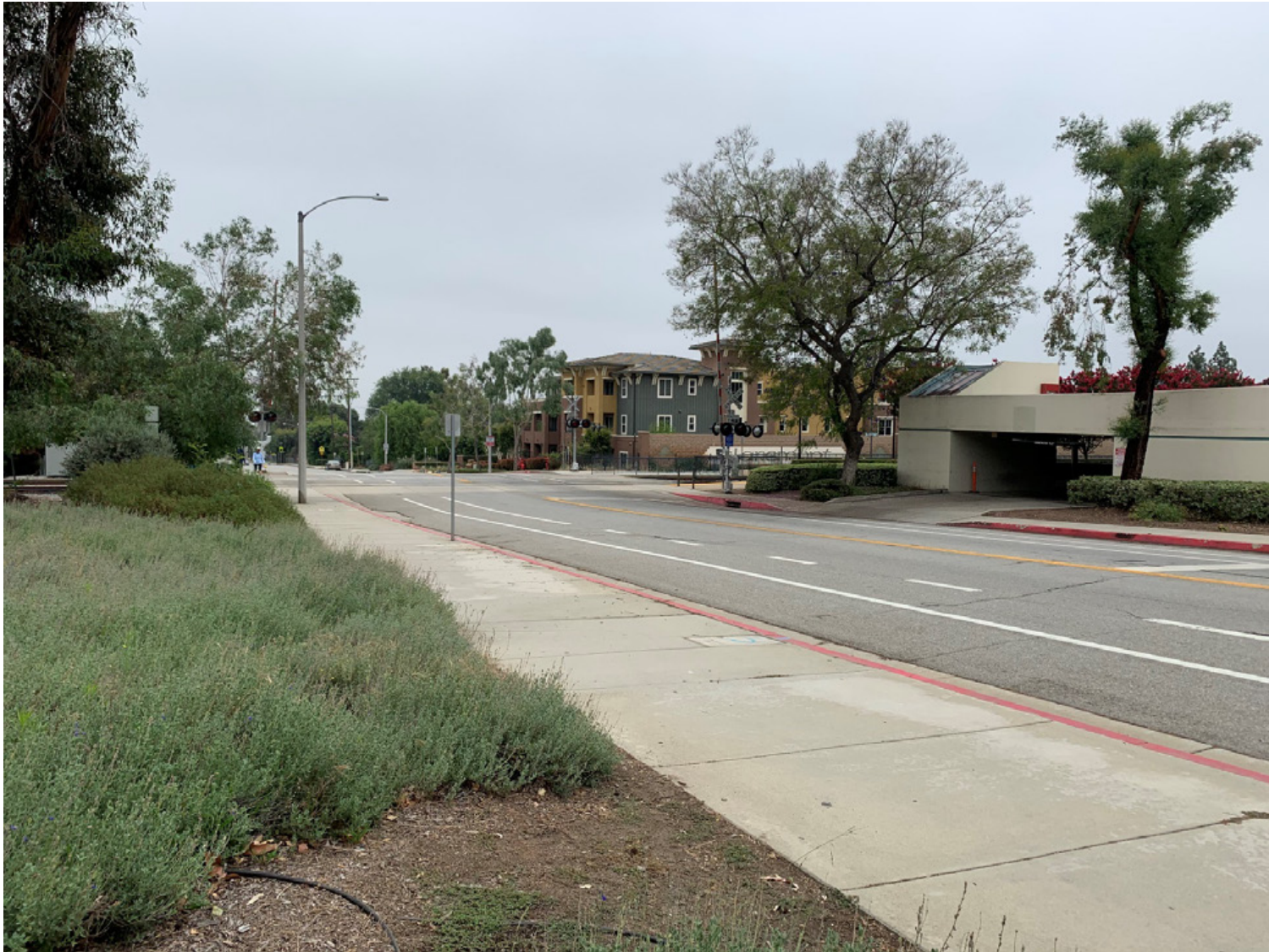
Figure 4.13-10. View looking southwest from the intersection of North College Avenue and East First Street toward the location of the new pedestrian crosswalk near the reconfigured Claremont Station parking facility.
