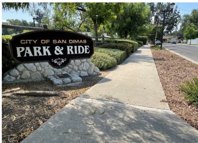
Sidewalks along the border of the Subject Property demonstrate negligible cracking.
