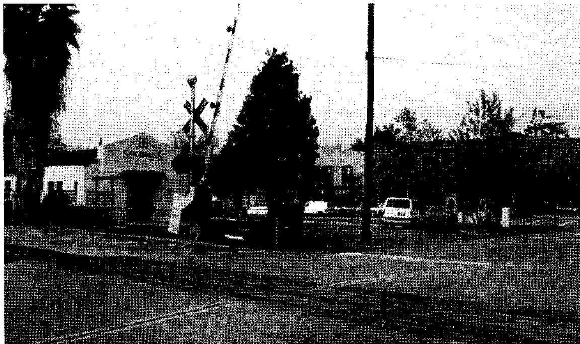
FIGURE 3-17.13: SAN DIMAS, ATSF DEPOT AND OLD BUSINESS DISTRICT, VIEW SW
