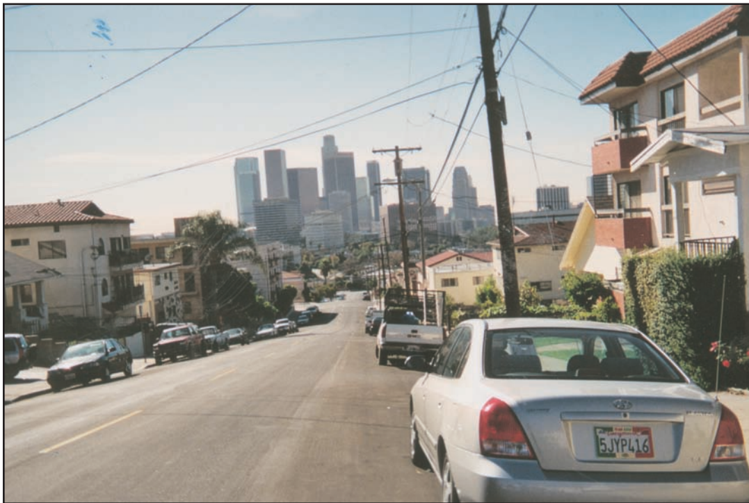
Photograph 11: Southerly view of the downtown skyline from Figueroa Terrace north of the Pasadena Freeway. The Project site is located to the left of the existing high-rise cluster in the background of the photograph. The Project's future towers would be visible from this perspective.
