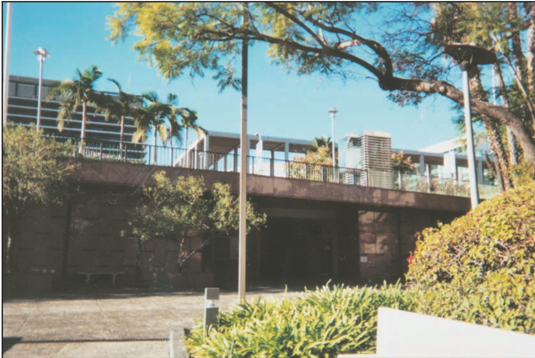
Photograph 6: The east portal of the pedestrian tunnel leading under Grand Avenue to the Los Angeles Music Center is visible on the right of the photograph. The grade difference between the westerly Civic Mall and the Music Center is evident in the height of the wall in the center of the photograph. Landscaping in the foreground is typical of the west segment of Civic Mall.
