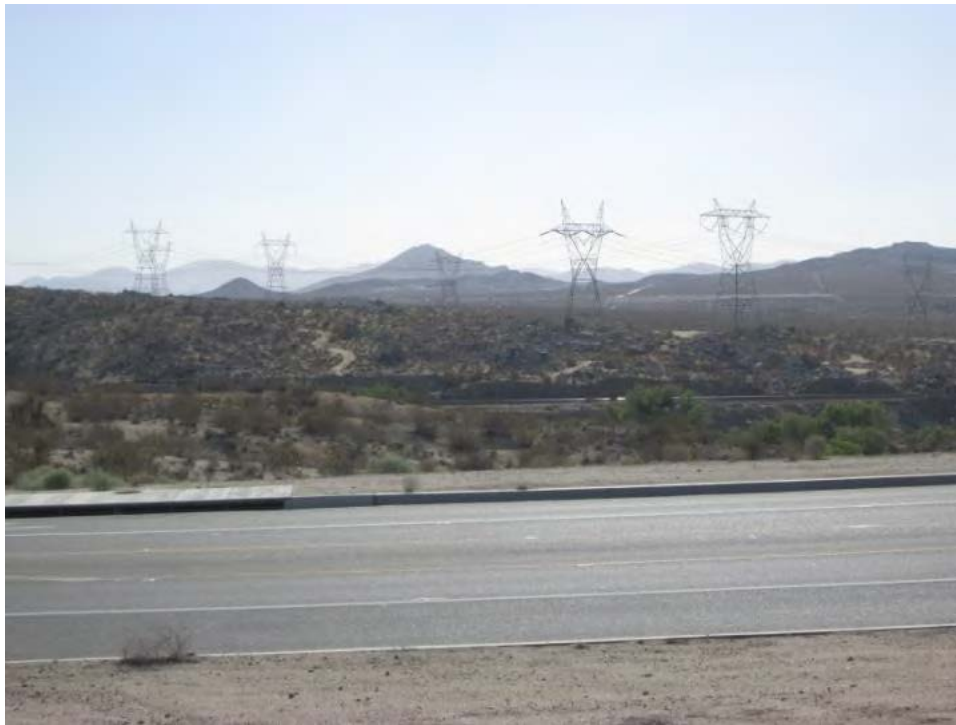
The two sets of ATSF/BNSF tracks are situated along the east bank of the Mojave River. View looking east from National Old Trails Highway/Route 66.
