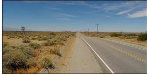
Source: Parsons, 2013 (Existing roadway in project area). The HDC would improve east-west mobility through the High Desert region of southern California.
