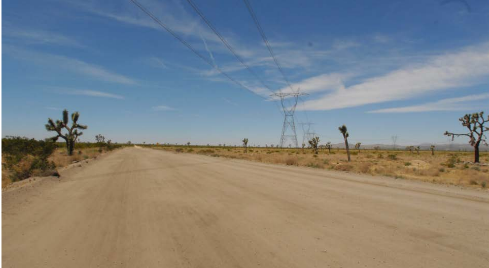
Figure 3.1.7-30 KV #14 Existing View
