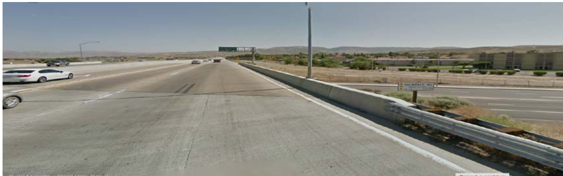
Figure 3.1.7-5 KV #2 Existing View
