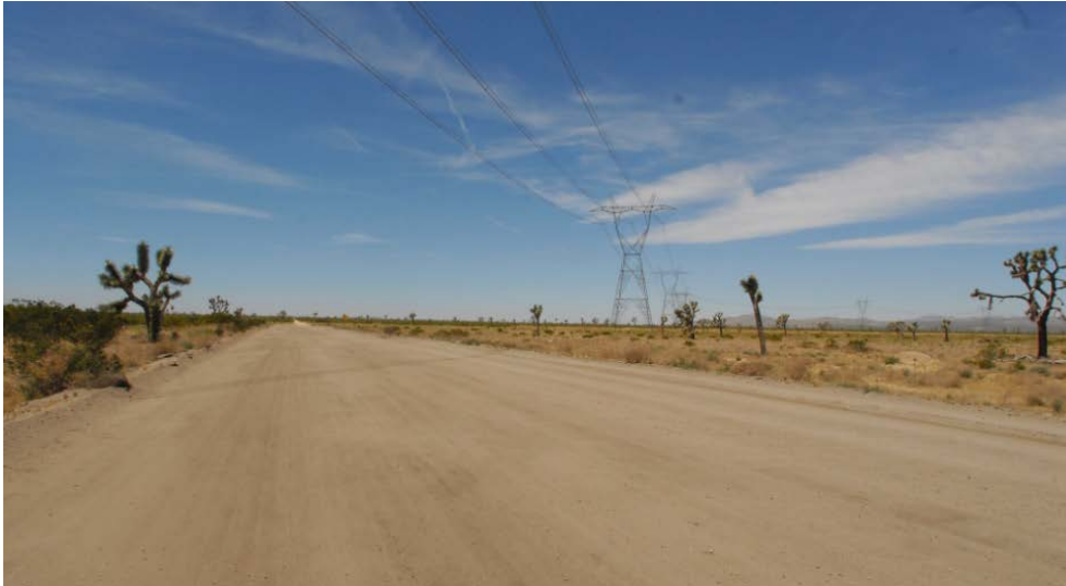
Figure 3.1.7-30 KV #14 Existing View
