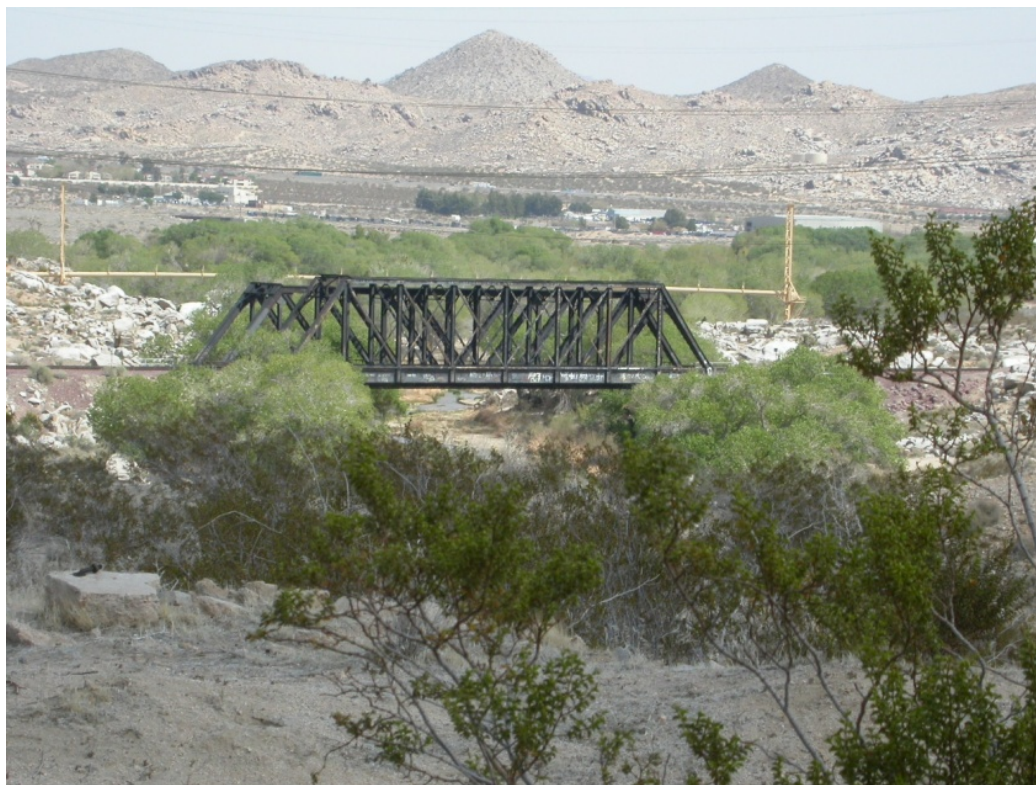
Figure 3.6-2 Mojave River Crossing
