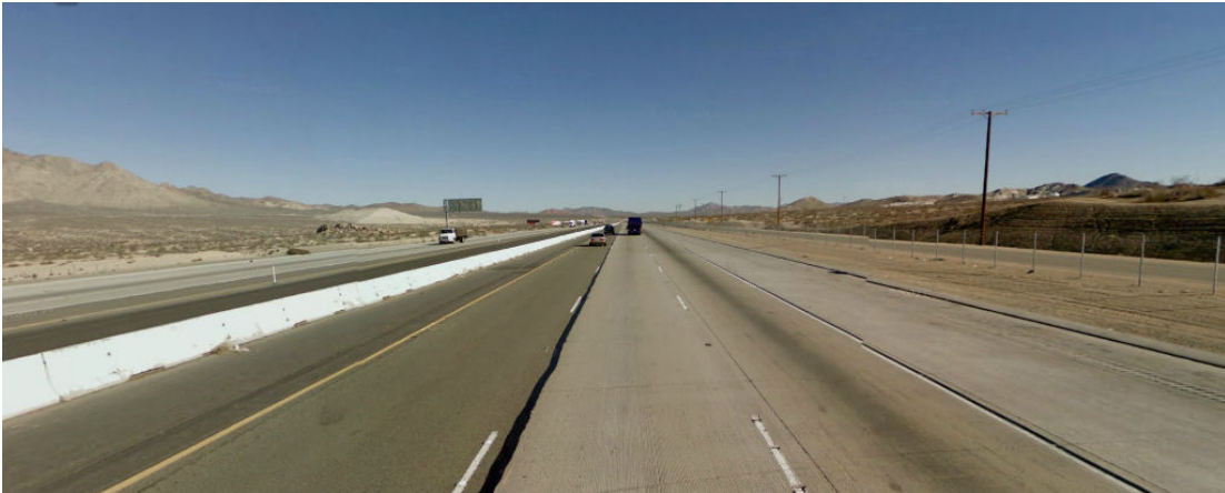
Figure 3.1.7-44 KV #21 Existing View
