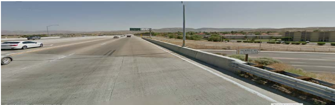
Figure 3.1.7-5 KV #2 Existing View
