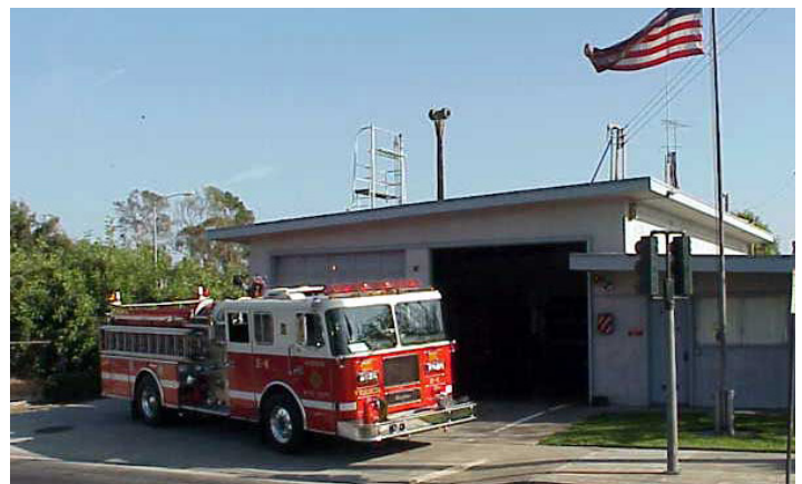
Fire Station No. 4 in the City of Vernon would require relocation under all I-710 build alternatives.
