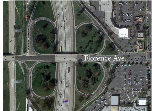
The "cloverleaf" interchanges built in the 1950s are not able to handle today's volume of traffic.
