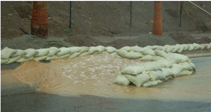
Controlling stormwater runoff during construction is critical to maintaining water quality in the Study Area.
