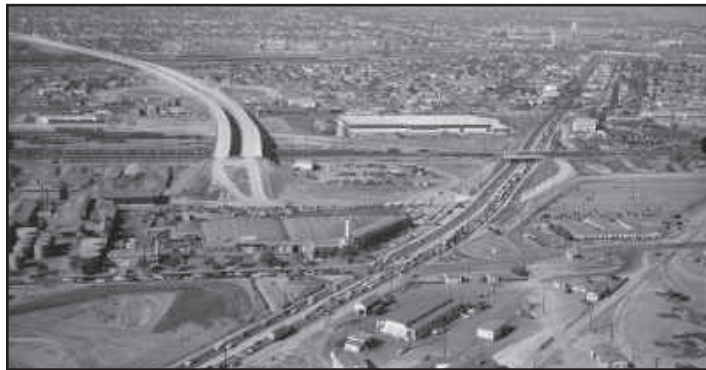
When State Route 7 (I-710) was built in the 1950's, there was still a great deal of agriculture and open space in the surrounding area.
