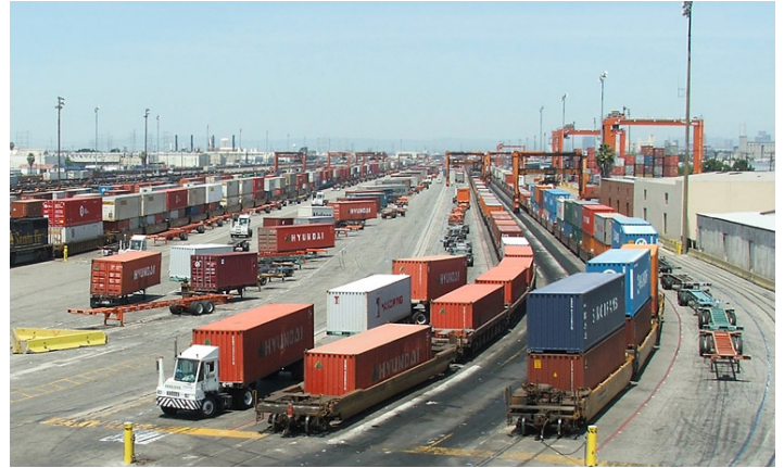
I-710 provides a critical linkage for interstate commerce between the San Pedro Bay ports, the BNSF and UP rail yards, and the rest of the nation.
