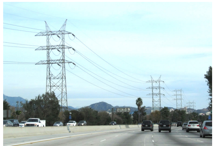
Under Alternatives 6A, 6B, and 6C, electrical transmission lines will be relocated to provide room for expanding I-710 to help reduce the amount of property that would otherwise need to be acquired.
