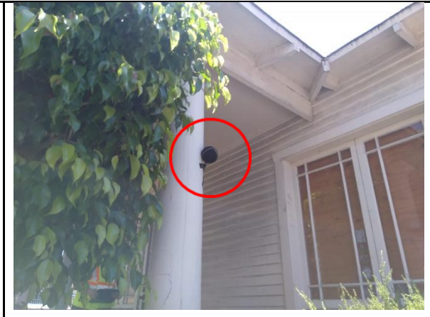
ML-20, facing house (looking SE)
